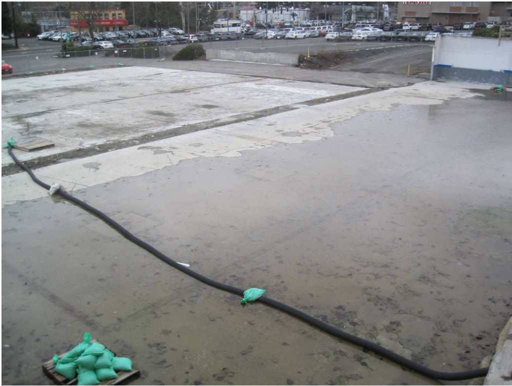
Photo 1. View looking northwest from above the southeast corner of the former dealership in February 2018.
