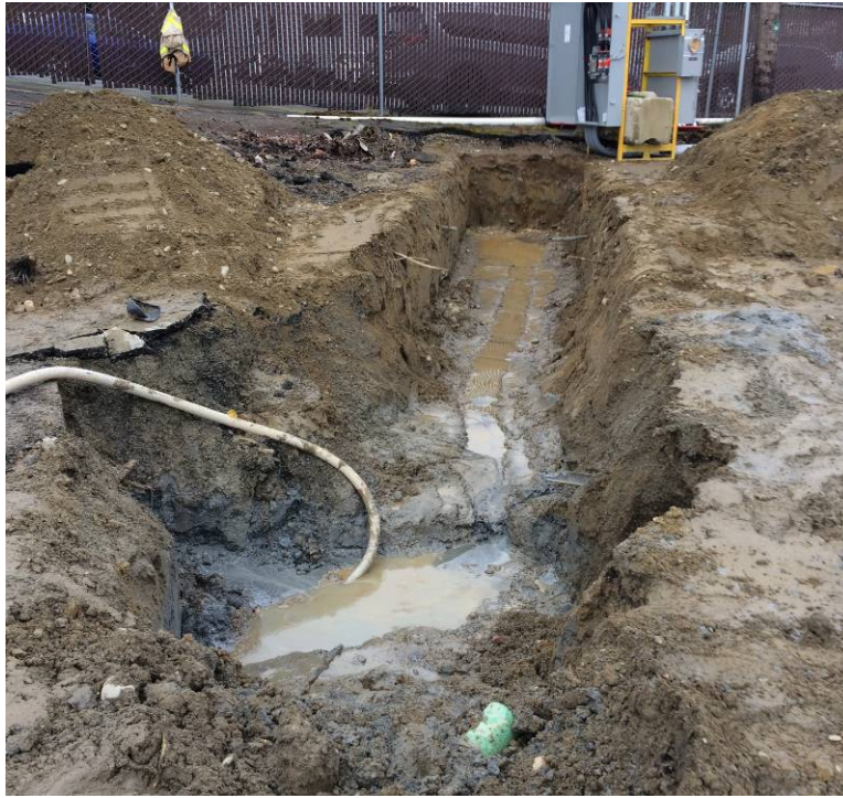
Photo 3. Electrical trench excavation, April 2018.
