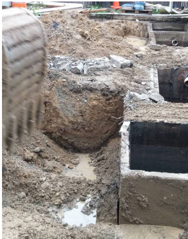
Photo 12. View of the oil/water separators being removed. October 2018.
