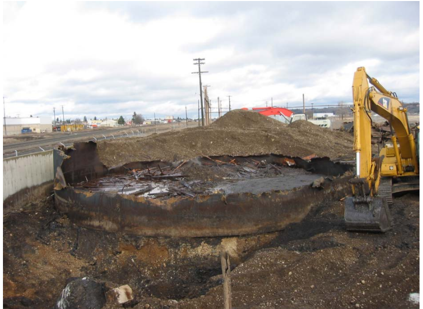
Black tank demolition, 2006.
