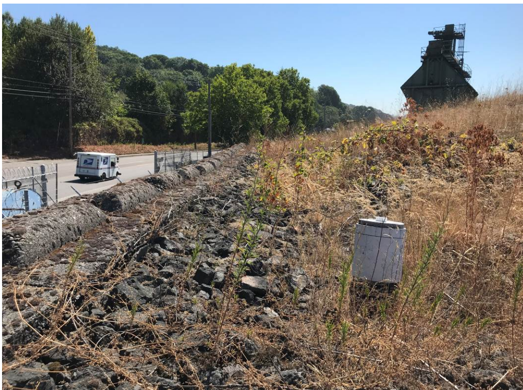
Photo 1: Top of containment cell looking east from northwest corner, northwest cleanout boot is visible in the foreground.
