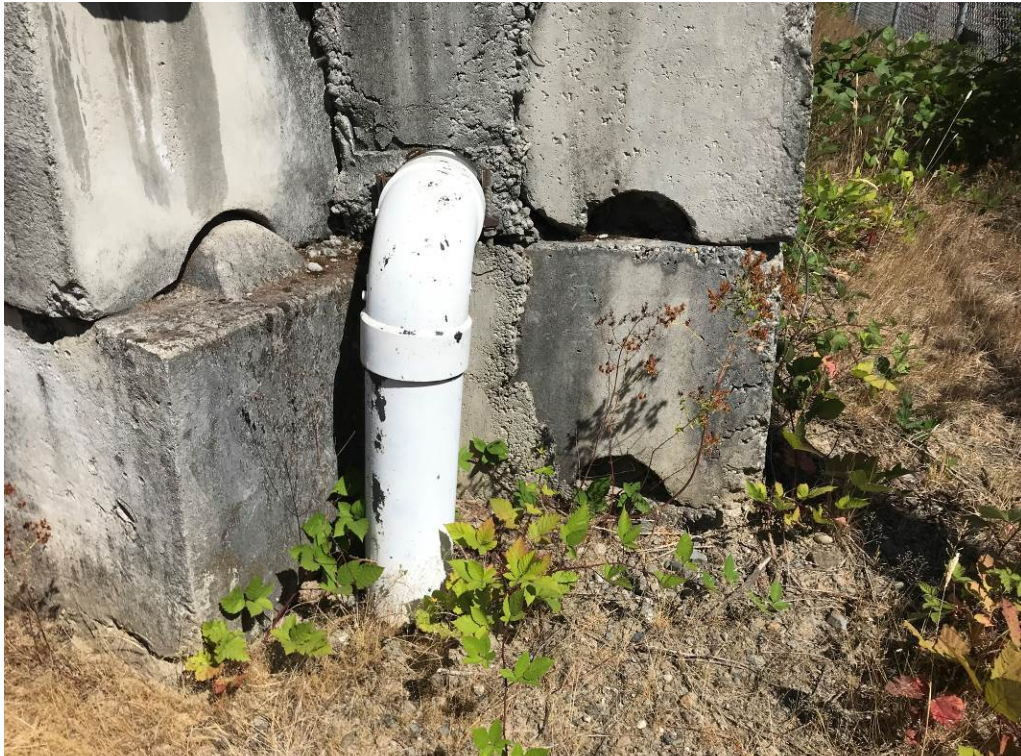
Photo 7: View to the north of the cell drain boot showing some aging on the paint coating.
