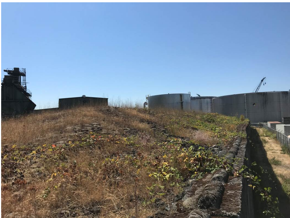
Photo 2: Top of containment cell looking south from the northwest corner, northern gas boot is visible.
