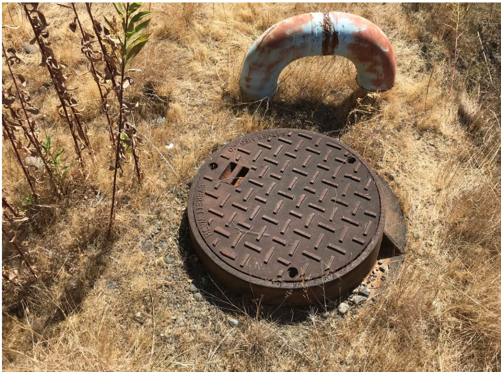
Photo 6: Leachate collection sump (manhole).
