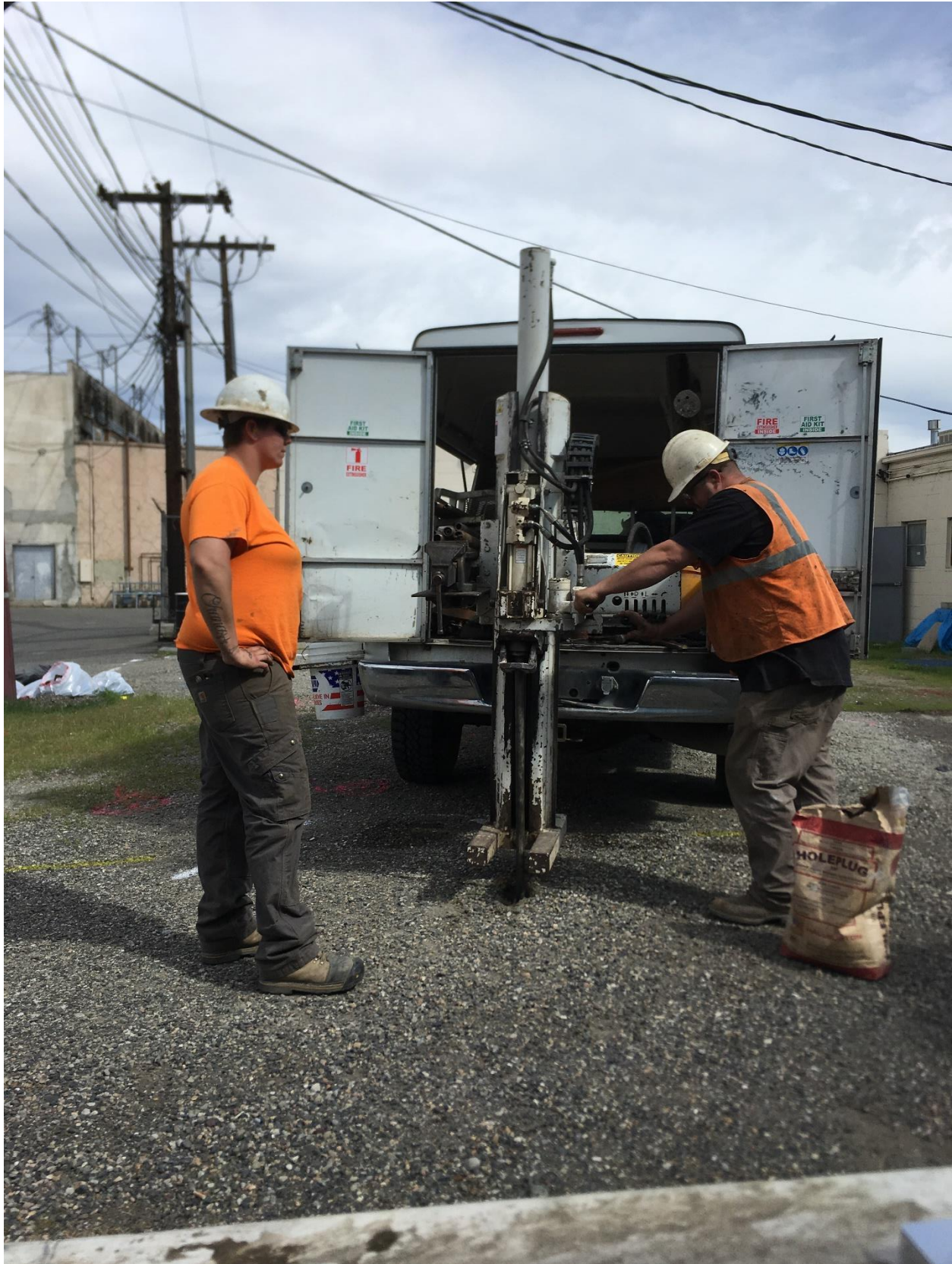
Photograph 4 – Drillers setting up to drill at boring SB-3 (facing north).
