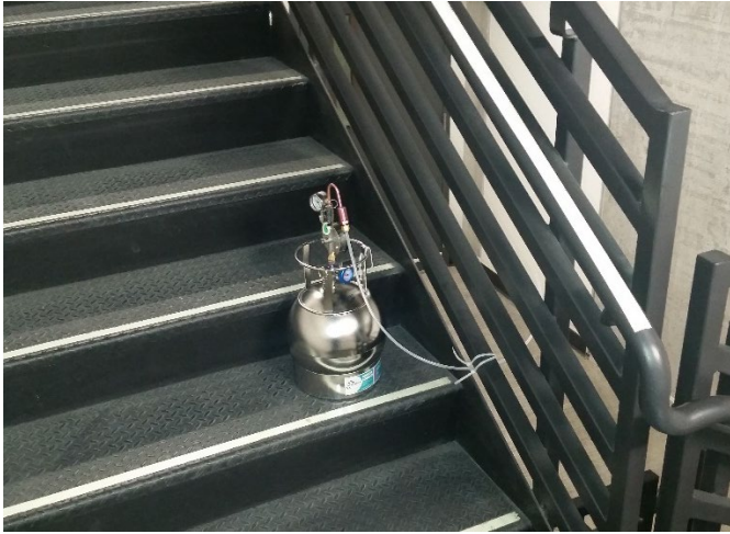
Photograph 1. Indoor air sample IA21, installed in Stairway 4 on Parking Level P5.
