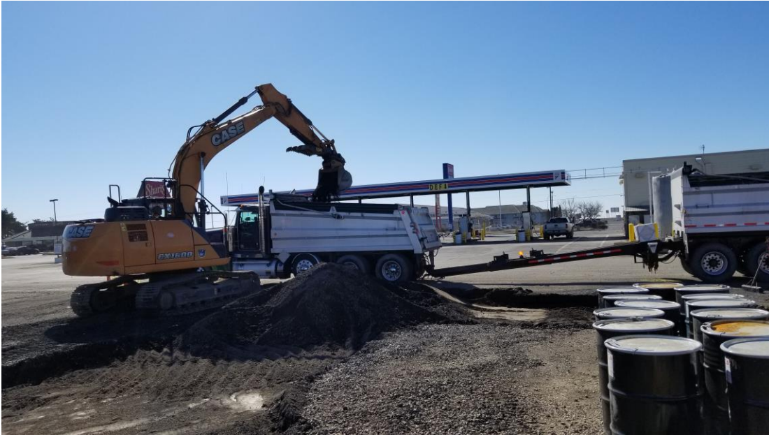
Photograph 3. Excavator direct-loading impacted soil into truck-and-trailer for off-site disposal.
