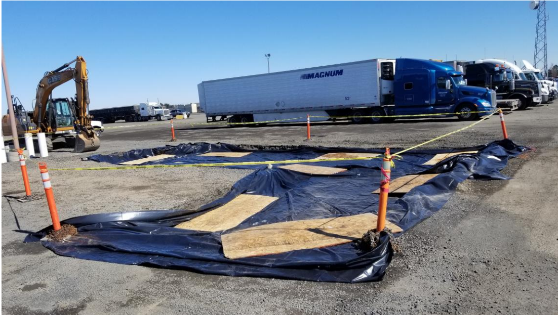
Photograph 5. Excavated area covered and coned off after excavation pending analytical results.
