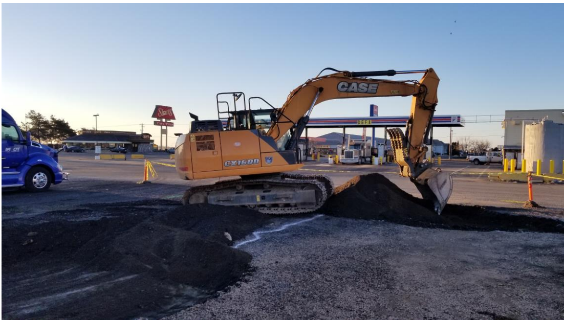
Photograph 2. Excavator beginning excavation.
