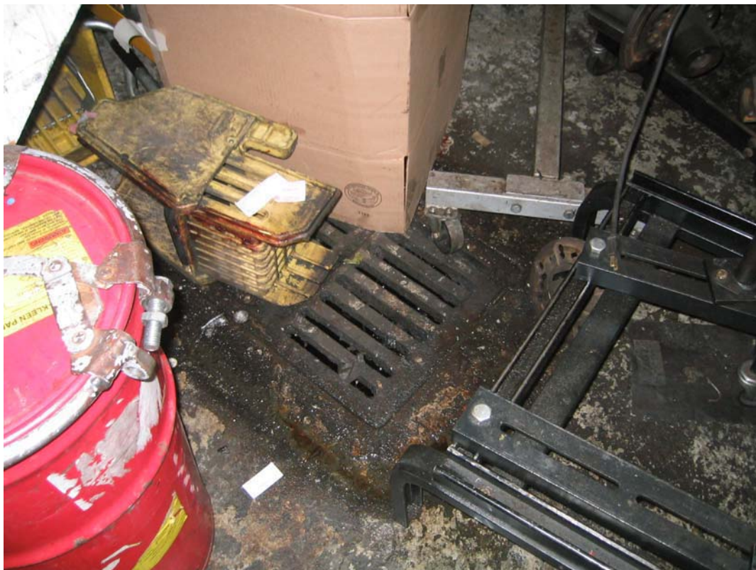
Photo 12. View of an interior floor drain in the service area at Dodge of Bellevue. Most floor drains in the service area showed evidence of oil staining but were cleaner than this one.
