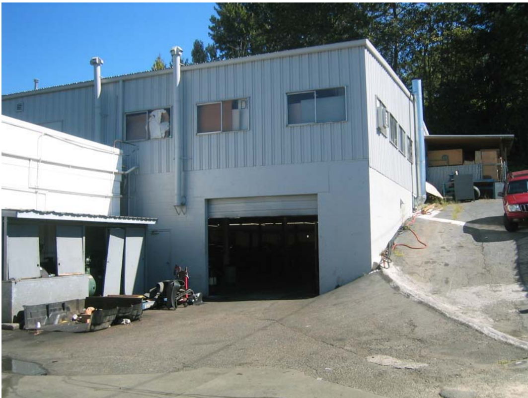
Photo 2. View looking east-northeast at the rear portion of the Eastside Chrysler-Jeep dealership. The top floor is occupied by offices and the parts department. The lower floor includes 19 service bays. An additional nine service bays are present in the building visible to the left.
