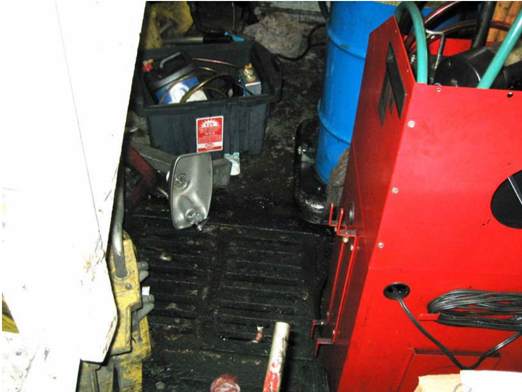
Photo 3. View of a floor drain at Dodge of Bellevue. The floor drain was surrounded by containers of new and used petroleum products. The drain was oil stained. All floor drains reportedly lead to an oil/water separator that is pumped out annually.
