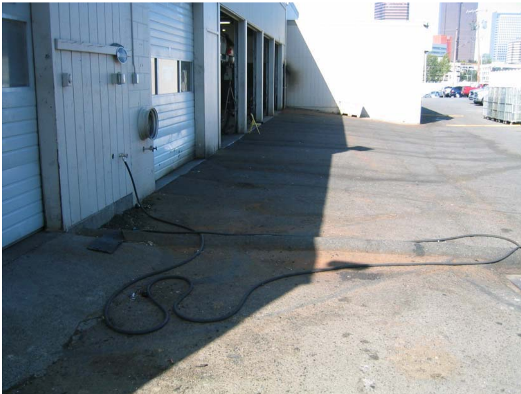
Photo 1. View looking west along the north side of a portion of the service bays at Dodge of Bellevue. Oil stains are visible across the asphalt leading to storm drains.
