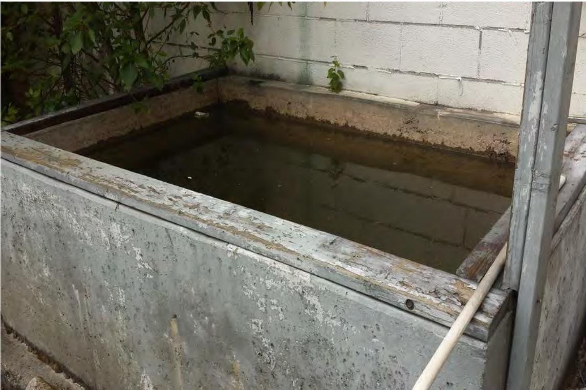
**Photo 10.** Containment vault on the south end of the Eastside Chrysler Jeep building that formerly held an aboveground oil storage tank (AST). The accumulated water was rusty and showed a slight sheen, and should be pumped out for proper offsite (non-stormwater) disposal.
