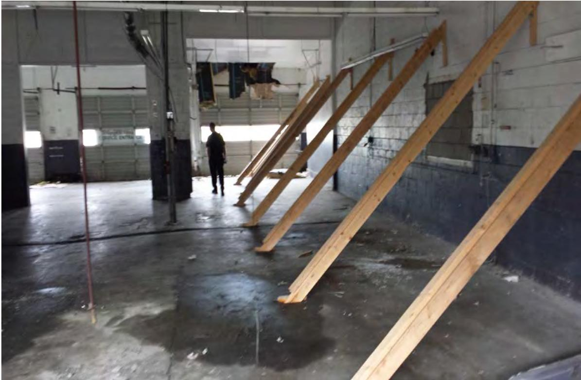
**Photo 5.** Interior view of the rear (easternmost) Dodge of Bellevue service bays. The timbered shoring was installed to support the back wall of the building after the easternmost section was demolished to make room for the 4<sup>th</sup> Street NE extension. Floor drains were observed along the foot of many of the garage doors.
