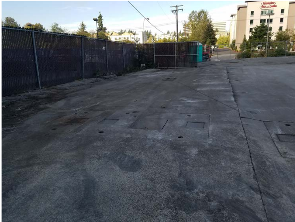
Photograph 5: Oil-water separator and drains on southern portion of Site.
