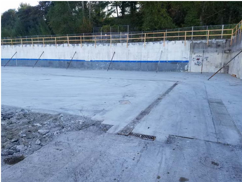
Photograph 4: Trench drain.
