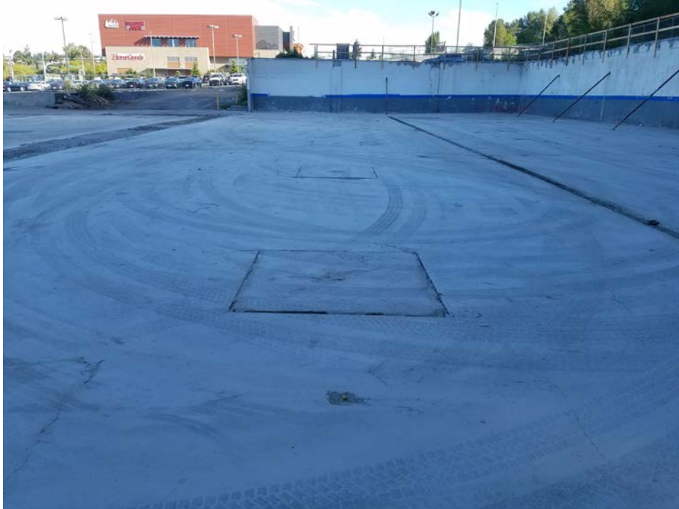
Photograph 3: Potential hydraulic hoists.
