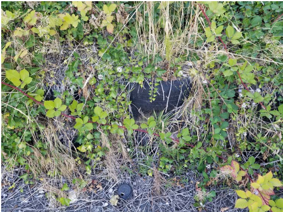
Photograph 8: Retaining wall with used tires.
