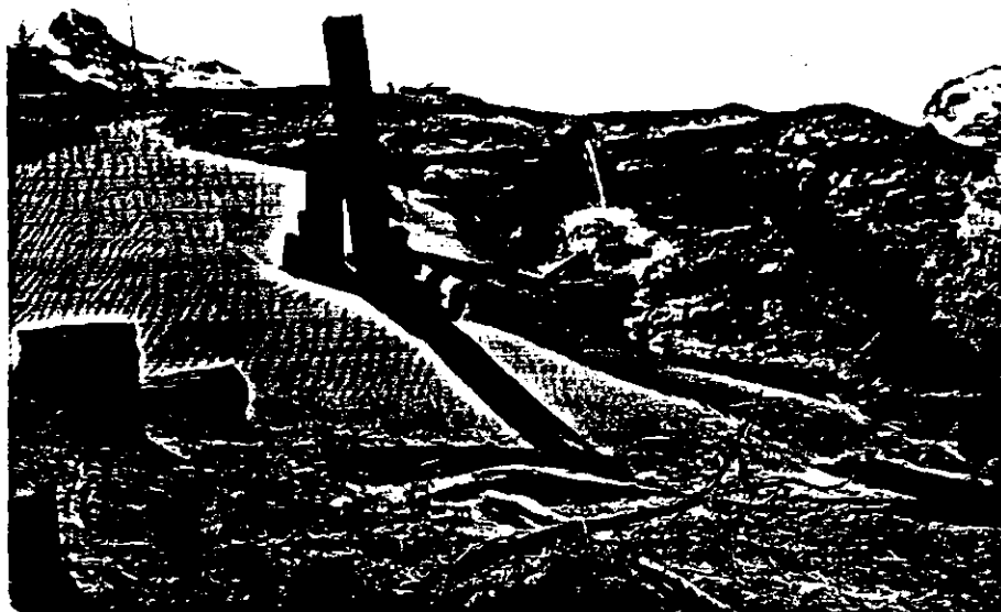
Photo No. 4. — East edge of tailings pile number 1 (photo is "off-color"). This picture shows the relative resistance to erosion of undisturbed oxidized tailings compared to wind deposited tailings. Culvert discharging stream of about 3 square inches in cross section falling 4 feet onto sloping surface of stratified tailings. Note the relatively minor erosion considering that this stream has apparently flowed, at least intermittently, for at least 20 years. No turbidity noticeable in the runoff.
