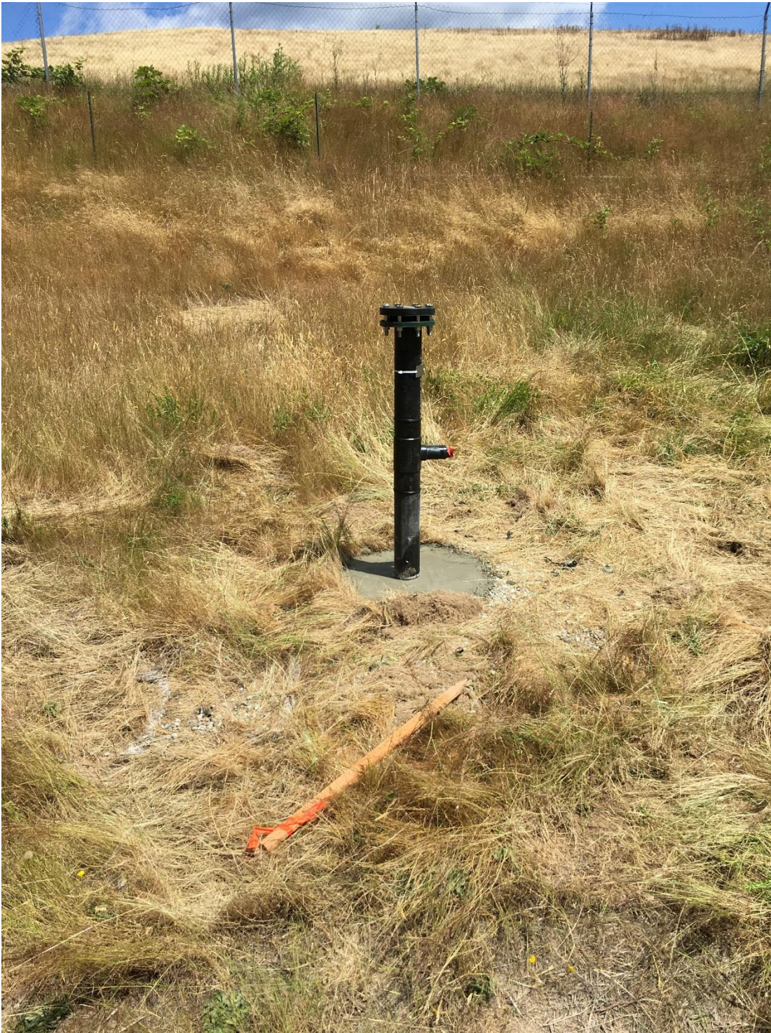
Photograph 2. View of completed extraction well GW-10, facing north up-slope.
