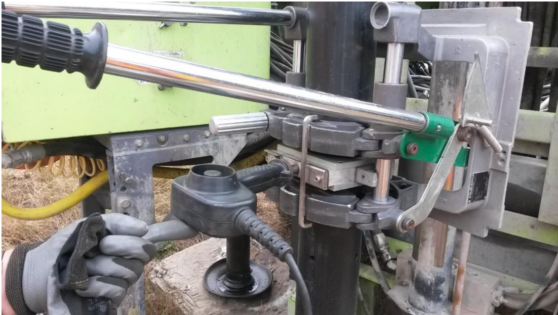
Photograph 1. Perforated section (below) being welded to blank casing (above) for GW-9
