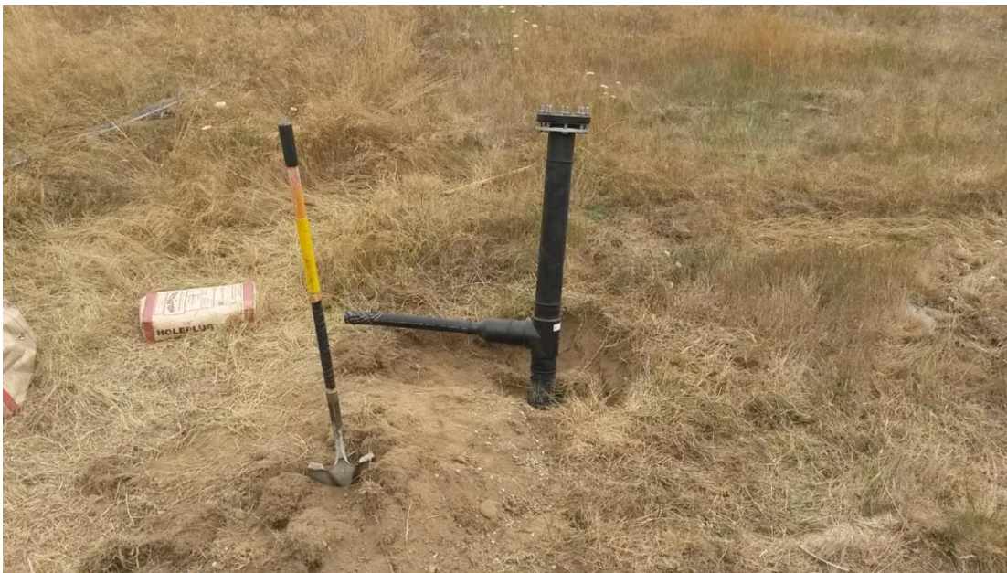
Photograph 2. Temporary wellhead completion at GW-9
