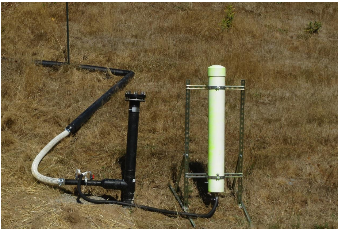
Photograph 4. Lateral connection at GW-9
