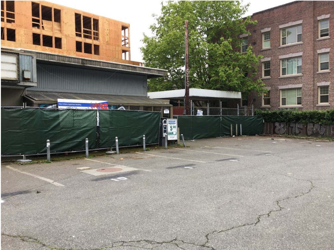
West side of the former Manhattan Express building and area that formerly housed remediation system equipment. Building visible on the right is the Del Roy Apartments.
