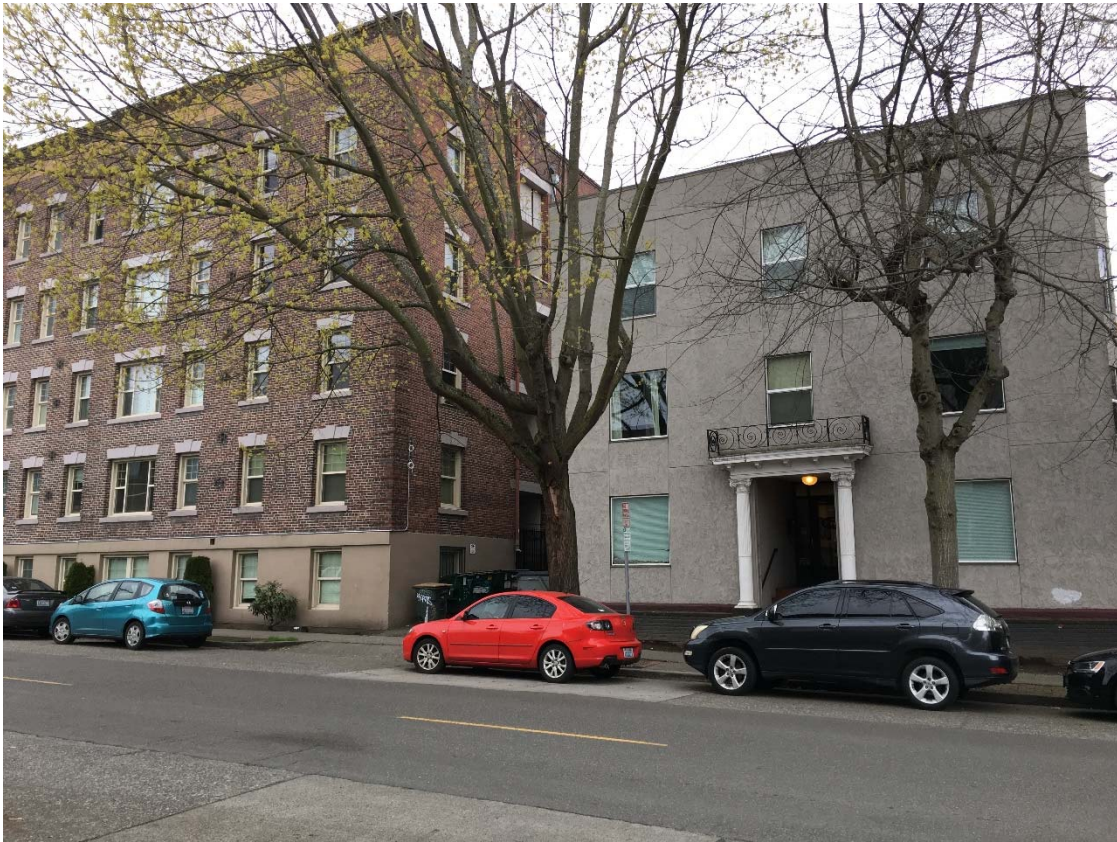
Western side of the Del Roy (left) and Monterey (right) Apartments, taken from across 1 st Avenue W.
