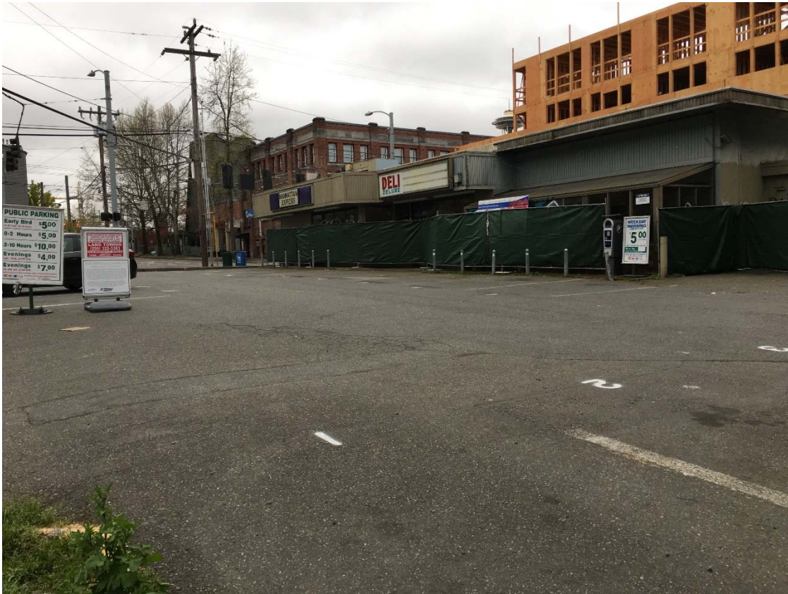
Former Manhattan Express building, with Bungalows construction visible above the building. (all photos from 4/10/19 site visit)
