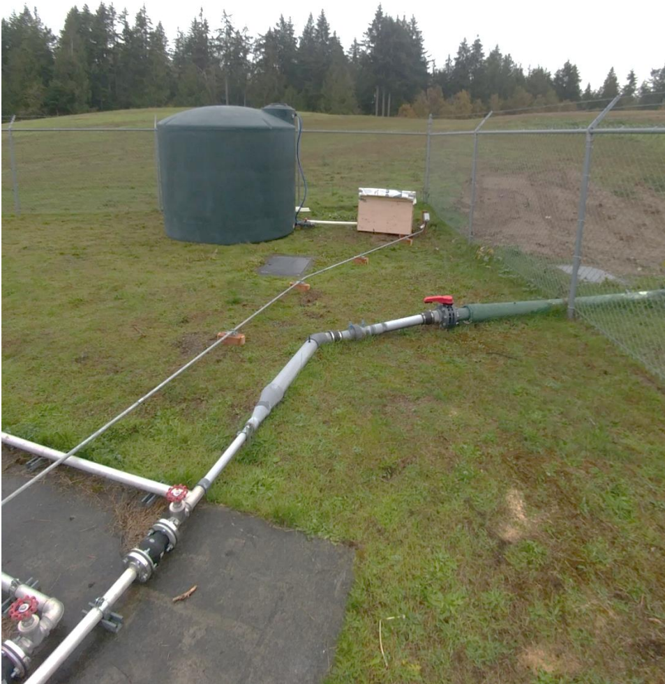
Photograph 2. Condensate system layout within flare compound
