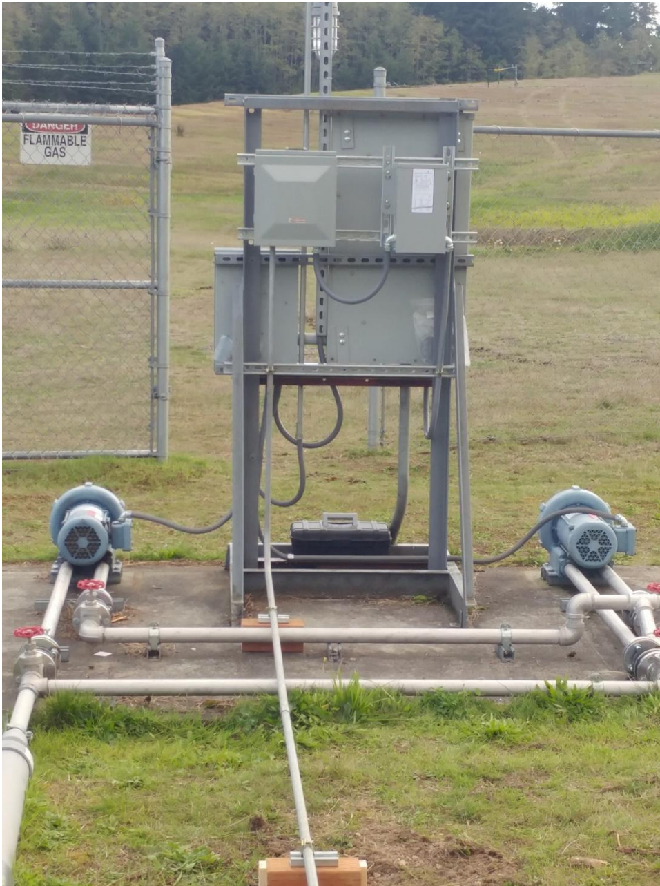
Photograph 1. Electrical connection at existing flare control panel
