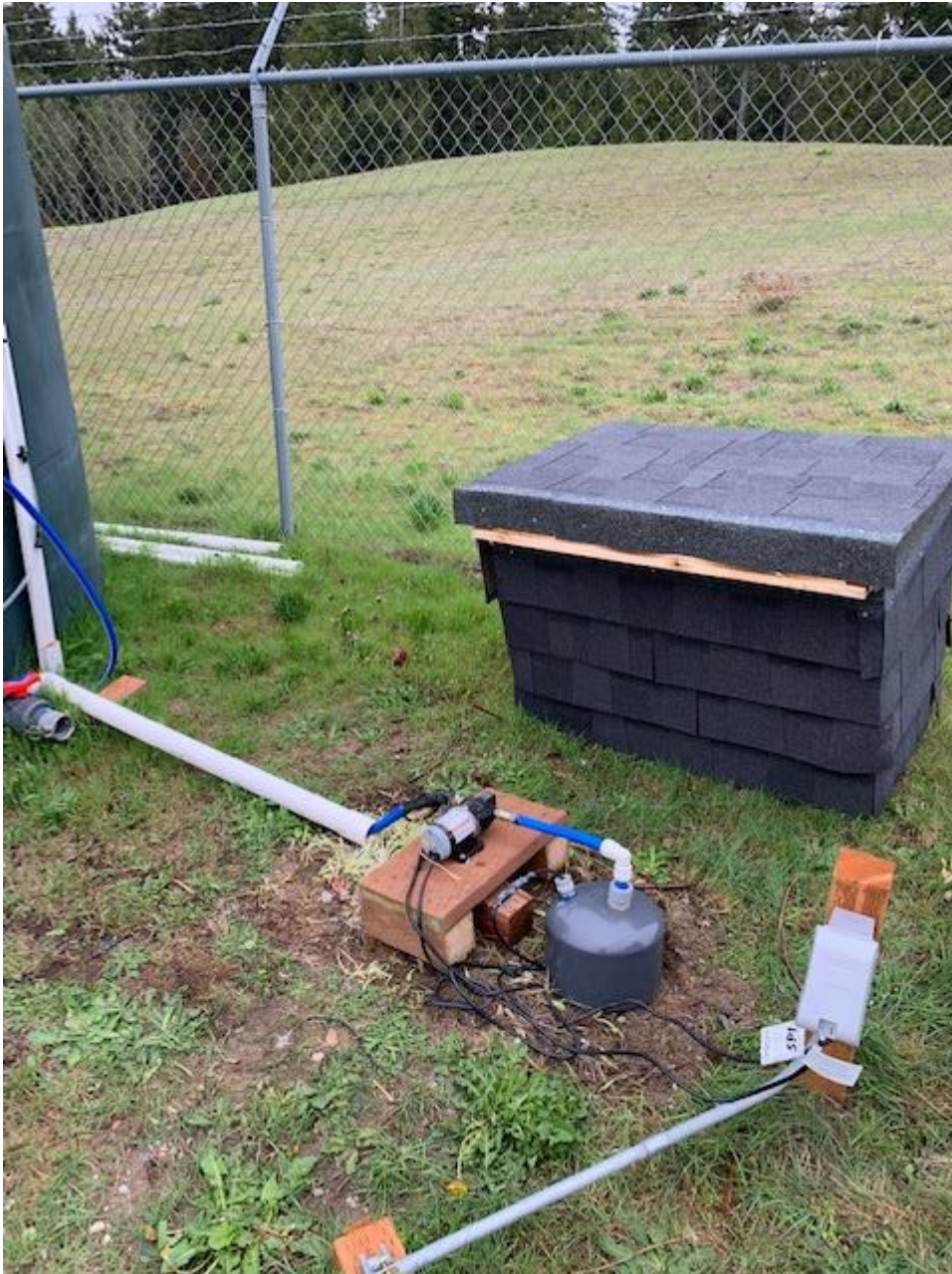
Photograph 3. Condensate sump wellhead detail
