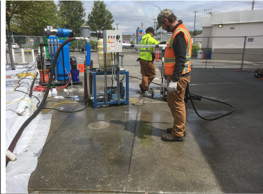
Photo #9: Inspecting wet ground for bubbles near IP-5 and SVE-1.
