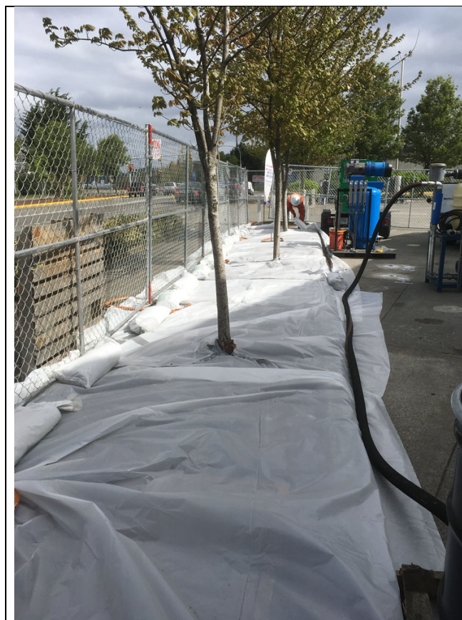
Photo #1: Setting up visqueen on gravel area adjacent to AS-1 prior to operation of the air sparge (AS) system.
