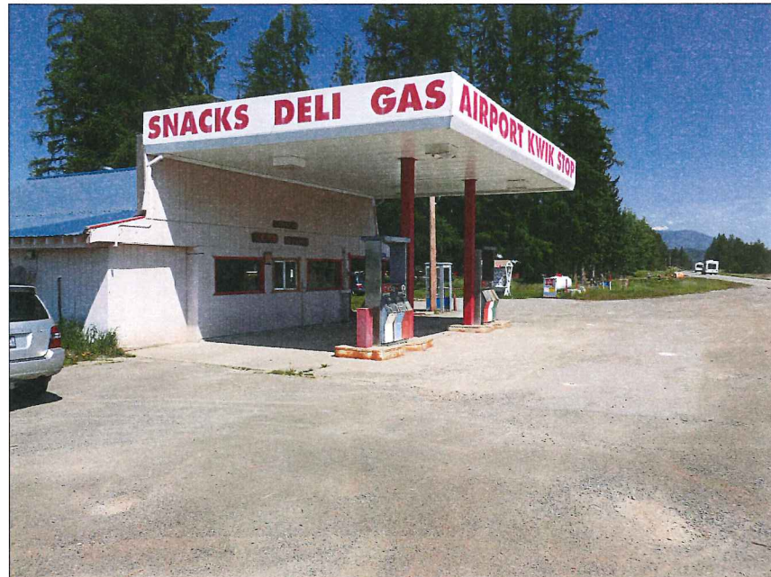
P-1 VIEW OF AIRPORT KWIK STOP FACILITY FROM THE SOUTHEAST.
