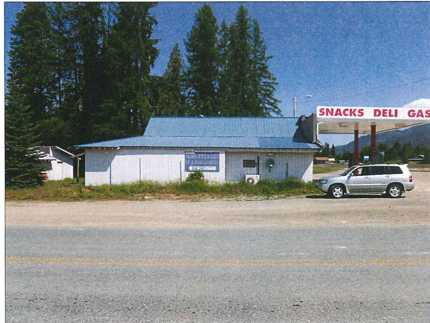
P-2 VIEW OF AIRPORT KWIK STOP FACILITY FROM THE SOUTH.
