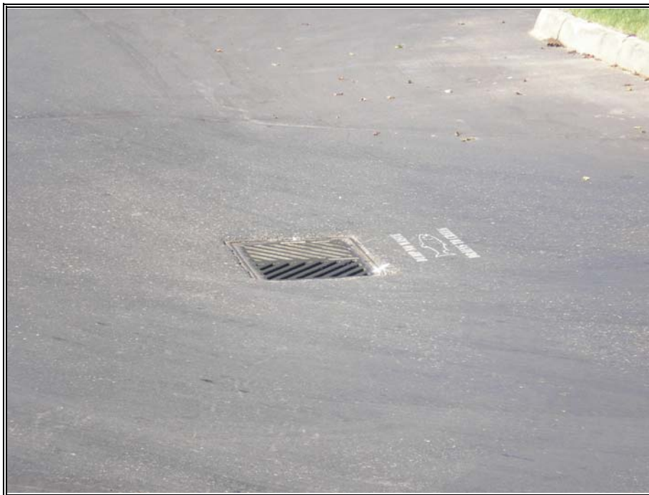
Photograph No. 5 View of typical storm drain in parking area.
