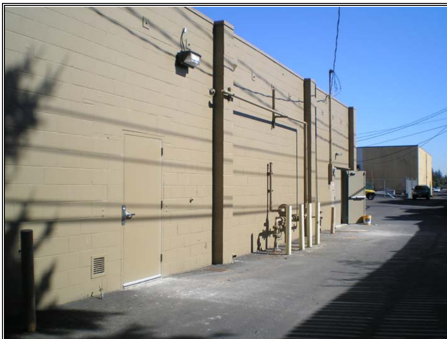
Photograph No. 2 View of south portion of site building.
