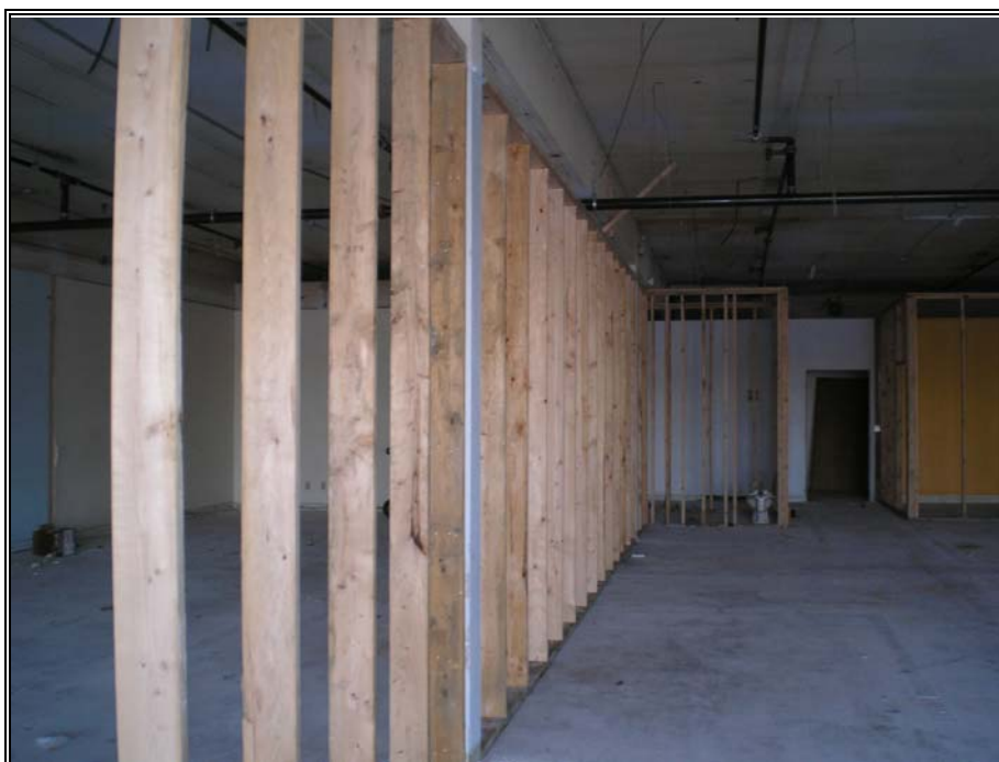
Photograph No. 4 View of vacant interior.
