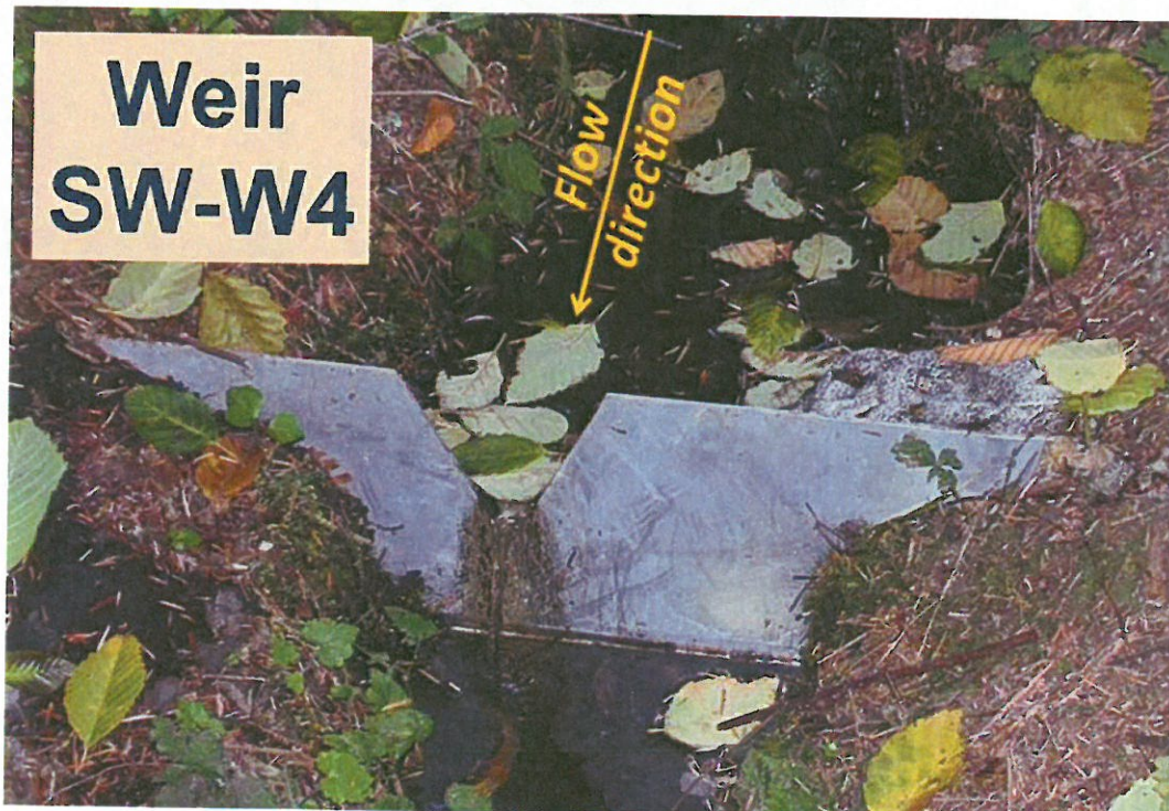
In the above photo, the inset shows how the weir used to fill up with debris and sediment during a high rainfall event. The newer weir has not had the problem.
