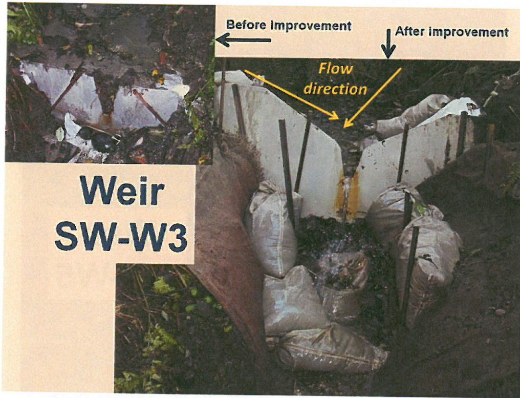
In the above photo, the inset shows how the weir used to fill up with debris and sediment during a high rainfall event. The newer weir has not had the problem.
