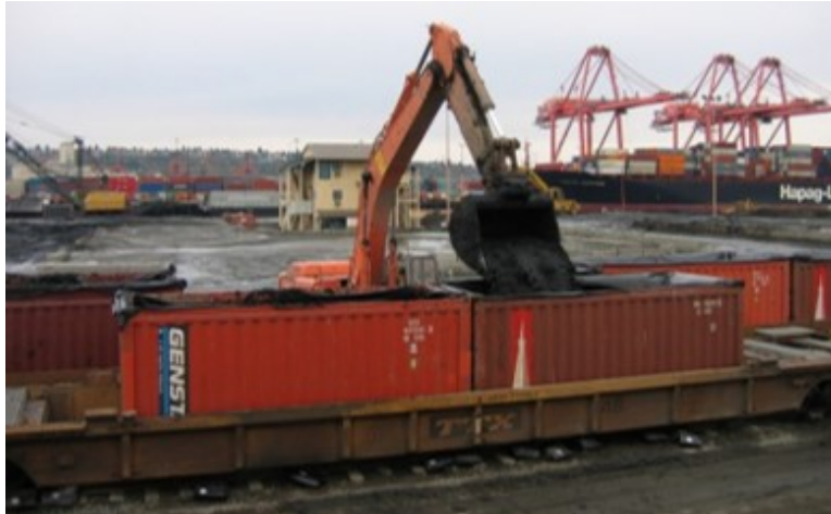
Exhibit 11. Land-based mechanical excavator
