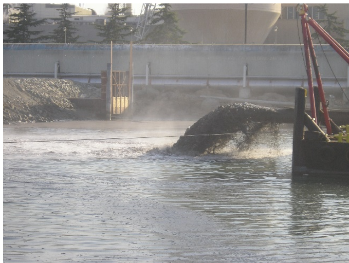
Exhibit 9. Hydraulic dredge slurry
