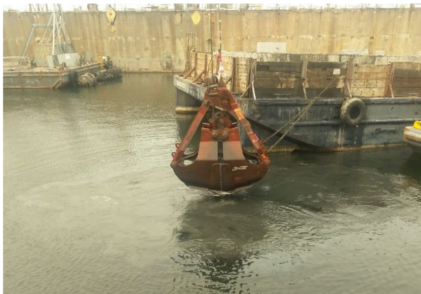
Exhibit 7. Mechanical dredge digging bucket
