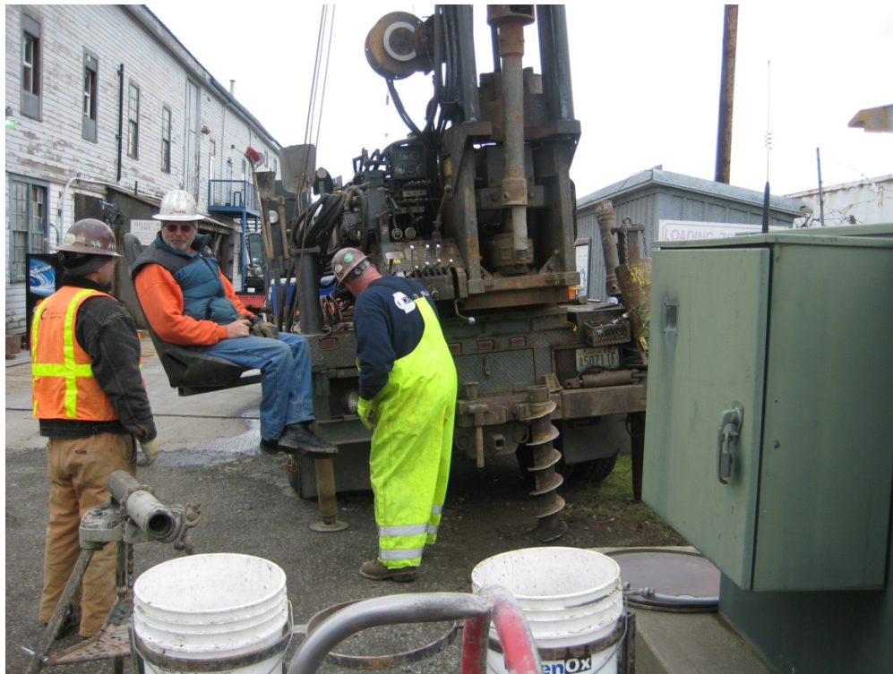
Photograph 10. View of auger rig installing Monitoring Well MW-06, March 2011.
