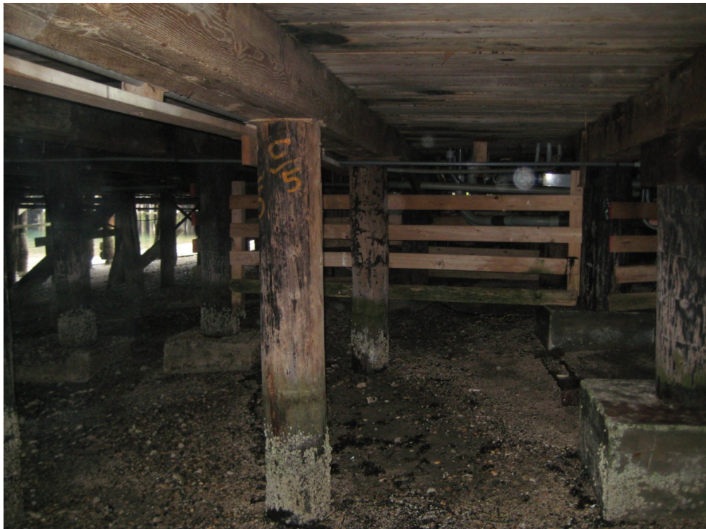
Photograph 20. View looking east underneath Loft and Pier Shops, April 2013.
