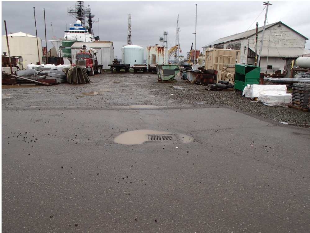
Photograph 26. AOC 3 and AOC 2 - central area of the Site.
