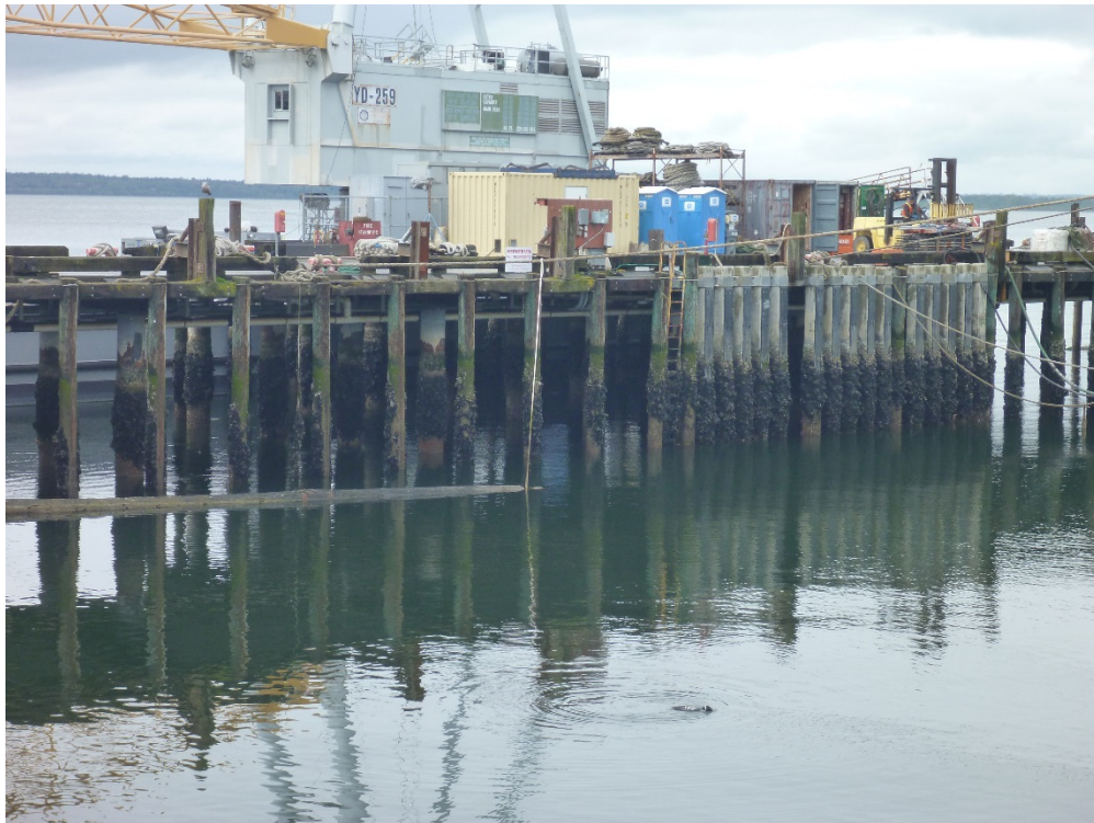
Photograph 48. Sediment Units 5 and 3A.
