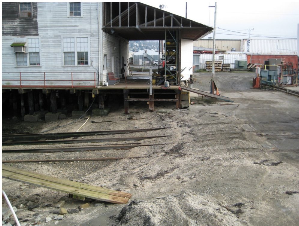
Photograph 2. View of the Marine Railway and shoreline area facing east, January 2013.
