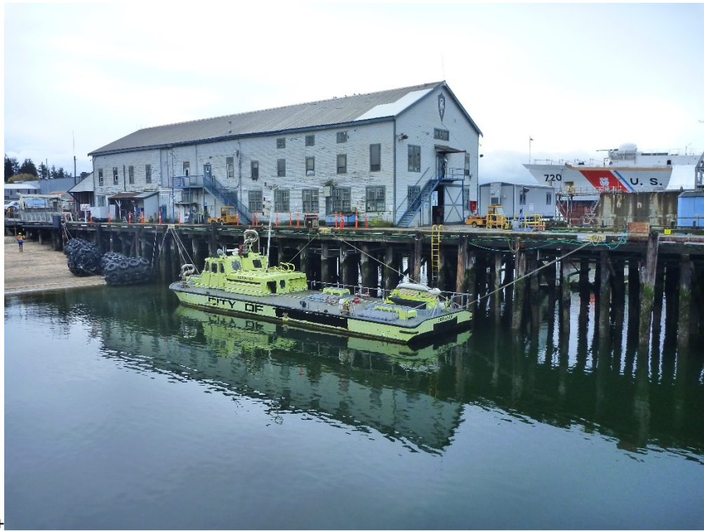
Photograph 37. Sediment Units 1 and 3A.
