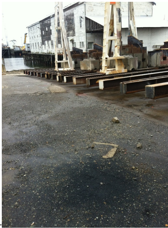
Photograph 23. AOC 2 looking north.
