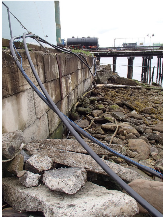
Photograph 54. Sediment Unit 8 and bulkhead wall.
