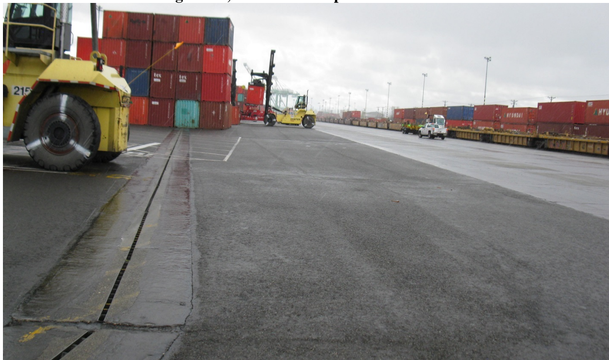
Photo 7: Container Storage Area, Resurfaced Cap Area and Slot Drain – From the North
