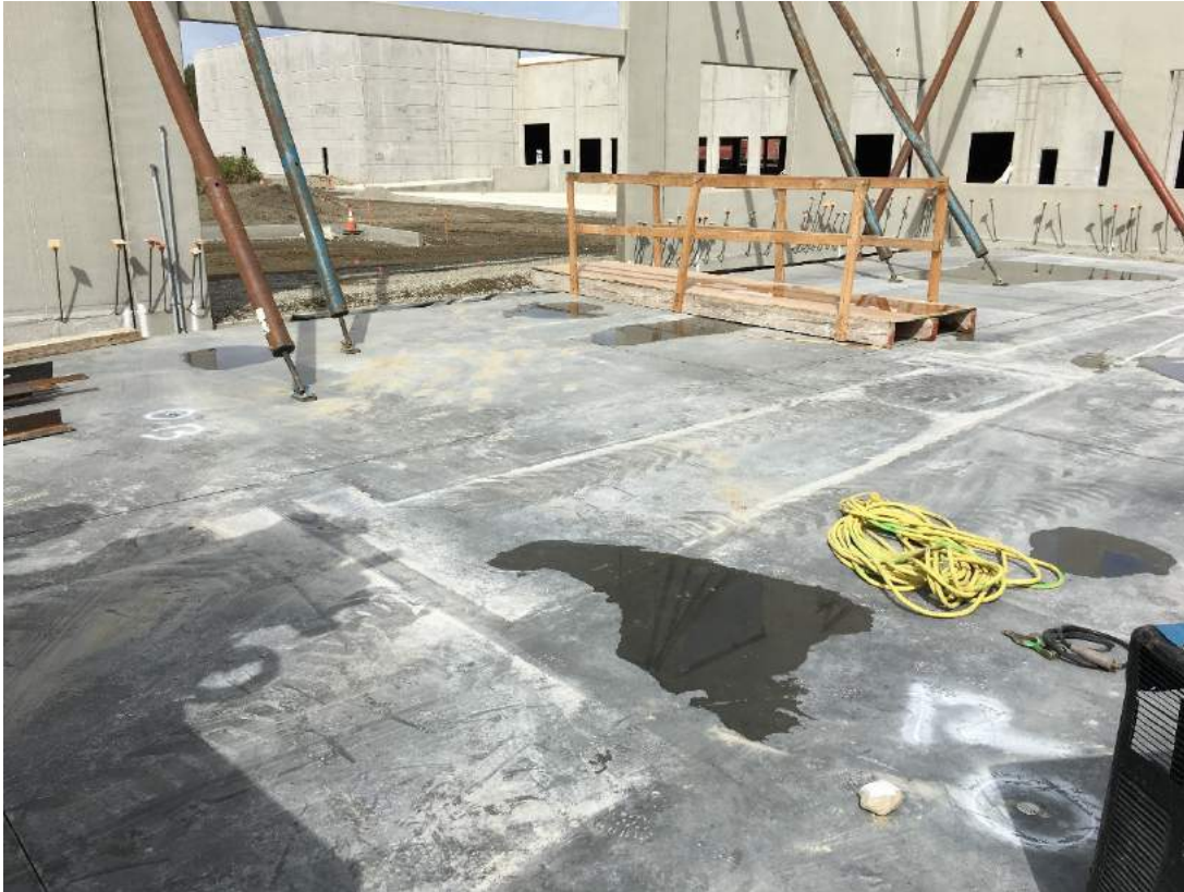
Vapor Pins VP-12 and VP-13 adjacent to northwest office in Building B in Ecology adjusted locations. Looking north-northwest
