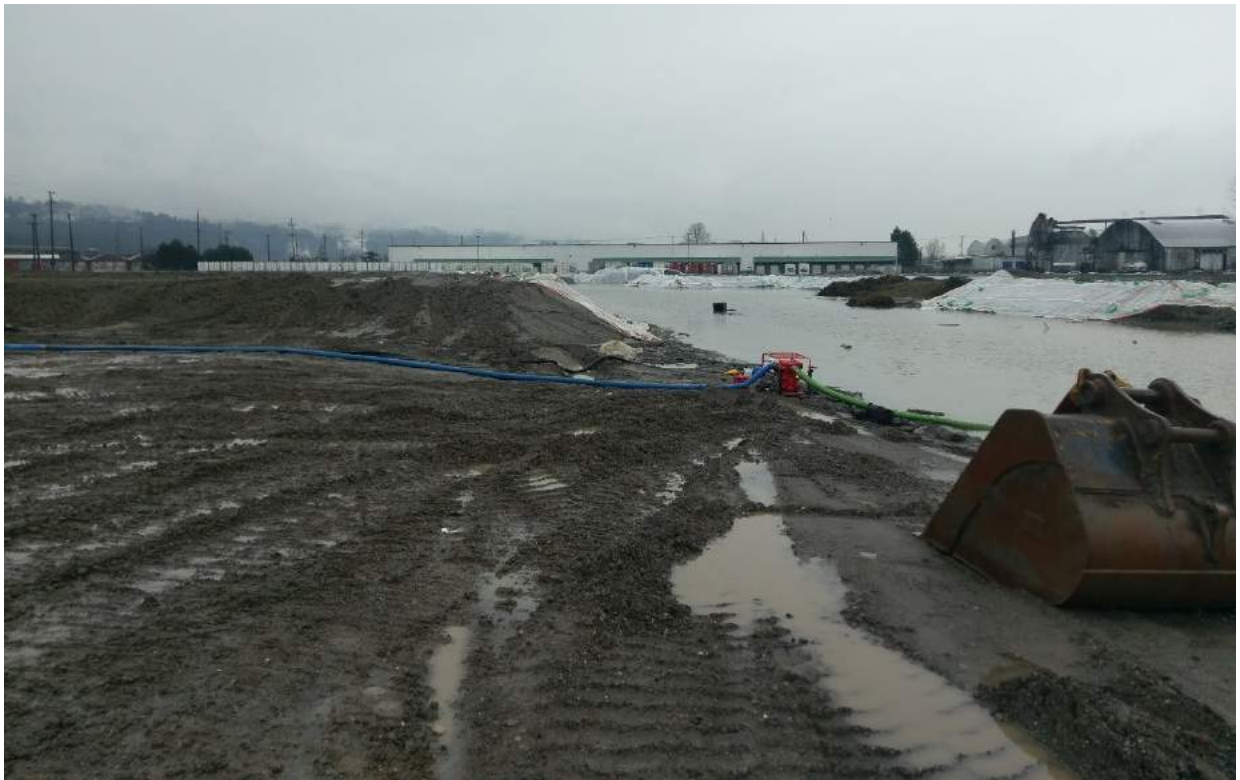
Photograph 6. Stormwater pump brought in to control excess water in the stormwater pond. Looking South
