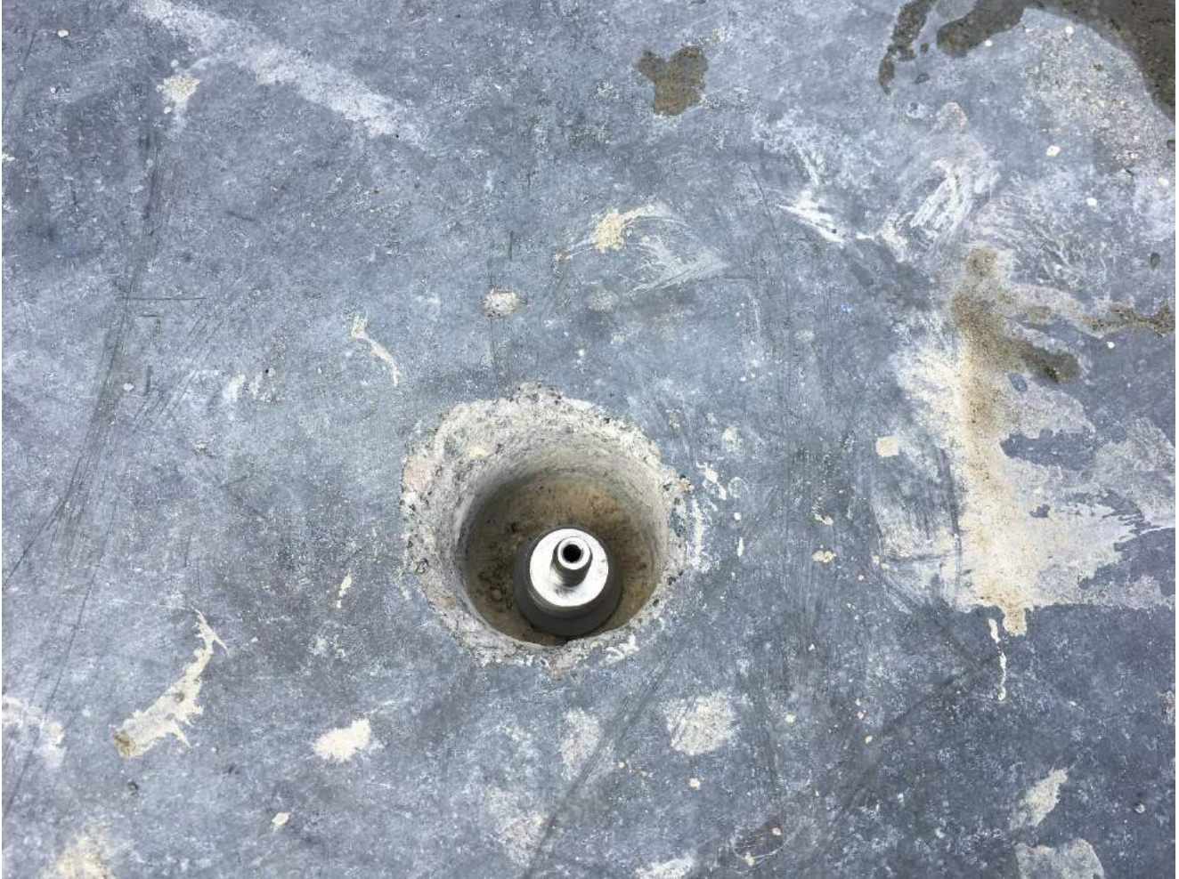
Vapor Pin VP-14 prior to capping and installing the flush-mounted cover.
