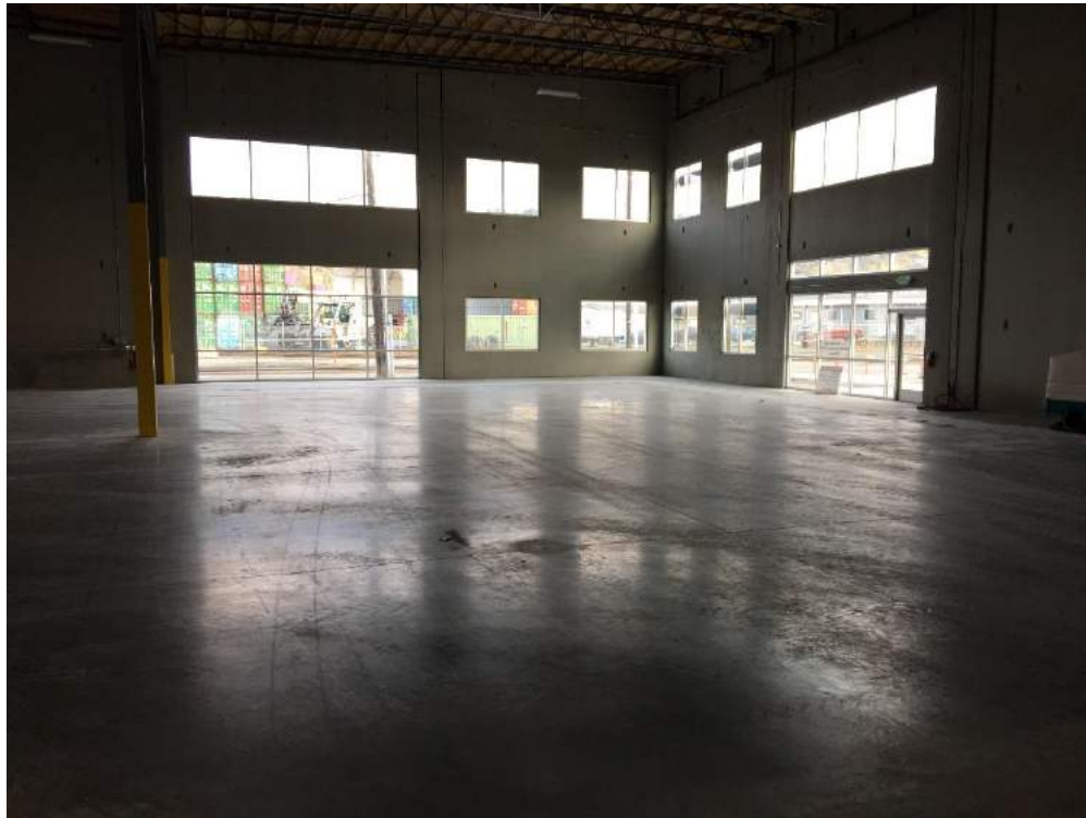
Photograph 7. Building A interior; northeast office node.
