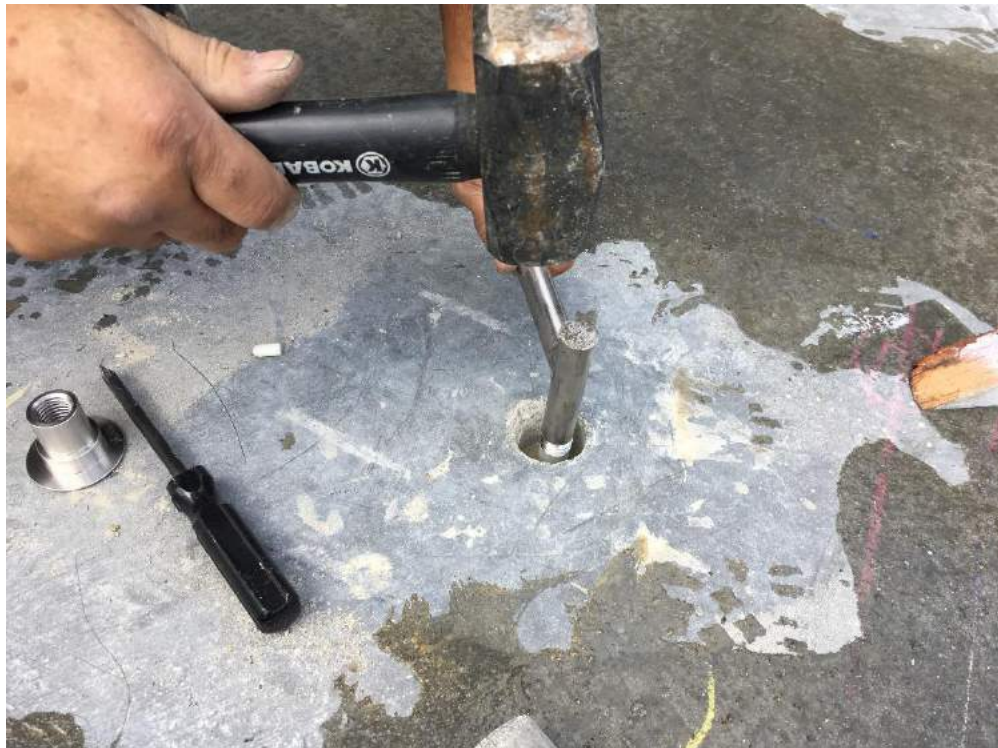
Photograph 2. Hammering vapor pin in place.
