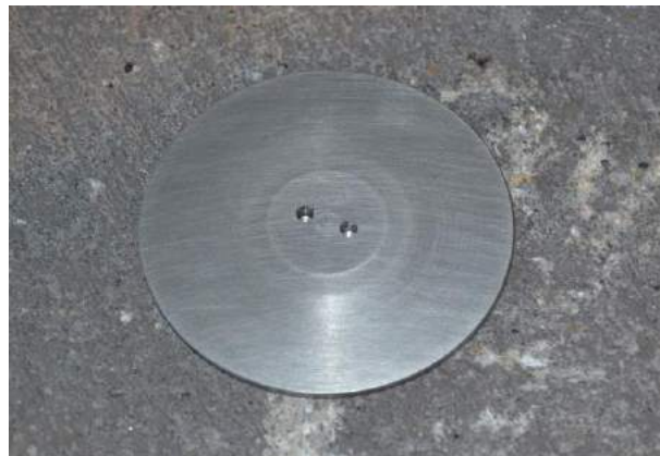
Figure 4. Secure Cover Installed
