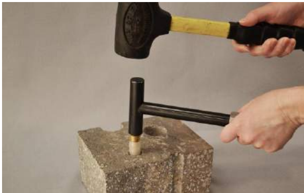
Figure 2. Installing the VAPOR PIN®
