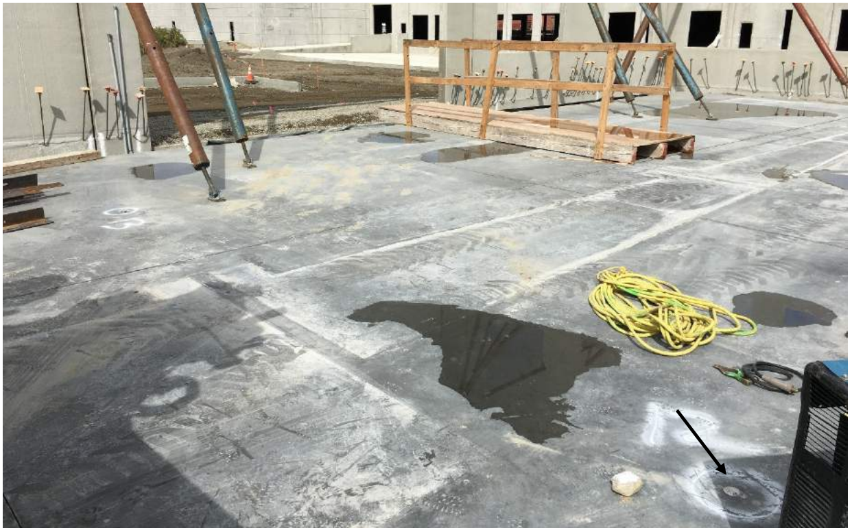
Photograph 14. Vapor Points VP-12 and VP-13 after installation.
