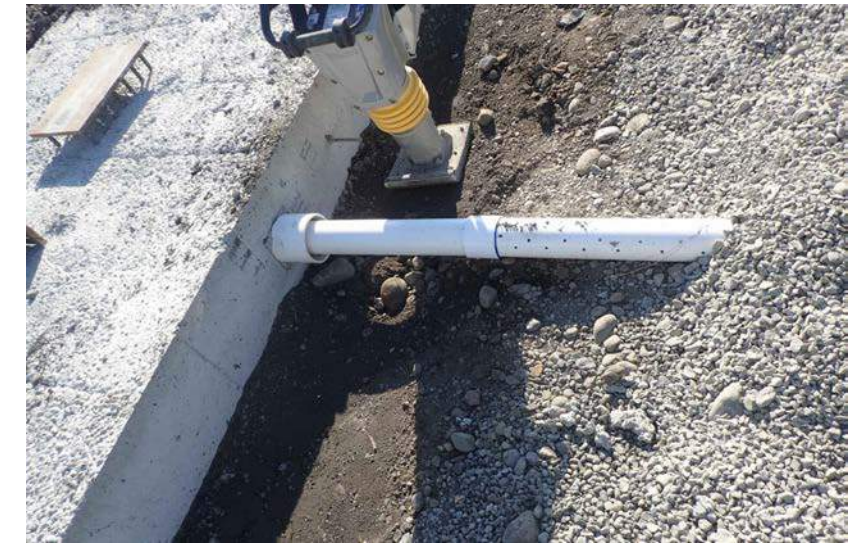
TYPICAL COLLECTION PIPE TROUGH GRADE BEAM PHOTO SCALE: NTS
