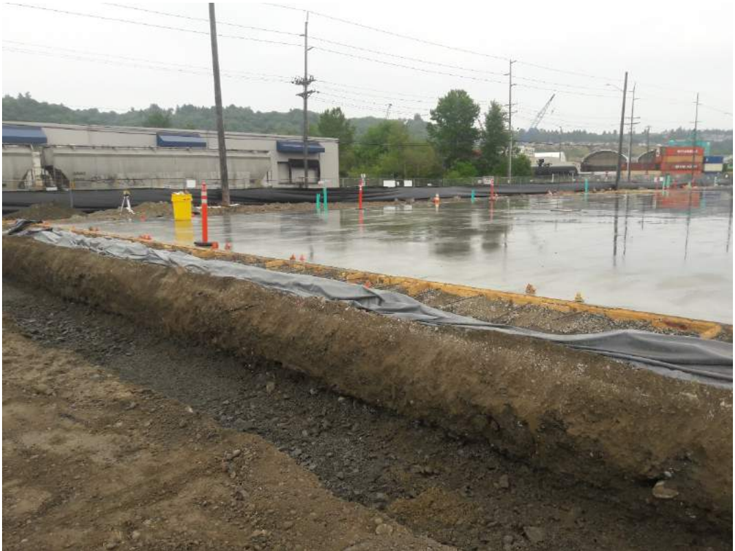
Photograph 10. Excavation of perimeter footing around recently poured floor.
