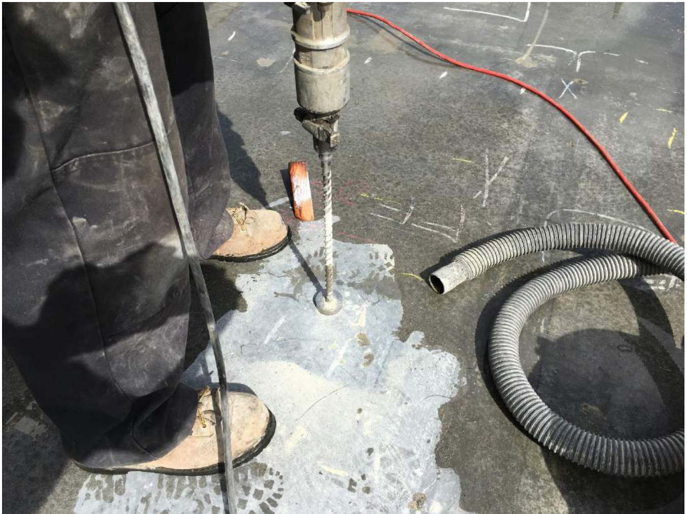
Installation of a Vapor Pin.
