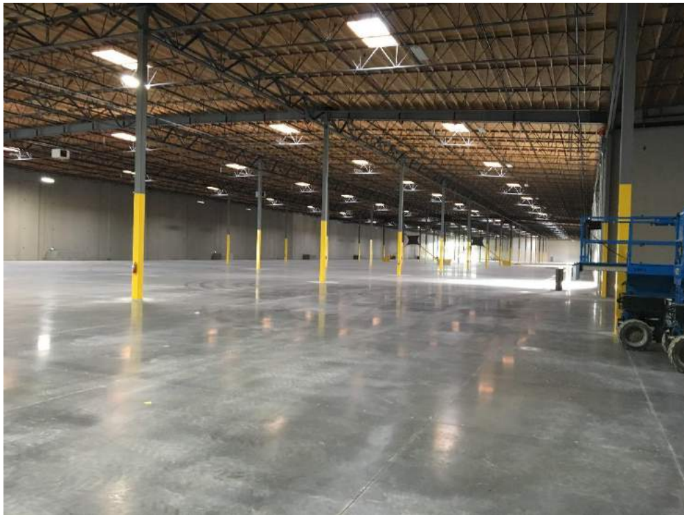
Photograph 10. Building A interior; southwest corner facing east.
