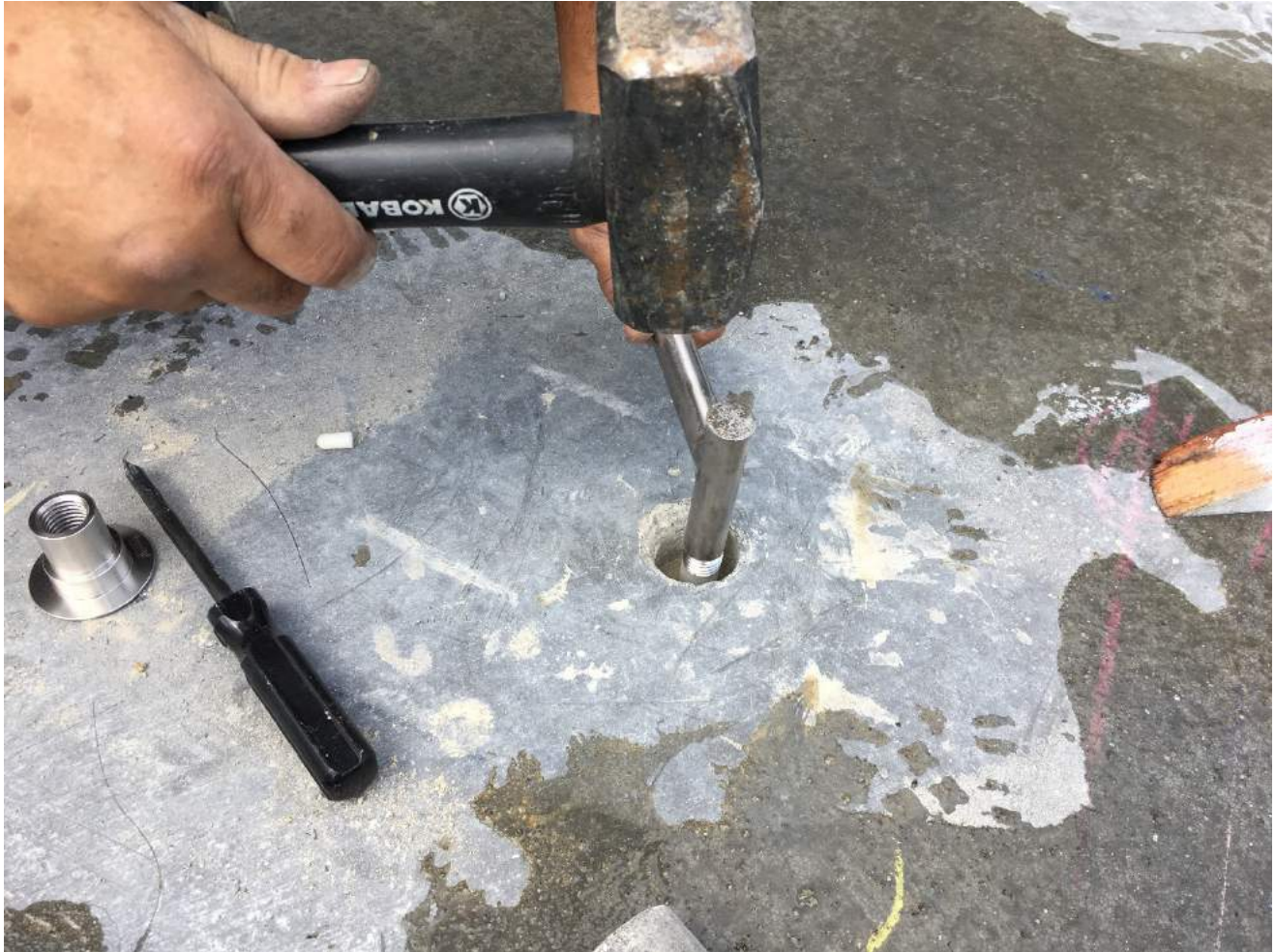
Hammering in Vapor Pin VP-14.
