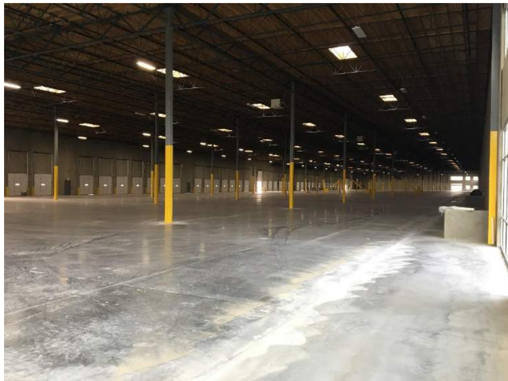
Photograph 6. Building A interior; northeast corner facing west.
