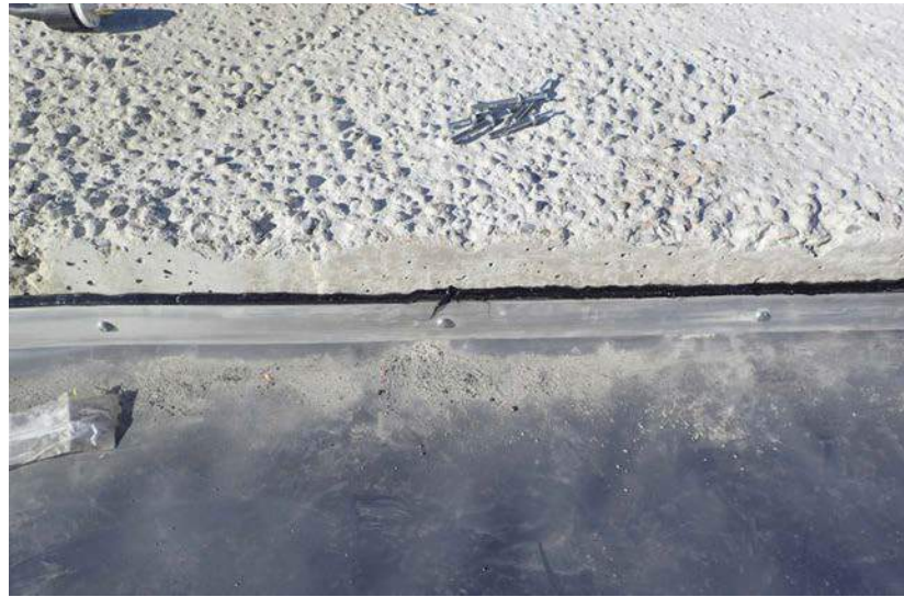
TYPICAL BATTEN STRIP SEAL PHOTO SCALE: NTS
