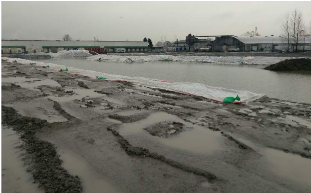
Photograph 5. Wet site conditions during initial methane and VOC vapor survey in April 2018. Stormwater Pond in Background, Looking North
