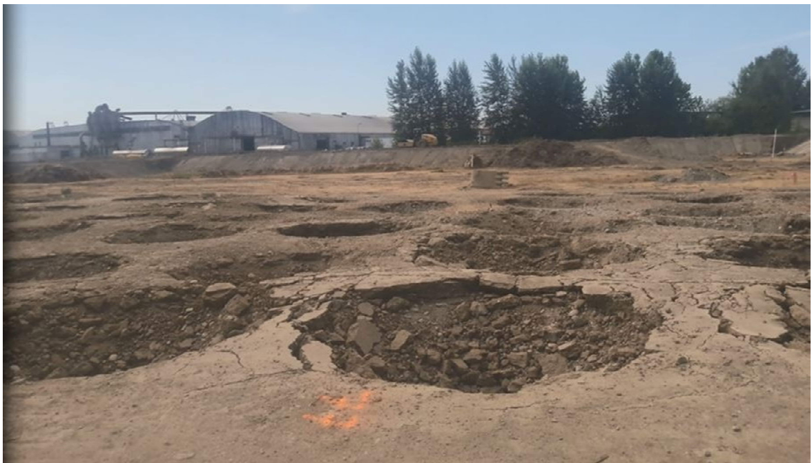
Photograph 2. Dynamic Compaction Impact Craters. Looking South
