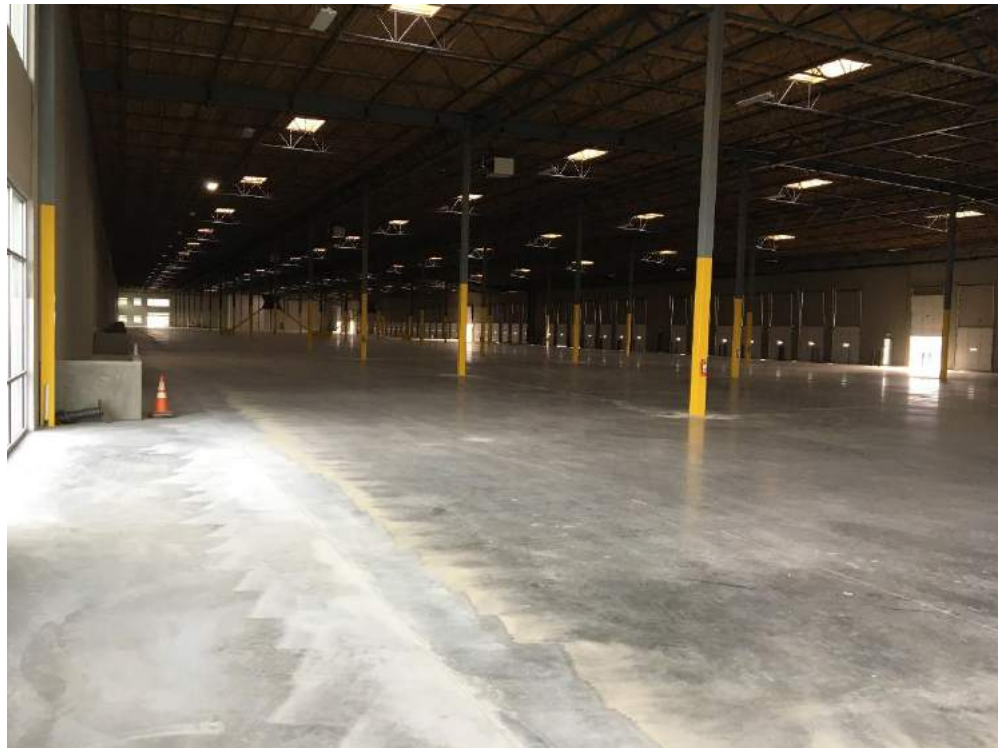
Photograph 8. Building A interior; northwest corner facing east.
