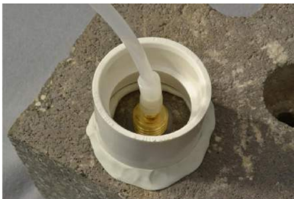
Figure 6. Water dam used for leak detection
