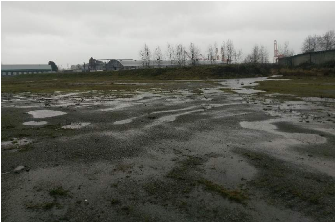
Photograph 1. Preconstruction Site Conditions. Looking south, existing surcharge pile in background.
