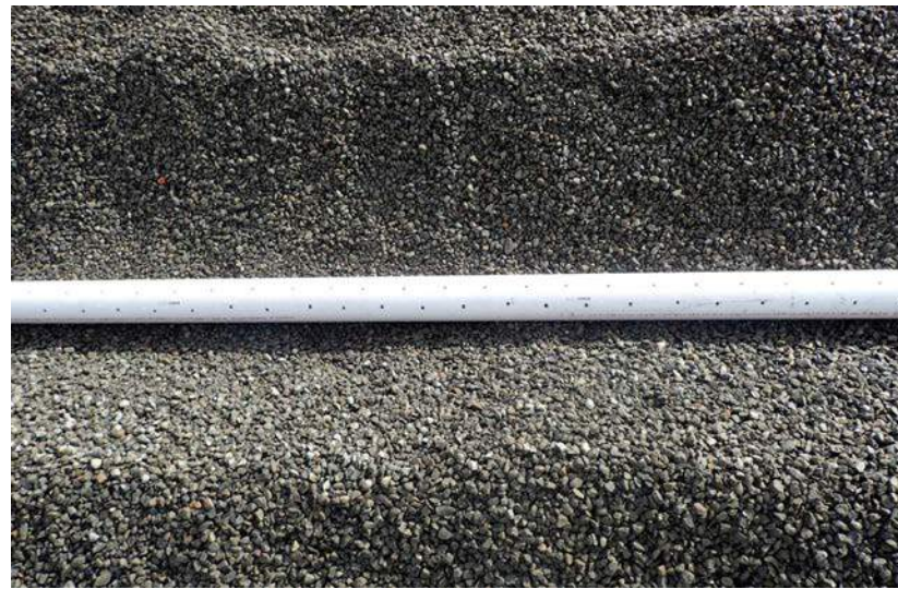
TYPICAL PERFORATED COLLECTION PIPE PHOTO SCALE: NTS
