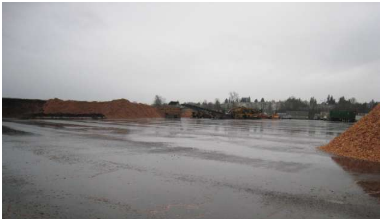
Photo 2: Paved containment area - from the east
