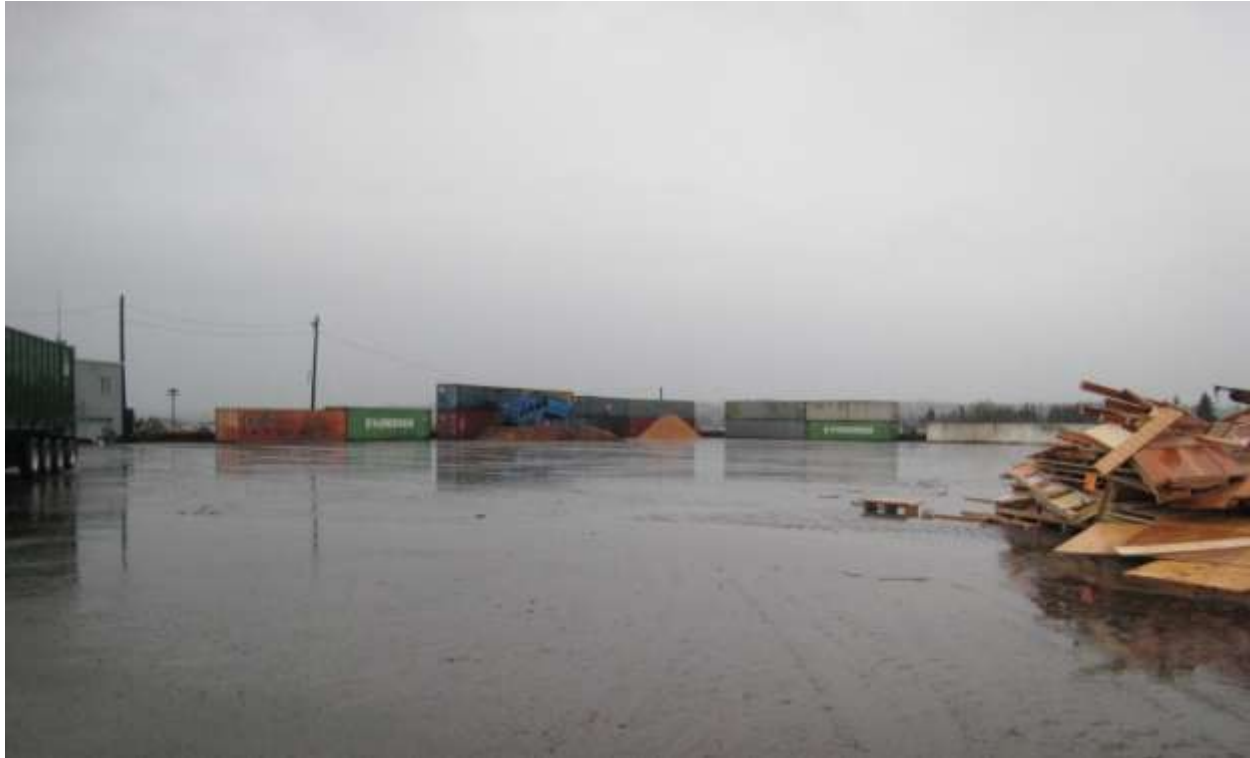
Photo 1: Paved containment area - from the west
