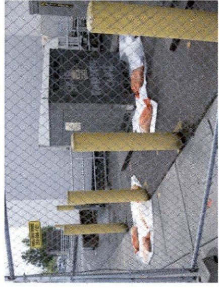
South transformer unit, plastic on ground covering oil & staining, pending cleanup.
