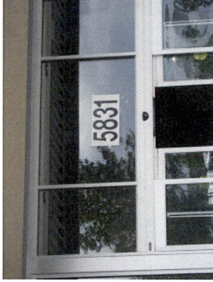
Store front facing south, to west of bldg demo.
