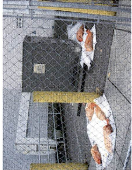
Spill at south transformer unit.
