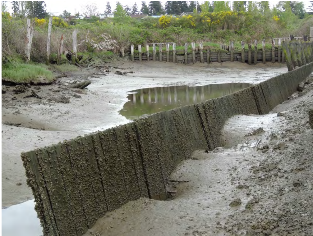
Photo 1: Tidally influenced “Finger Area” – looking approximately easterly (Ecology Photograph)
