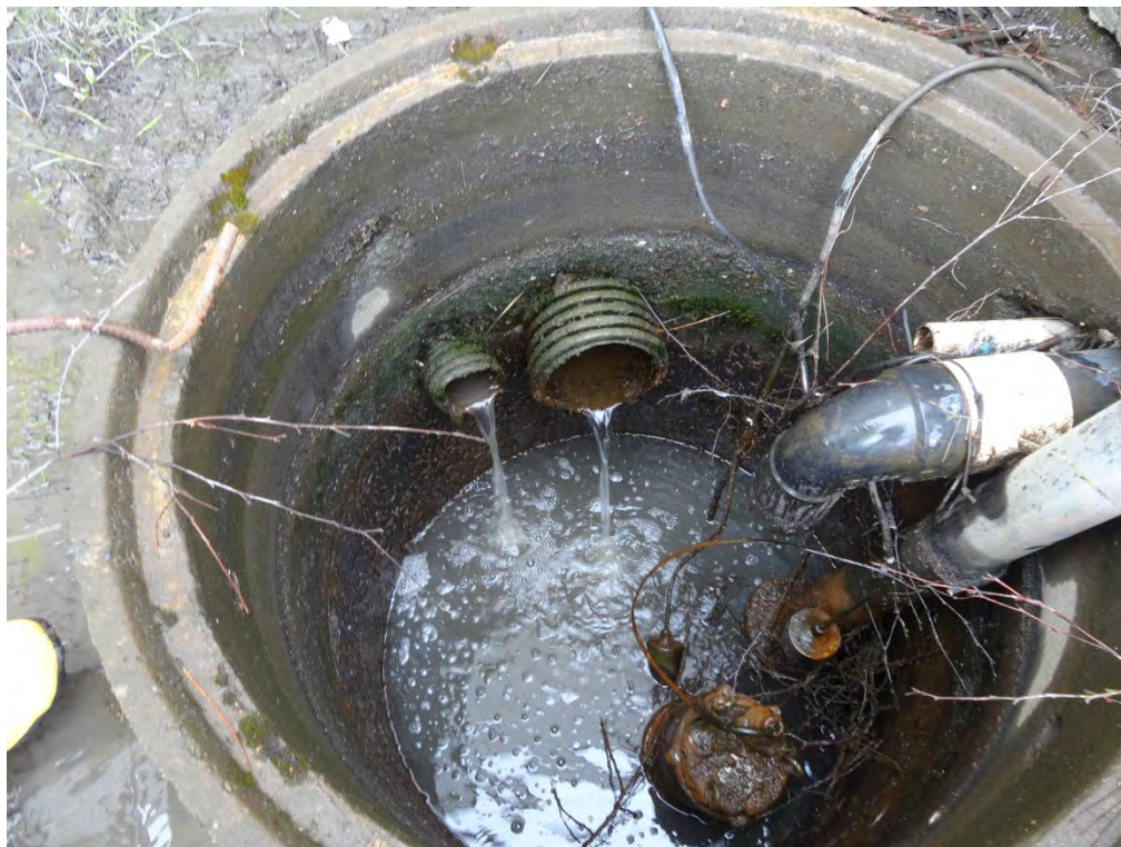
Photo 2: North truck dock area sump (Ecology Photograph)
