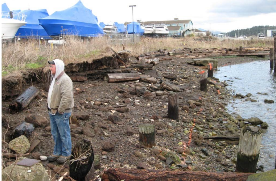
Photograph 2 Zone 1 – Before emergency action implementation.
