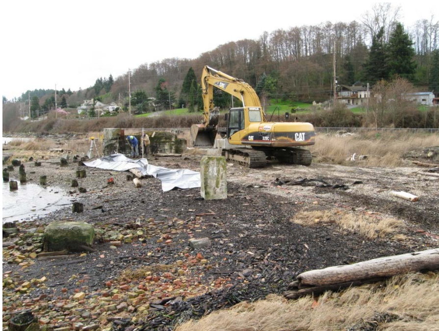
Photograph 7 Zone 2 – Before emergency action implementation.
