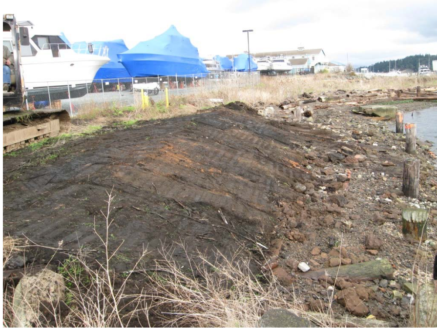
Photograph 4 Zone 1 – Final grade before geotextile is laid down.
