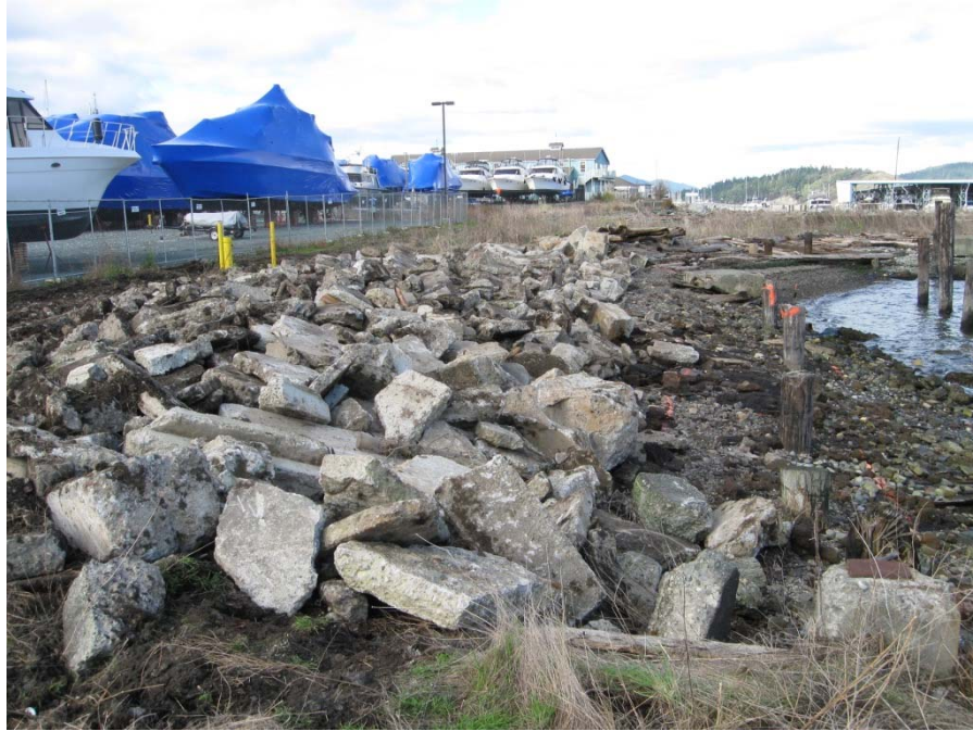
Photograph 6 Zone 1 – Emergency action implementation complete.
