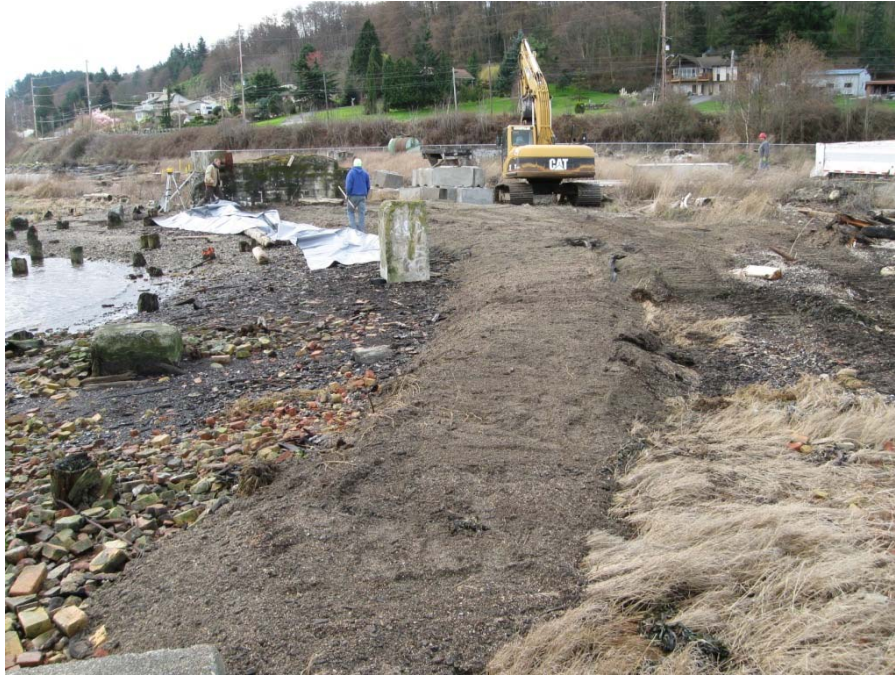
Photograph 8 Zone 2 – Berm transect line being leveled.
