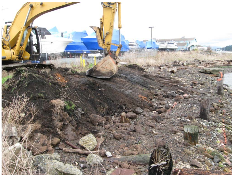
Photograph 3 Zone 1 – During emergency action implementation.
