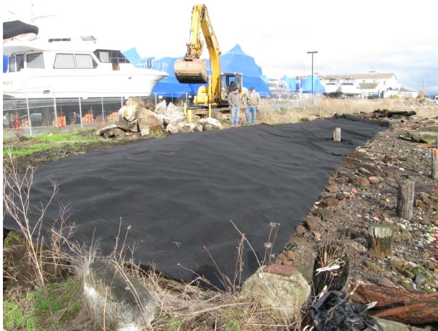
Photograph 5 Zone 1 – Geotextile completely rolled out.
