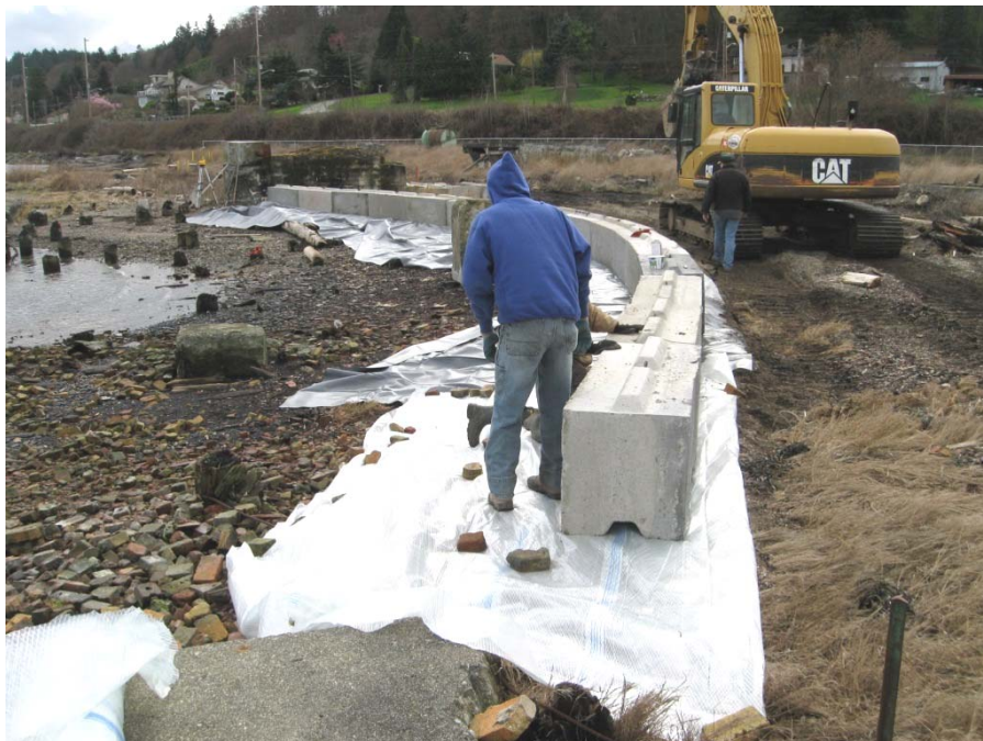
Photograph 9 Zone 2 – Placement of Ecology blocks along transect.
