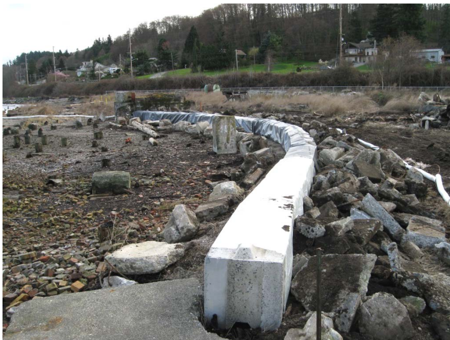
Photograph 11 Zone 2 – Emergency action implementation complete.
