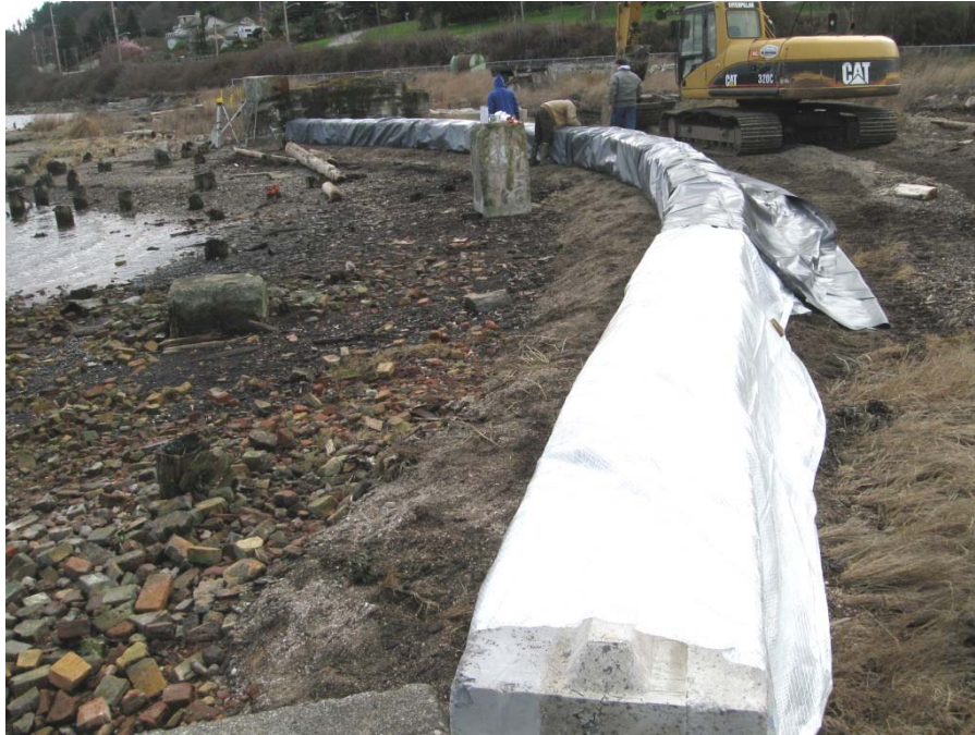
Photograph 10 Zone 2 – Folding the PVC liner over the Ecology blocks.
