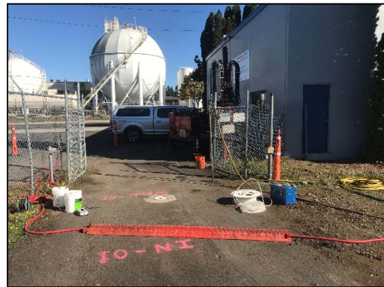
Photo 4: Injection setup and water well monitoring equipment.
