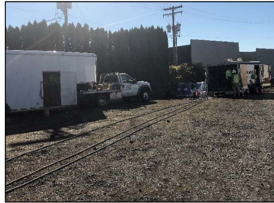
Photo 2: Drill rig storage and injection trailer location – hose length setup.
