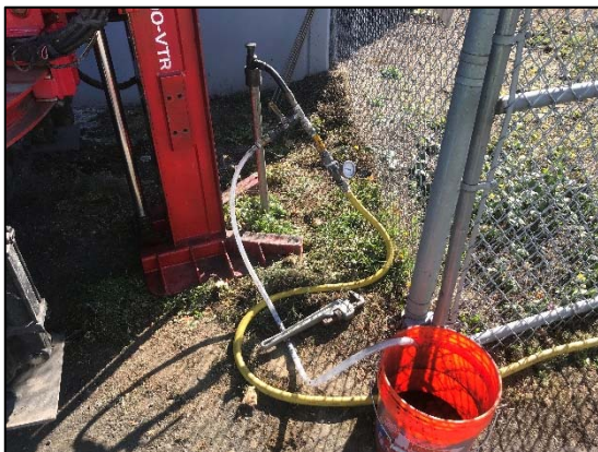
Photo 5: Injection cap and pressure relief bypass.
