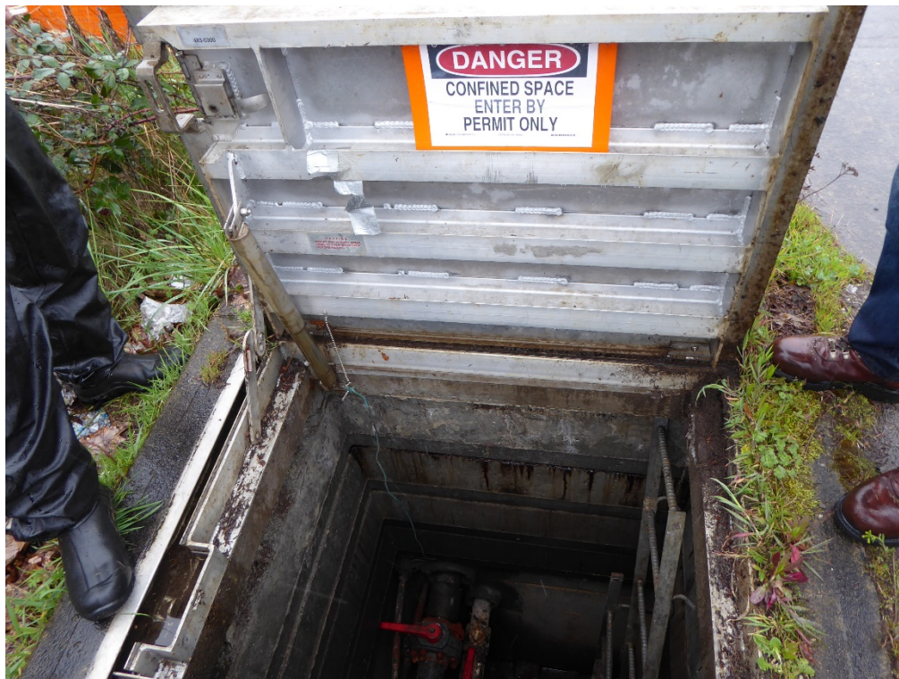
Containment vault CV-9
