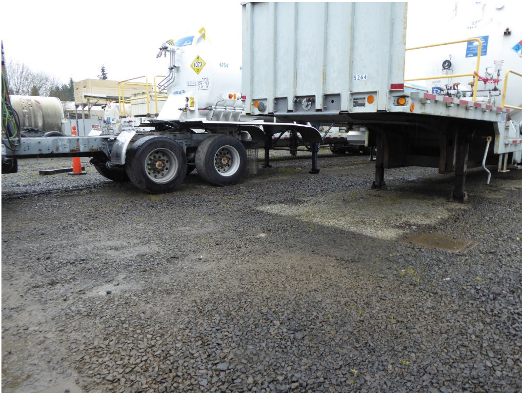
Infiltration gallery on Linde property
