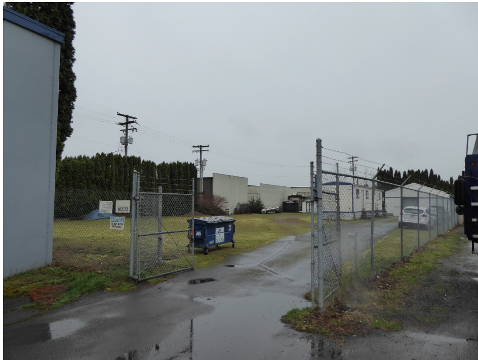
Fenced entry to Boomsnub property
