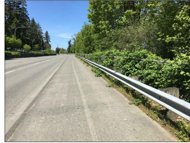
P-3 CF-2 VIEW NORTHWEST - EAST MARINE VIEW DRIVE
