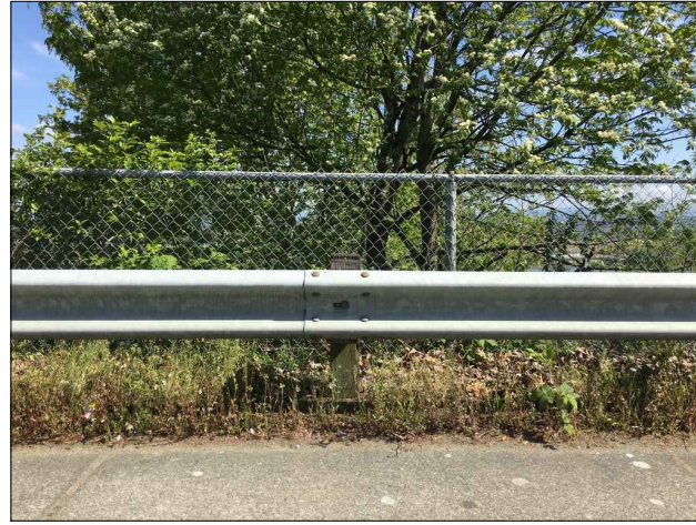
P-2 CF-2 VIEW NORTHWEST - EXISTING 4-FT CHAIN LINK FENCE AND GUARDRAIL
