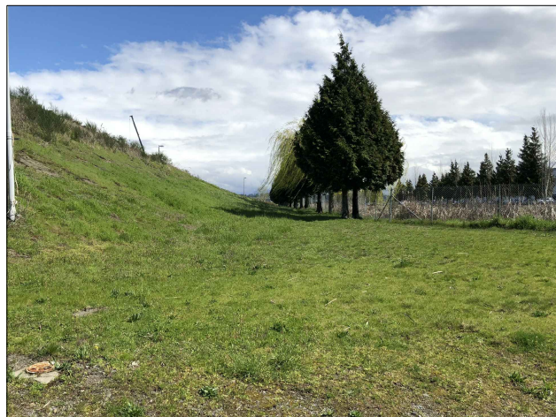
P-9 CD-2 VIEW EAST - RIVERSIDE ROAD SOUTH EMBANKMENT
