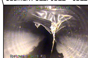
BROKEN PIPE AT 19 FT FROM CB11
