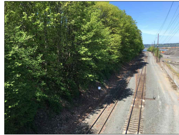
P-7 CF-2 VIEW NORTHWEST - RAILROAD TRACKS EAST OF AREAS C2 AND C3
