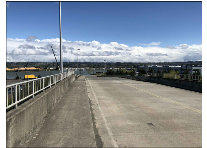
P-8 CD-2 VIEW EAST - RIVERSIDE ROAD BRIDGE APPROACH
