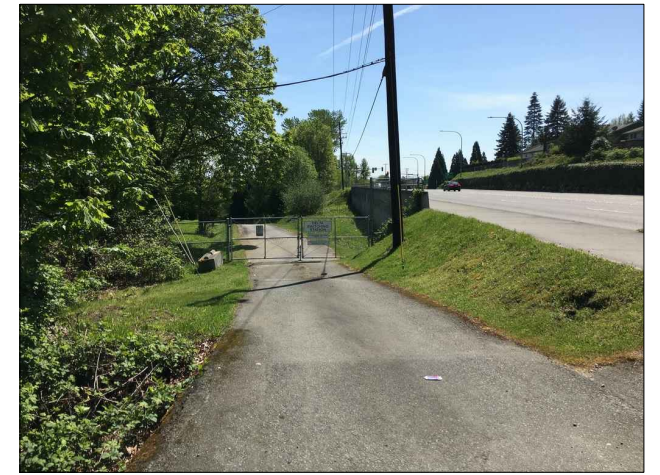
P-8 CF-2 VIEW SOUTHEAST - PUD DELTA SWITCHING STATION ACCESS ROAD GATE
