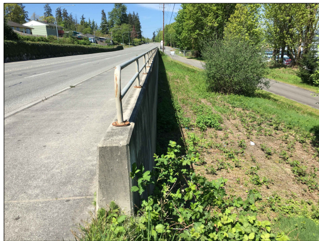
P-9 CF-2 VIEW NORTHWEST - RETAINING WALL AND RAILING
