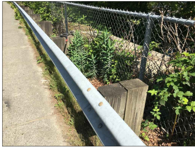
P-5 CF-2 VIEW NORTHWEST - GUARDRAIL AND FENCE
