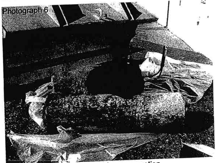
USTs 1 & 2 following removal from excavation
