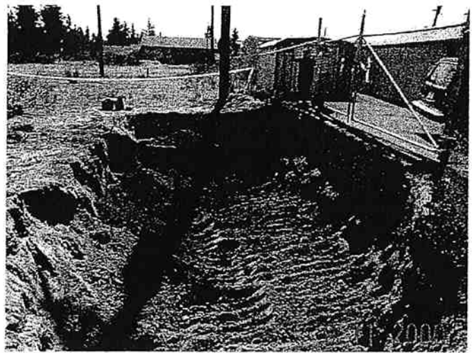
View of 4 foot BGS excavation from the north.
