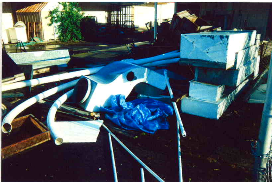
Photo 8: Loading dock area located immediately south of the spray painting shed.
