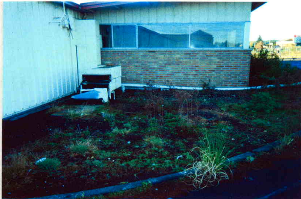
Photo 6: Location where two 80-gallon Kerosine USTs were removed
