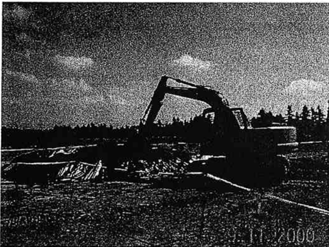
PCE contaminated stockpile contained in a plastic-lined berm area.
