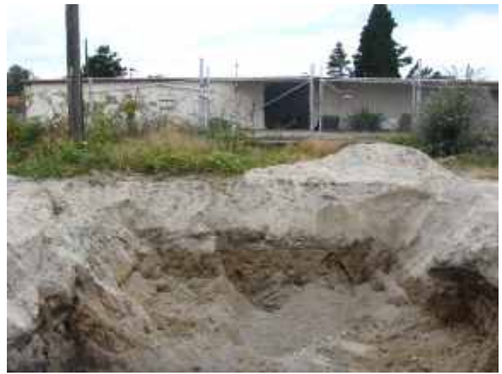
Photograph 04: Excavation area - View West
