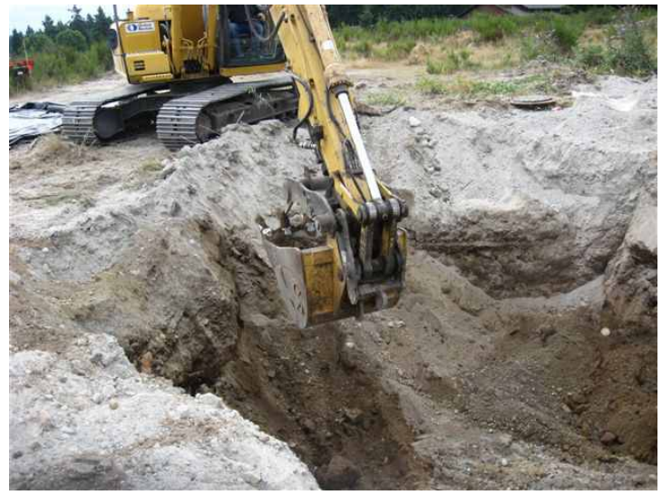
Photograph 02: Excavation of soil
