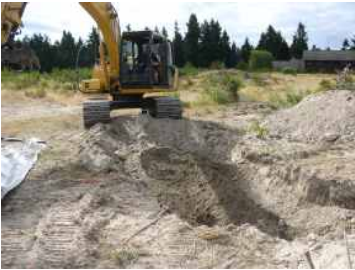
Photograph 01: Excavation area - View east
