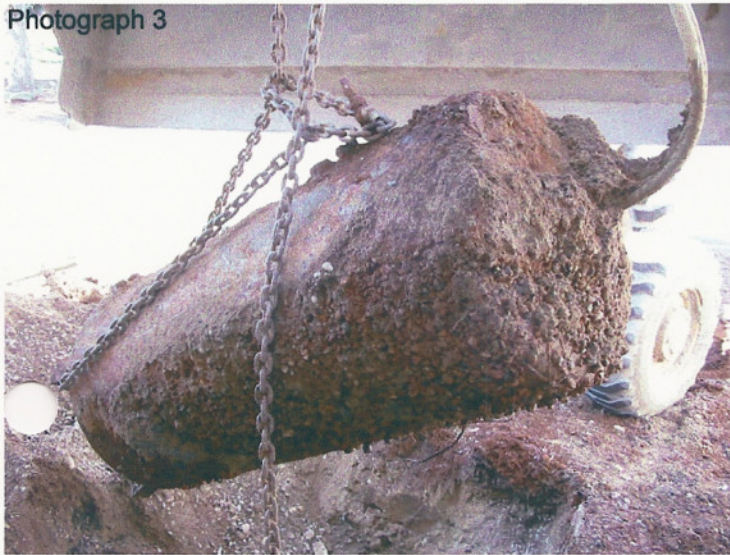
UST 1 during removal
