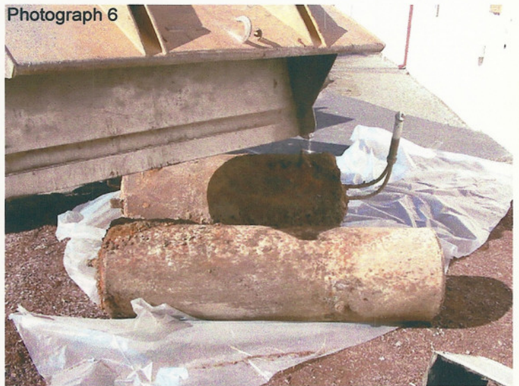
USTs 1 & 2 following removal from excavation
