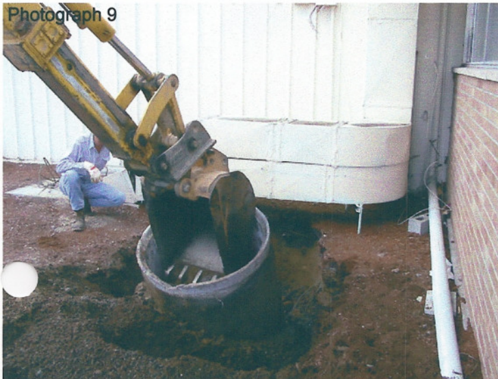
Removal of piping system housing
