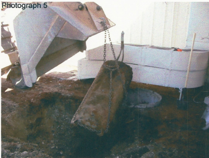
UST 2 during removal
