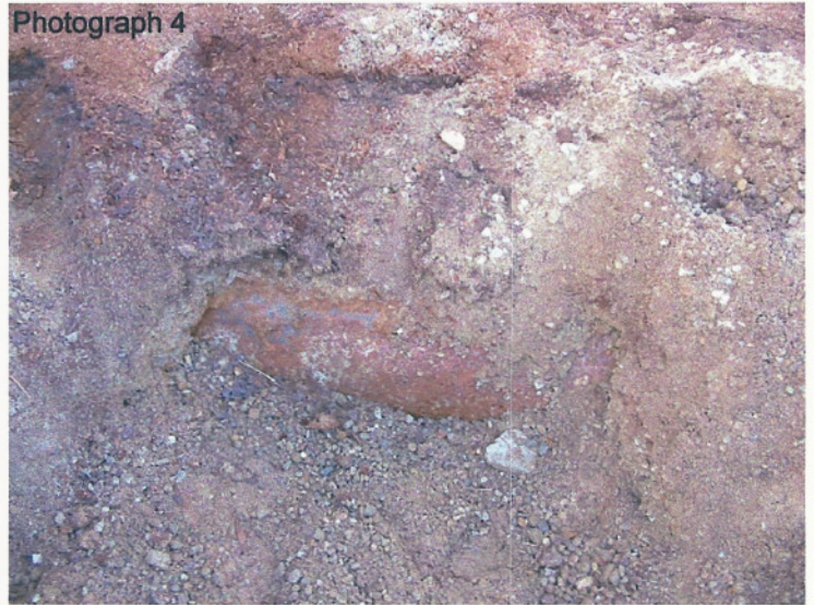
UST 2 observed during soil sampling activities - View to south
