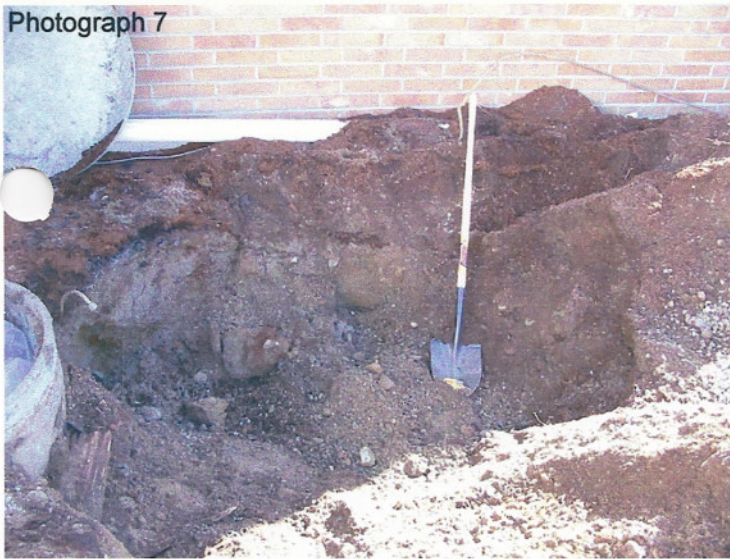
UST Excavation - View to south
