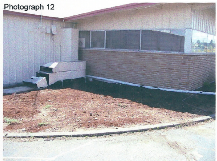
UST excavation area following site restoration
