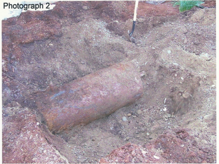
UST 1 during excavation - View to southwest
