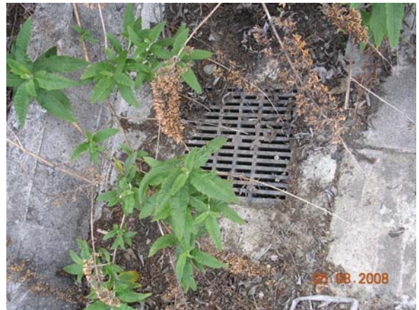
Photo #10 The catch basin in the drum storage area
