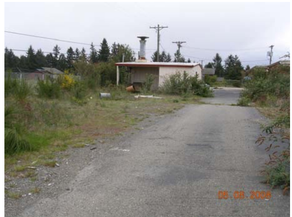
Photo #4 A paved drive east of the main building with the painting building in the background
