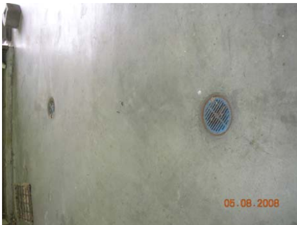
Photo #5 Floor drains in the painting building
