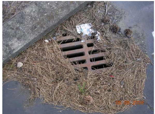
Photo #2 A catch basin in the parking lot
