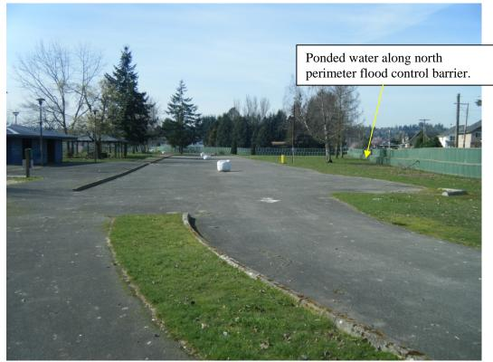
Photo 4- Ponded water observed along north perimeter flood control barrier.
