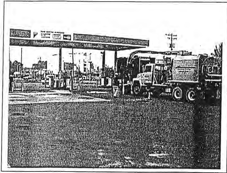
Overview of site, note vacuum truck.
