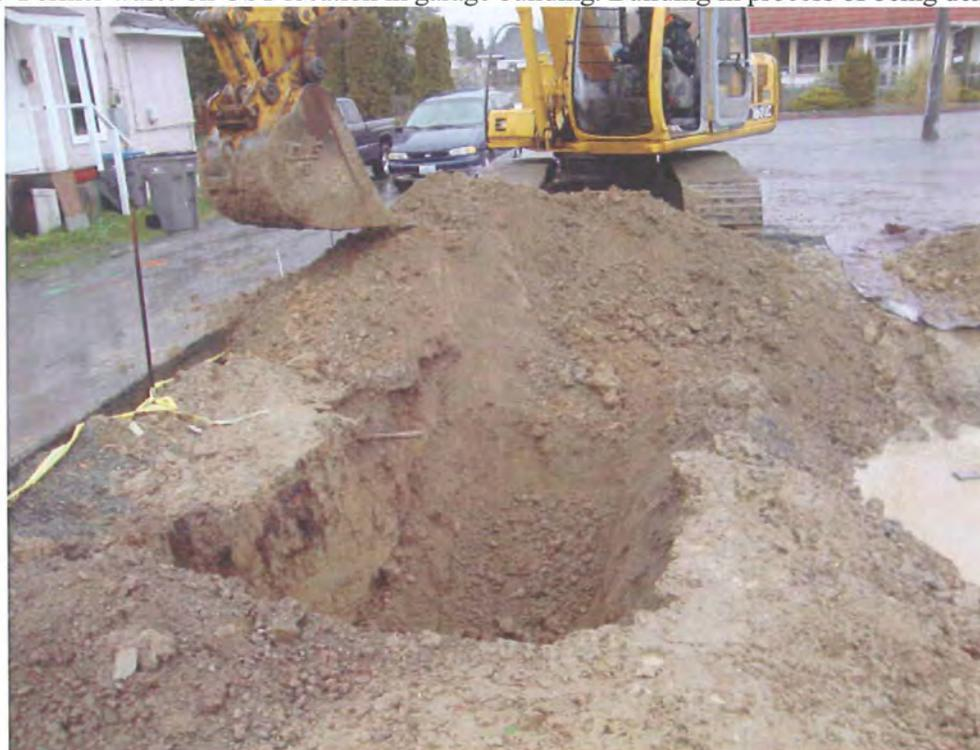
Photo 2: Excavation in former waste oil location.
