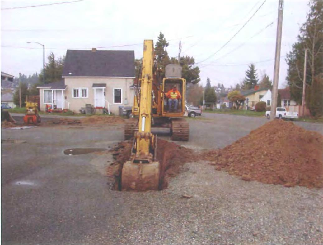
Photo 5. Excavation in the area of the former USTs.
