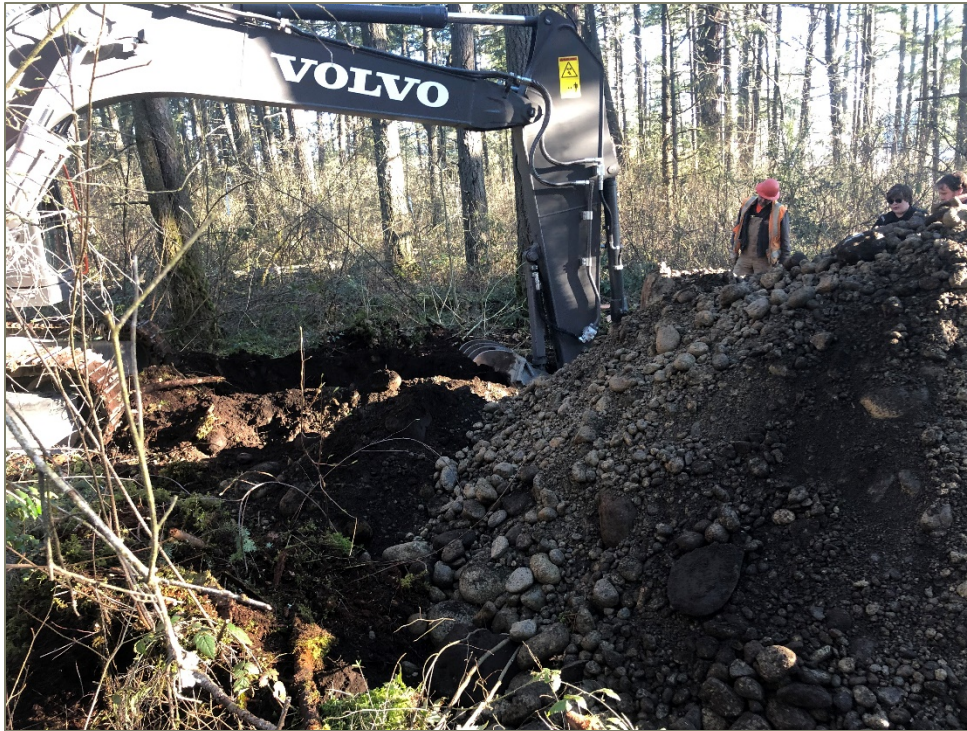
Photograph 1: Excavation of Test Pit 7 (TP-7).
