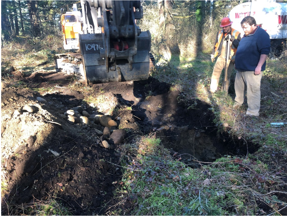
Photograph 3: Excavation of Infiltration Trench 1 (INF-1).
