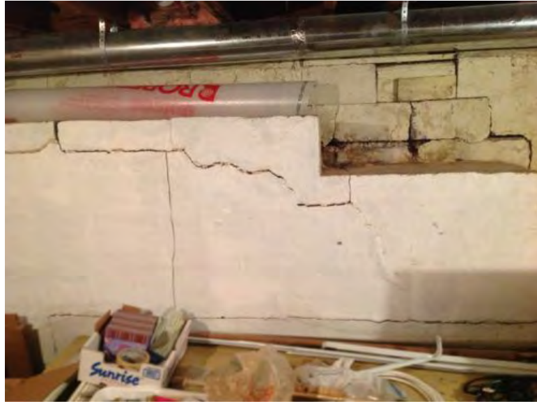
Photograph 21. Foundational cracks in the walls of the basement at 305 N 1st Avenue, July 2013.
