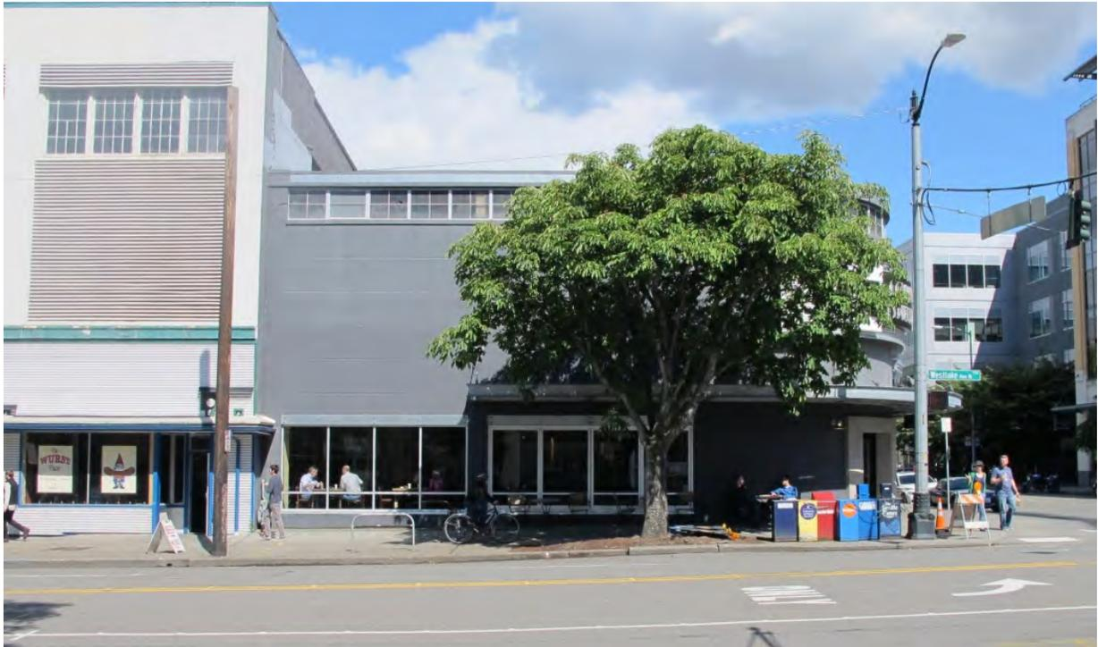
2014 view of west elevation (Westlake Avenue) of south portion of building, originally constructed as an addition in 1947. Windows at roof line retain original 1947 sash; storefront window sash is modern and dates to 2003; corner entry at right is not original and dates to some time between 1968 and 2003.
