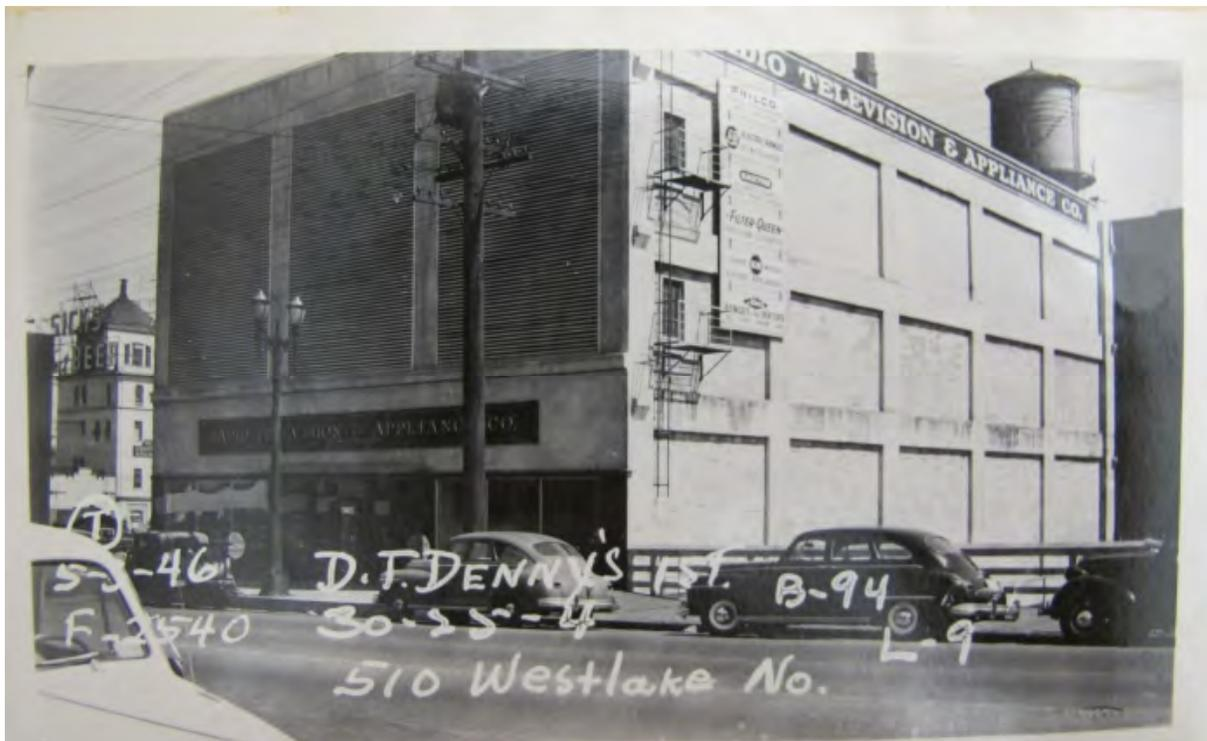
1946 view of the west elevation of building occupying lot 9, with alterations compared to the 1937 photograph. The empty lot to the right is lot 8. Note changes to shaped parapet, upper floor windows, and storefront windows.
