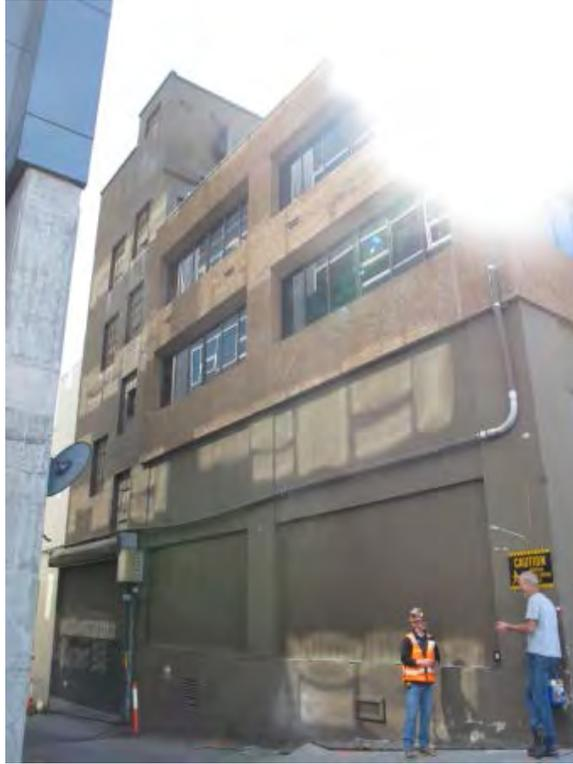
2014 view of east elevation/rear of building (alley). Original 1920 staircase can be seen on the left with steel sash windows which have been painted over.
