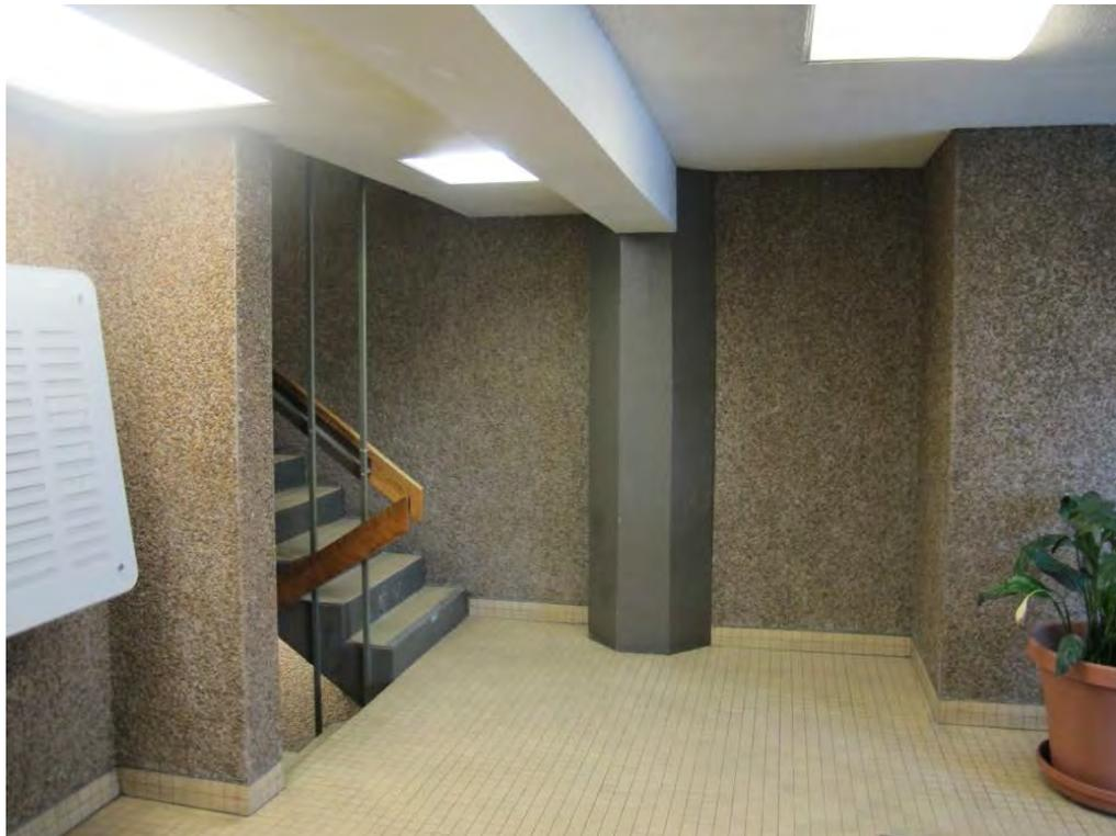
Interior-first level, lobby space, showing marbled concrete walls, tile flooring, wooden railing on staircase, low suspended ceilings of acoustic tile.
