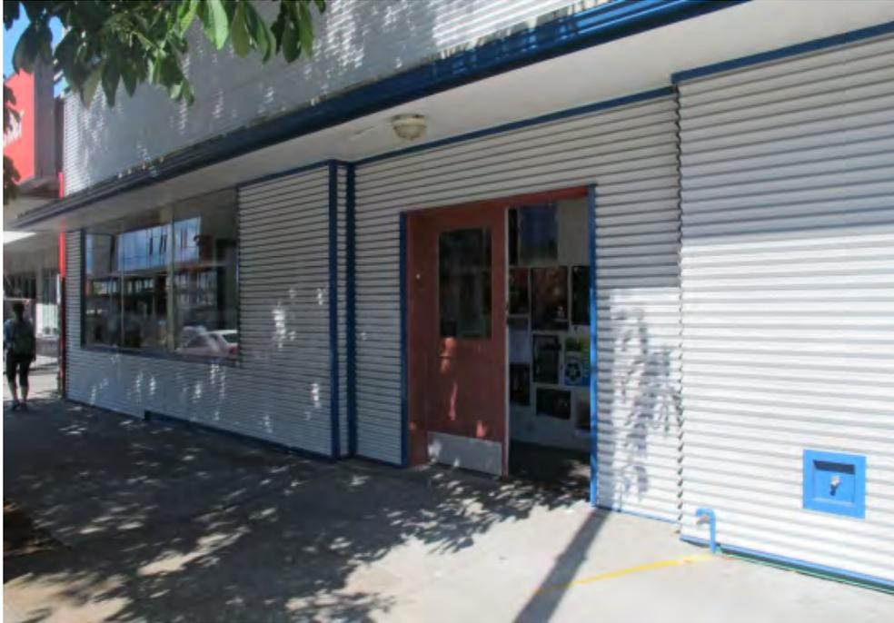
2014 storefront view of north portion of building (510 Westlake) originally constructed in 1919, showing entrance to The Wurst Place, a restaurant. Non-original corrugated metal siding at first floor was installed at an unknown date. First floor windows may date from 1947 renovation to building. Entry door is recent and not original.
