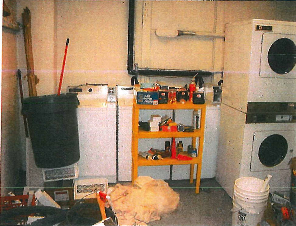
Photograph 2 Del Roy Apartments
