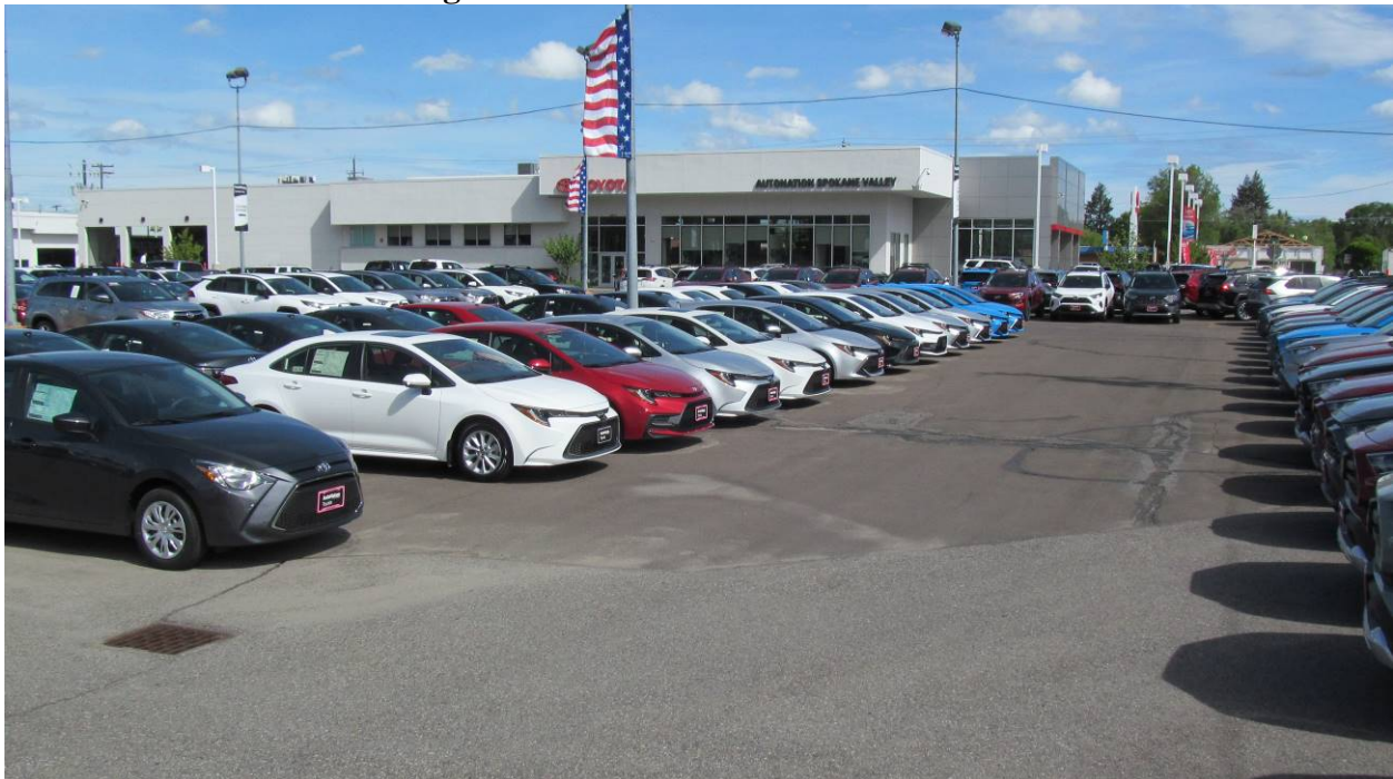
Photo 2: East Side of Building - from the northeast
