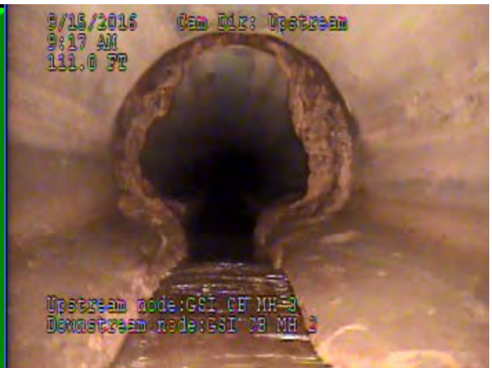
Photo E-10: Sedimentation in and evidence of leakage along joints (right) in the stormwater conveyance system.
