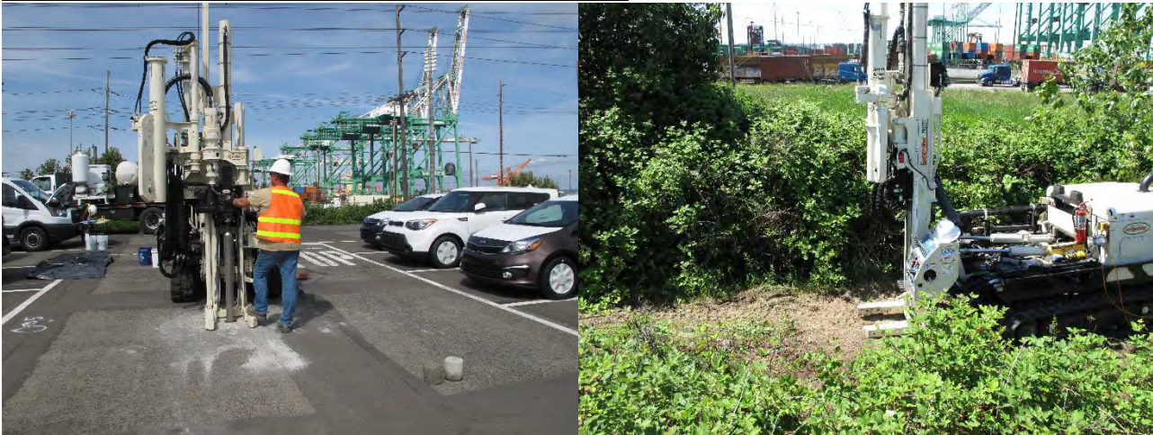
Photo E-12: Geoprobe Drill Rig
