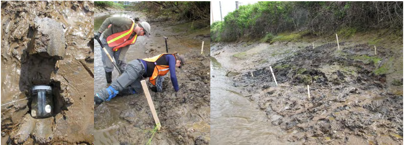
Photo E-19: NMDS Installation
