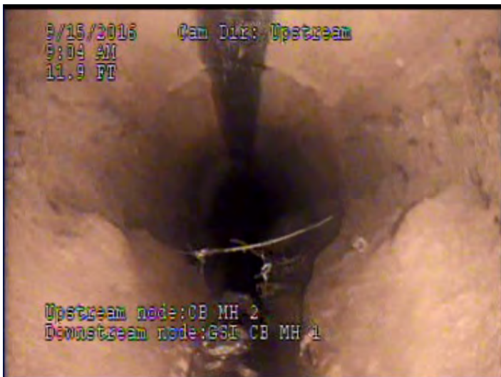
Photo E-10: Sedimentation in and evidence of leakage along joints (right) in the stormwater conveyance system.
