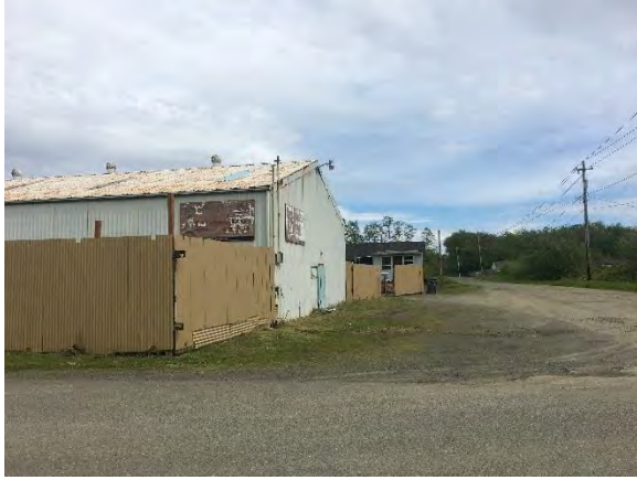
Exterior view of adjacent building associated with large AST - facing east
