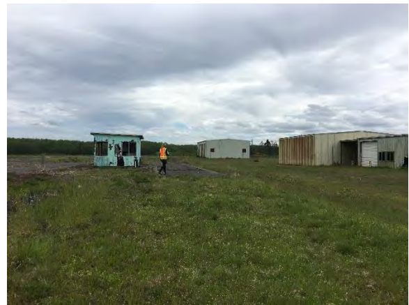
View of abandoned buildings in northwest portion of property - facing east
