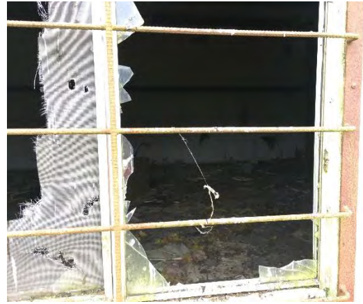
Interior view of eastern most abandoned building - facing south
