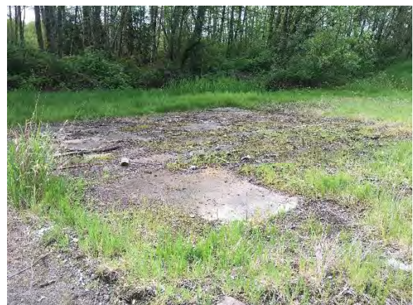
Building footprint in northeast corner of property - facing south
