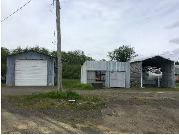
View of three storage structures - facing west
