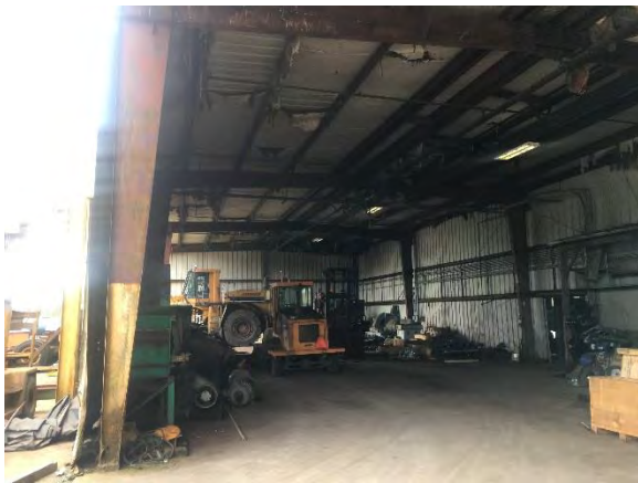
Equipment inside Willis Enterprises warehouse – facing south
