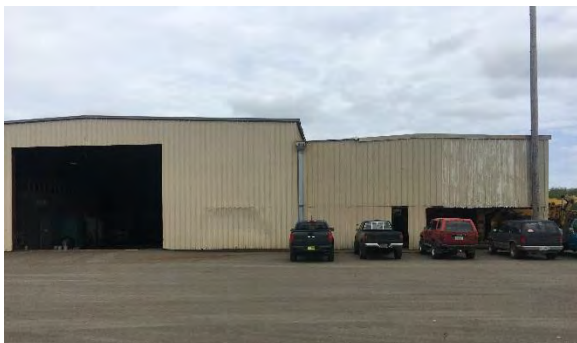
View of Willis Enterprises warehouse – facing north
