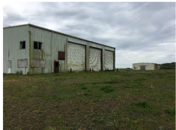
Exterior view of eastern most abandoned building - facing southwest
