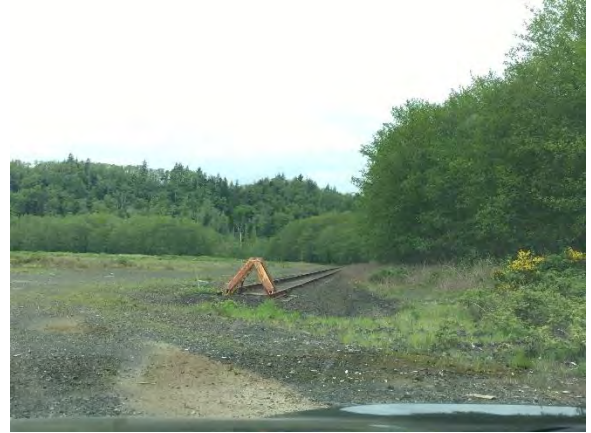
Rail spur - facing north
