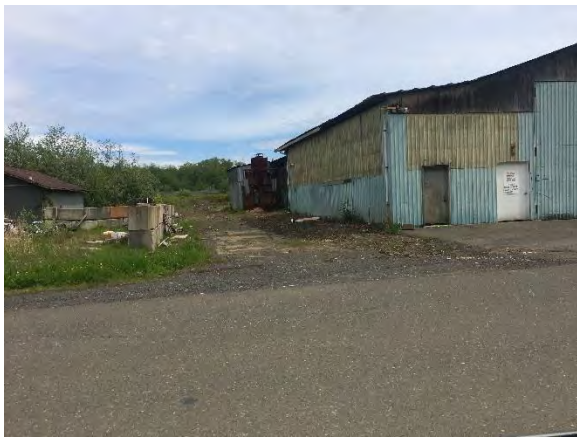
View of adjacent property - facing east
