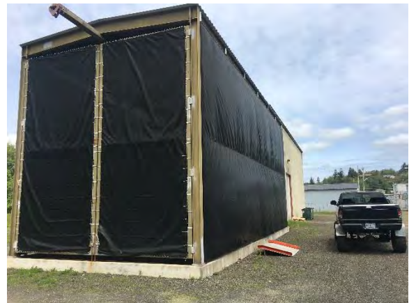
Eastern side of warehouse - facing north
