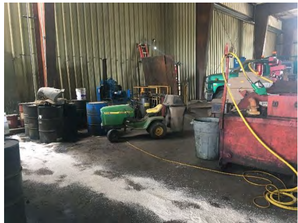
Absorbent material noted around 55-gallon drums and diesel AST
