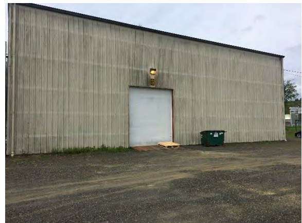
Eastern side of warehouse - facing west
