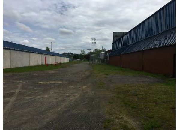
Pole-mounted transformers - facing east
