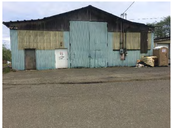
View of adjacent property - facing east
