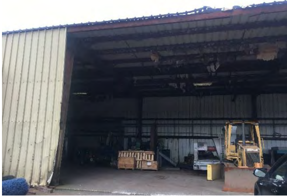
Willis Enterprises warehouse – facing west
