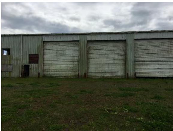
Exterior view of eastern most abandoned building - facing south
