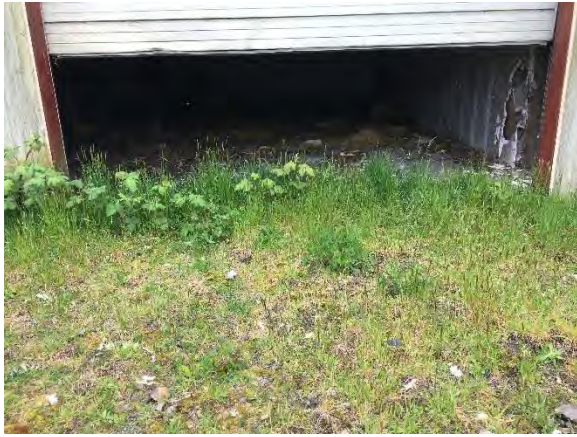
Interior view of western most abandoned building - facing south
