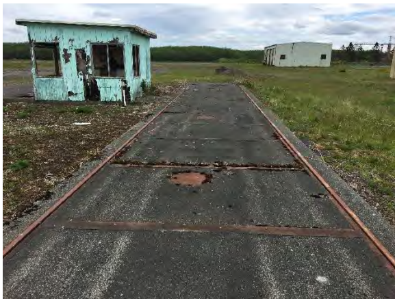
South side of weigh station - facing east
