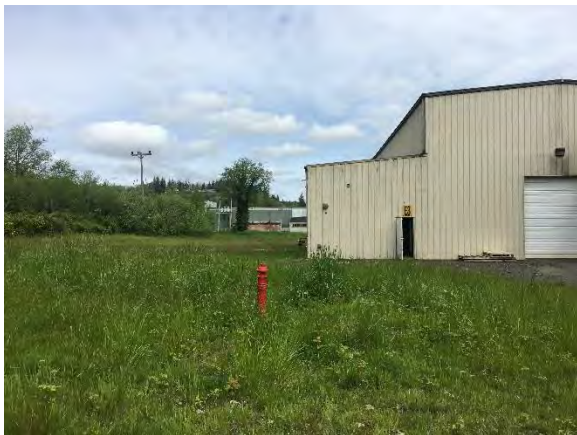
View of warehouse in northeast corner of property - facing north
