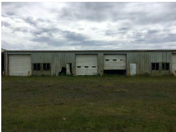
Exterior view of westernmost abandoned building - facing south
