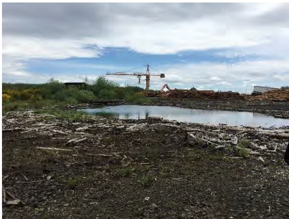
Standing water west/northwest of Willis Enterprises
