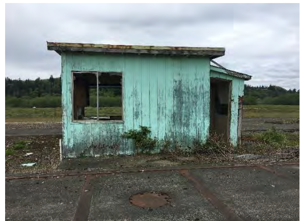
Exterior view of weigh station office - facing north
