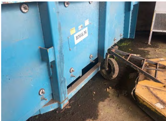
Oil staining inside Willis Enterprises warehouse
