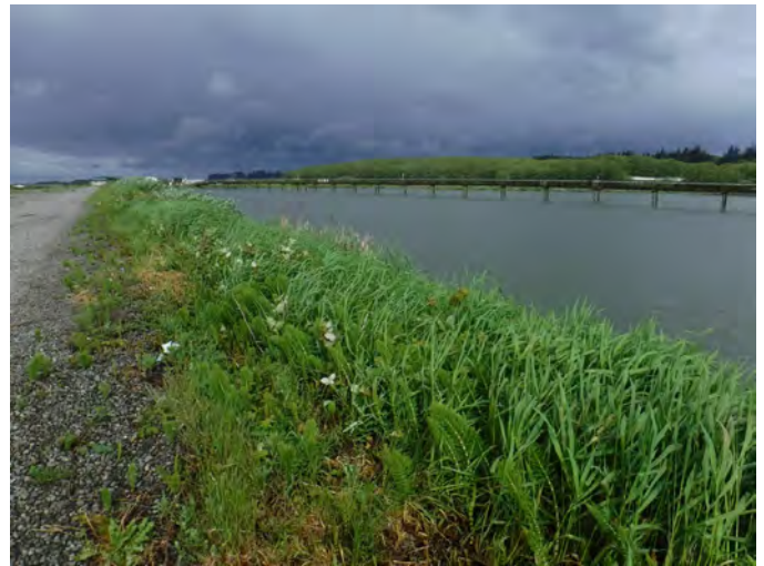
City of Hoquiam Wastewater Treatment Lagoon (non-wetland)
