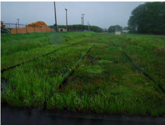
Stormwater Bioswale (non-wetland) facing East
