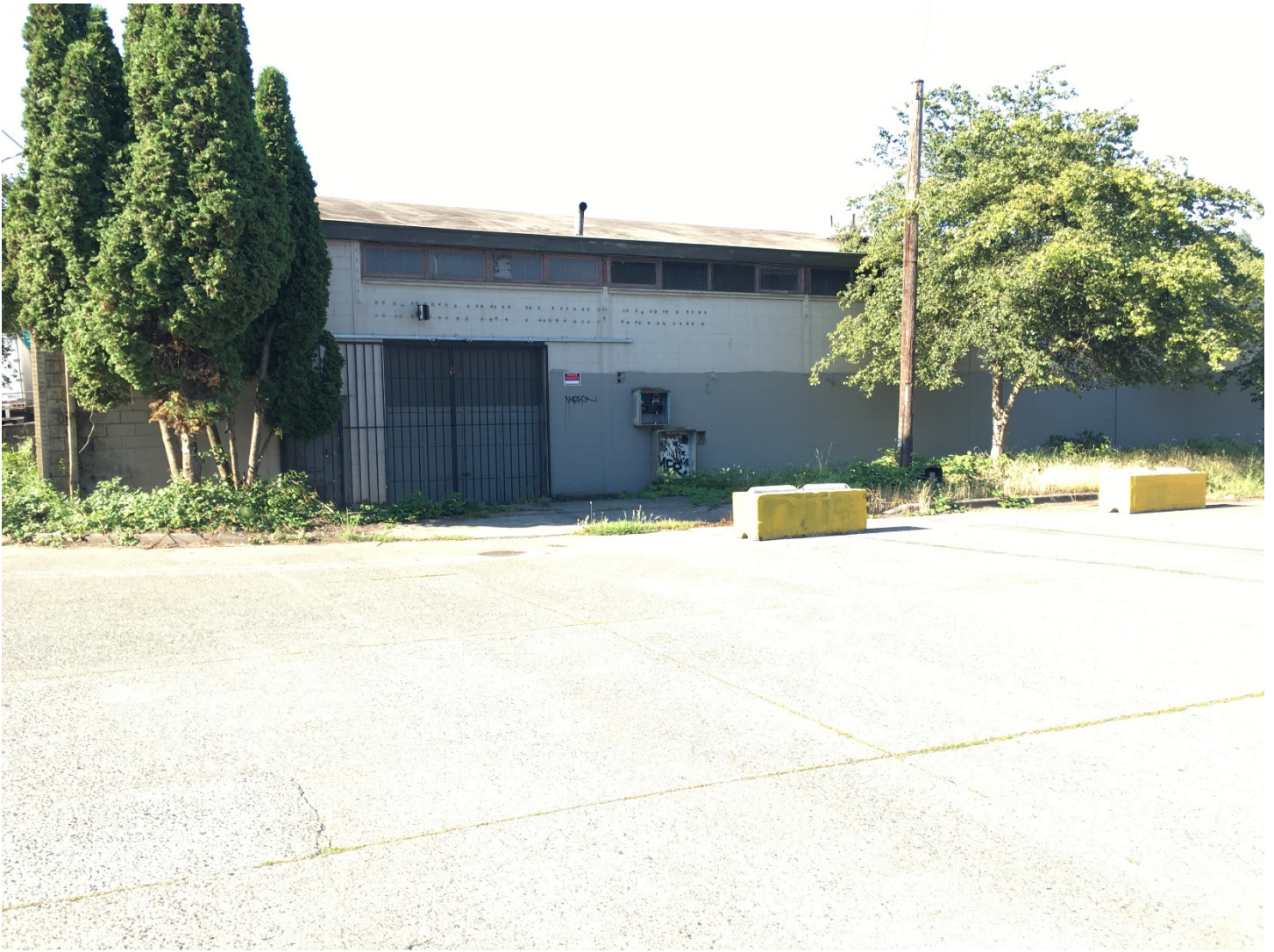
Figure 7. Photo taken during 7/29/19 site visit. East end of the north side of the former Northwest Plating building.
