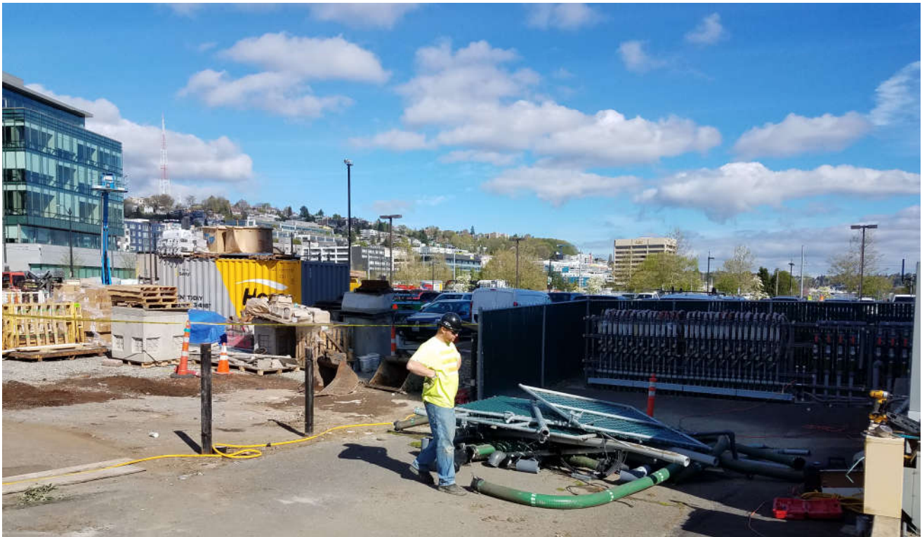
Photograph 4: View to the north – Removal of system fencing and conveyance piping.
