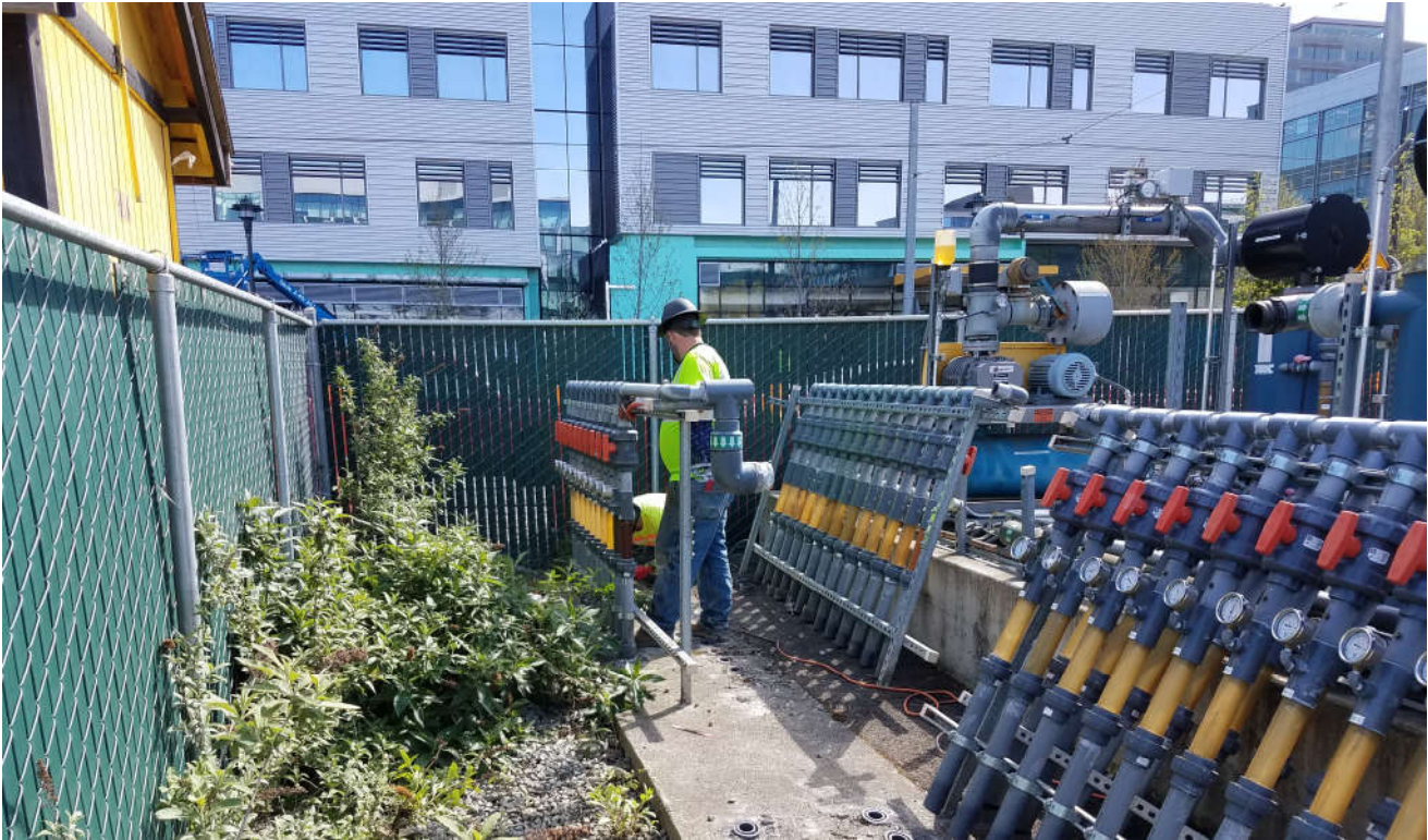
Photograph 5: View to the east – Removal of SVE manifolds.
