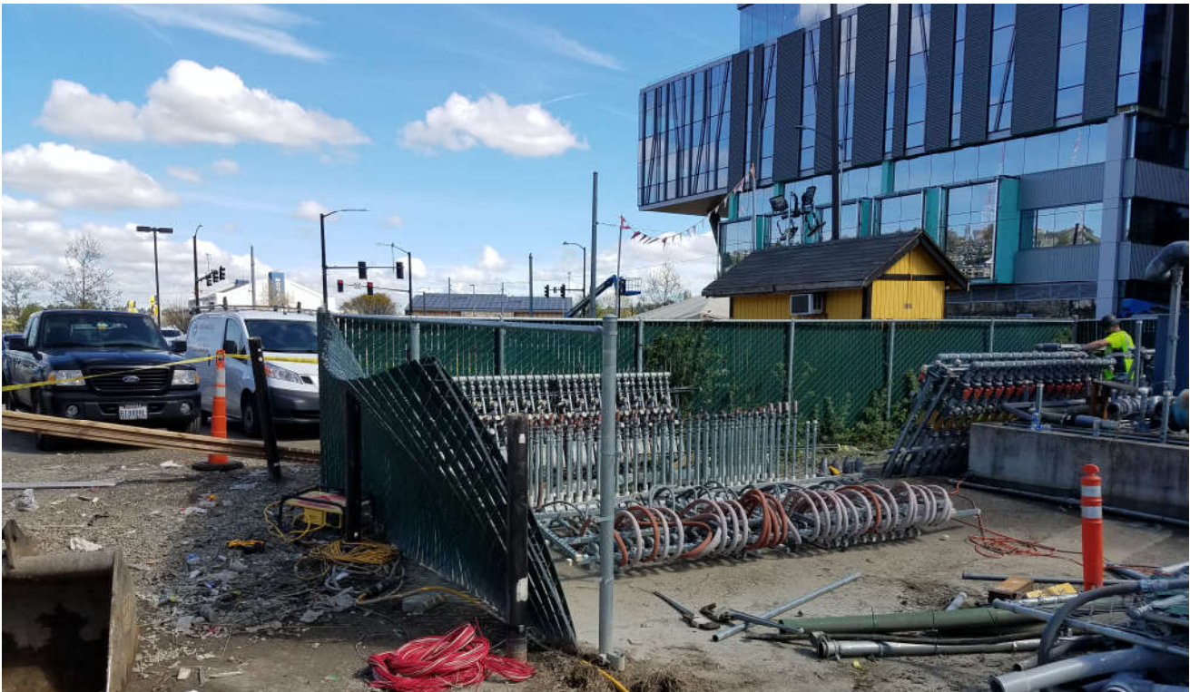
Photograph 6: View to the northeast – Removal of air sparge manifolds.
