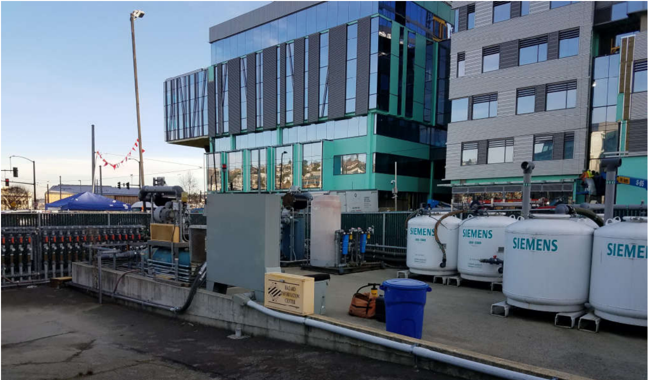
Photograph 1: View to the northeast – Former remediation system compound prior to removal.
