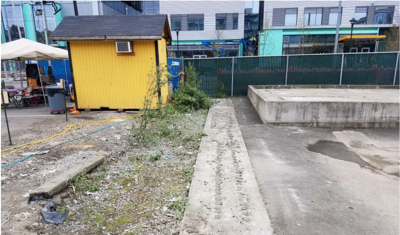
Photograph 13: View to the east – Grout sealed manifold piping.
