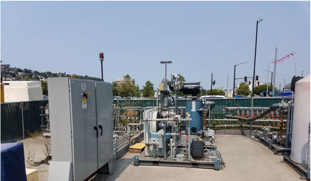
Photograph 2: View to the north – Former remediation system compound prior to removal.
