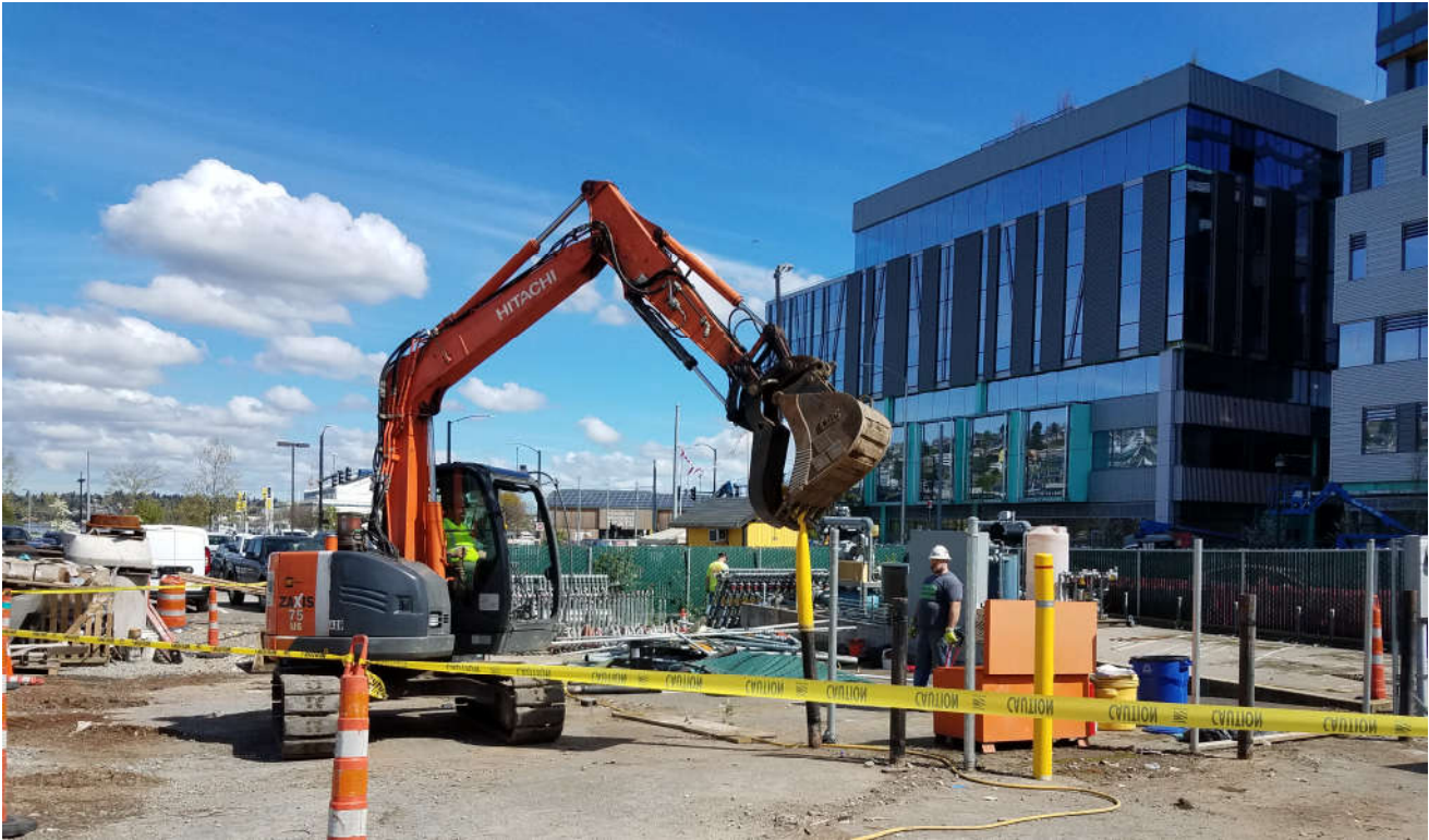
Photograph 7: View to the northeast – Removal of bollard posts.
