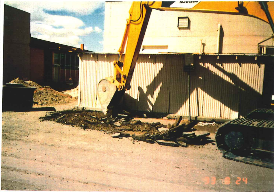
PHOTOGRAPHED BY: Paul Danielson DATE: 8/24/93 VIEW: Excavation in progress at Tank #24 location. Tank located beneath galvanized shed in background at 1342 Jadwin Avenue. Note vent pipe on masonry wall behind street sign. Tank left in place.
