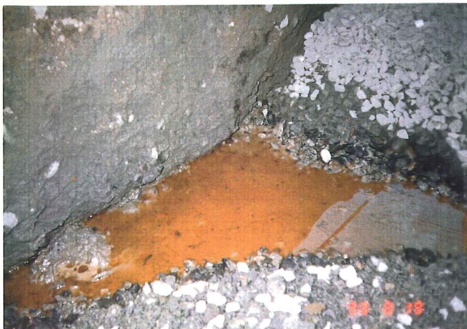
PHOTOGRAPHED BY: Dan Uldall DATE: 8/19/93 VIEW: Floating product on groundwater on south side of tank #10-#16 excavation. Gravelly backfill visible at top and bottom of photo - discolored PCS visible at left under footing.
