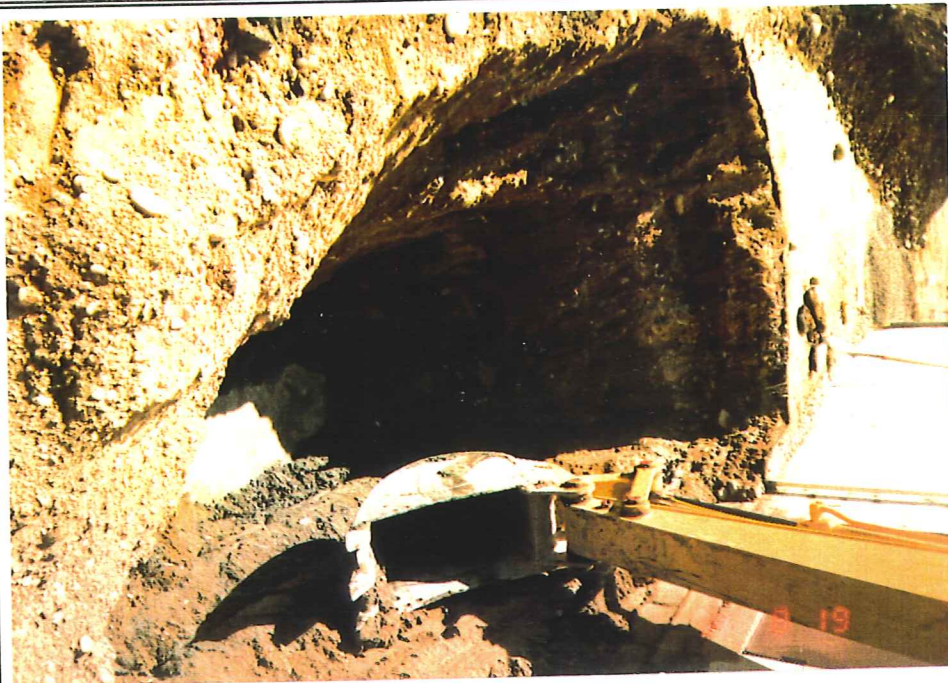
PHOTOGRAPHED BY: Dan Uldall DATE: 8/19/93 VIEW: Excavation adjacent to Tanks #19 and #20 (under building at 1364 Jadwin Avenue). Groundwater visible in base. The tanks were not removed.
