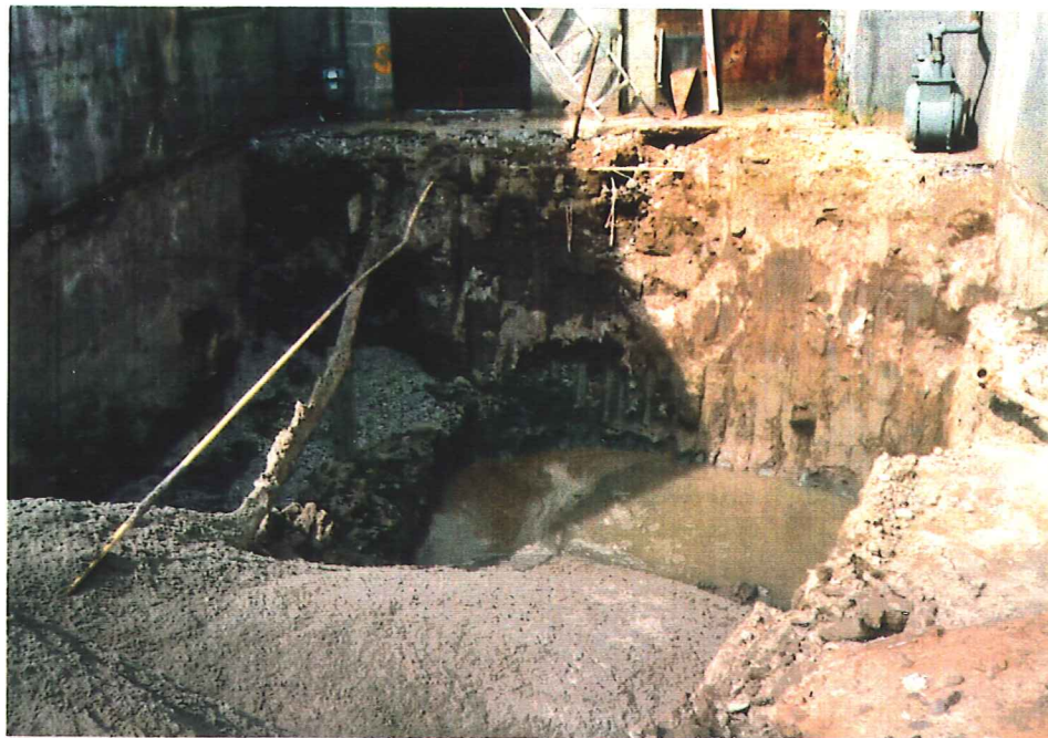
PHOTOGRAPHED BY: Dan Uldall DATE: 8/20/93 VIEW: Partially backfilled excavation from which Tanks #10-#16 have been removed. Groundwater visible with floating product to the left. Gasoline and sewer lateral crossing excavation on left half of photo. Greenish gray PCS visible near water. Excavation is in alcove bounded by 1386, 1388 and 1398 Jadwin Avenue.
