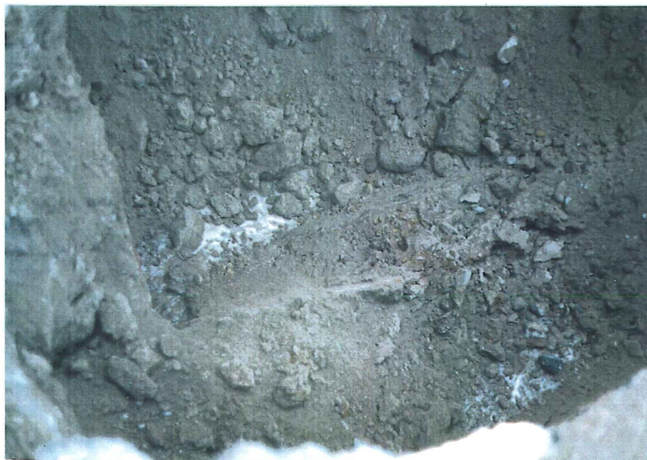
DATE: 8/09/93 VIEW: Tank #3 excavation behind 1319 George Washington Way. Some PCS visible. Water from broken sewer lateral leaking in at left (north).
