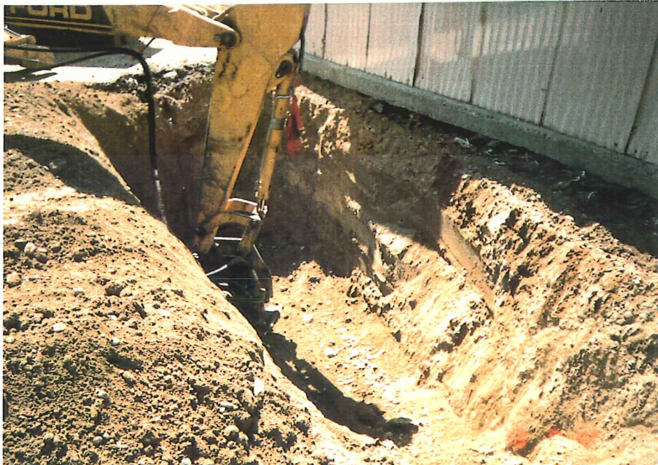
PHOTOGRAPHED BY: Paul Danielson DATE: 8/24/93 VIEW: Backfilling and compaction of Tank #24 excavation. No free product or PCS soils were observed.
