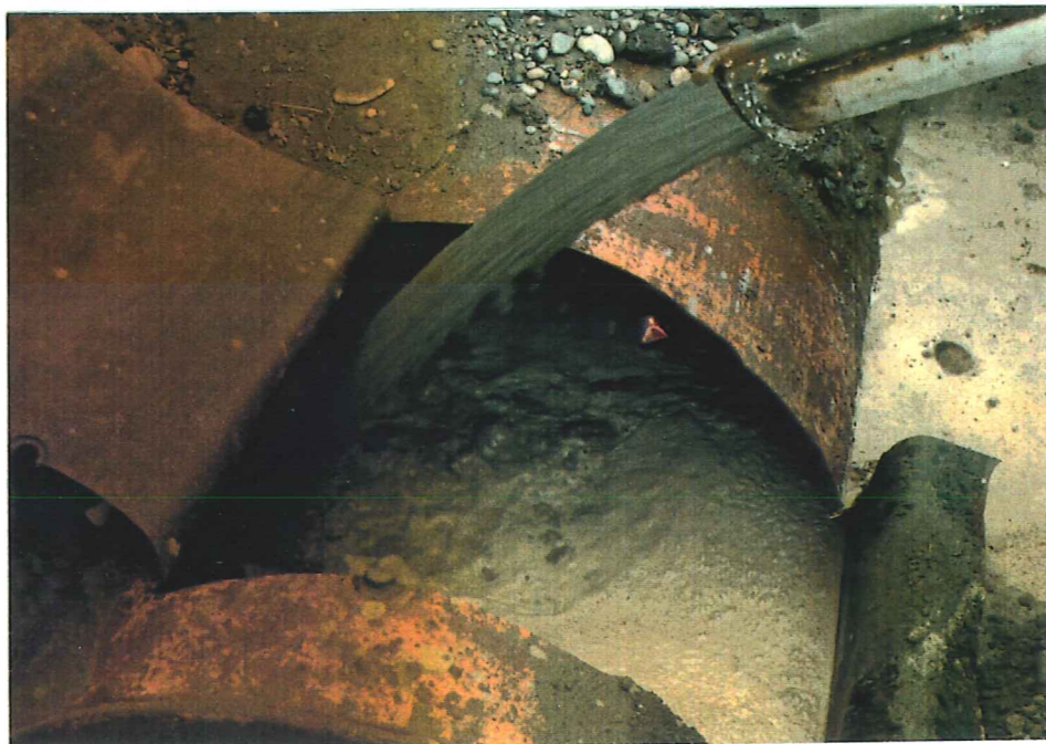
PHOTOGRAPHED BY: Dan Uldall DATE: 8/19/93 VIEW: Grouting of Tank #7 during abandonment in place procedures.
