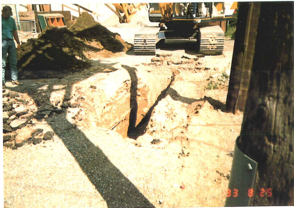
PHOTOGRAPHED BY: Dan Uldall DATE: 8/25/93 VIEW: Trench adjacent to Tank #32 behind 1375 George Washington Way to evaluate potential PCE groundwater contamination.
