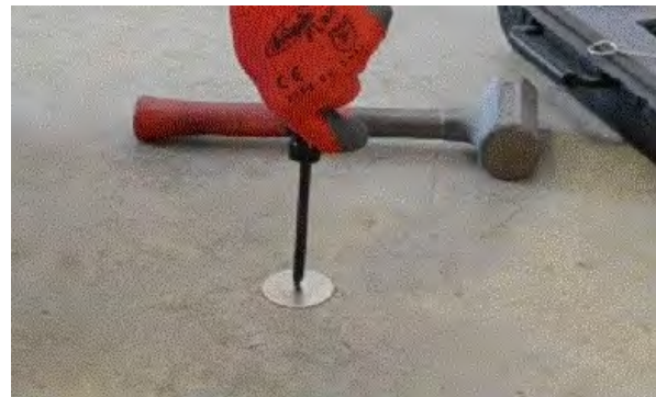
Figure 5. Tightening the Secured Cover.
