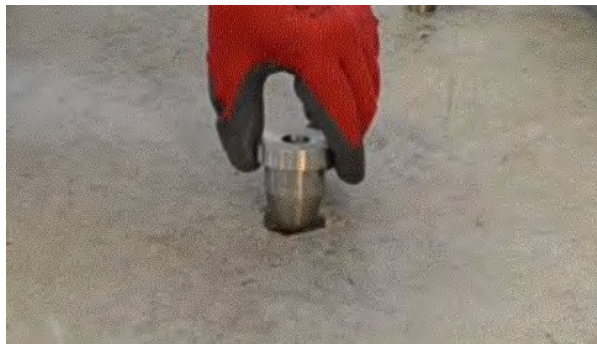
Figure 3. Testing Depth with the Drilling Guide.
