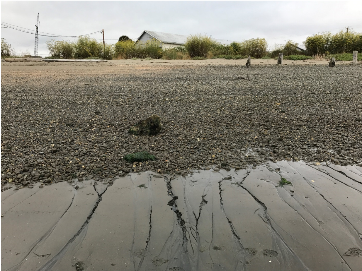
View from the lower beach looking east at the Quiet Cove Site (building is the office/maintenance building).
