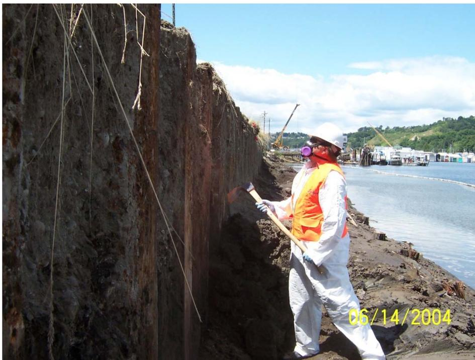
**Photo P-3b:** During shoreline remediation approximately the upper 6' of the sheet pile wall on the waterway side was exposed.
