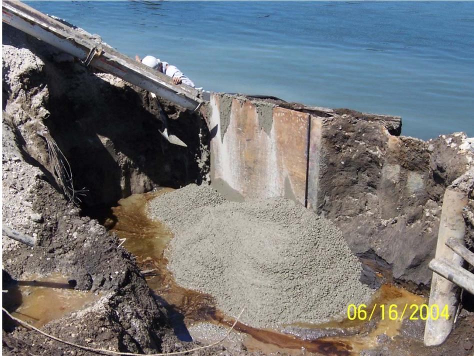
**Photo P-8a:** Hole repaired by Arkema by welding a plate onto the existing sheet pile wall and backfilling excavation with concrete.
