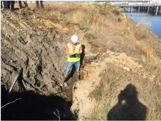
Each test pit was backfilled with soil excavated from the test pit. The backfill material was placed in appropriate lifts and compacted with the excavator bucket and track-rolled.
