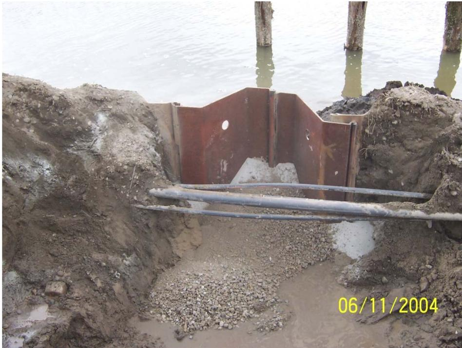
**Photo P-6a:** Hole in sheet pile wall was repaired by Arkema by welding a remnant pair of sheets to the existing wall and placing grout along the weld seam.
