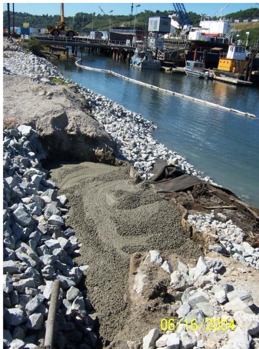
**Photo P-8b:** Groundwater and soil outside of the repair was removed and backfilled with spalls. Soil was placed over the concrete once it cured.
