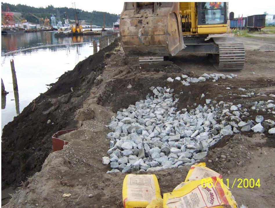
**Photo P-6b:** Hole around repair was backfilled.
