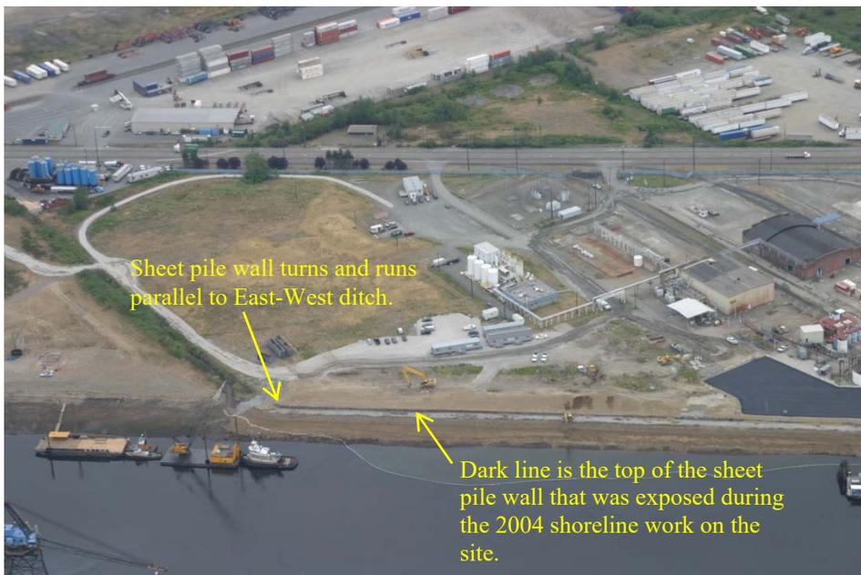
**Photo P-1b (07-02-2004):** The top of the sheet pile wall was exposed during the 2004 shoreline remediation work. As the wall nears the East-West Ditch, it turns parallel to the ditch and continues for approximately 300' along the ditch.
