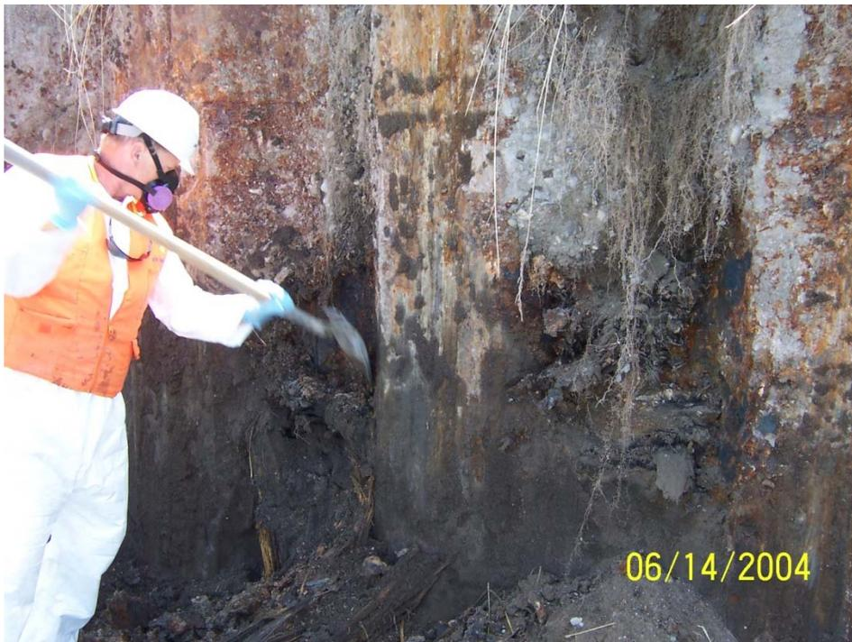
**Photo P-4b:** Worker clearing around a timber pile at sheet pile wall.
