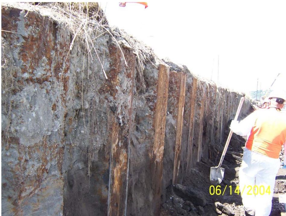
**Photo P-2b:** Workers removing soil from inshore sheet pairs to identify sheets that were driven low. Two pair driven 4'-5' low were discovered and repaired by Arkema.
