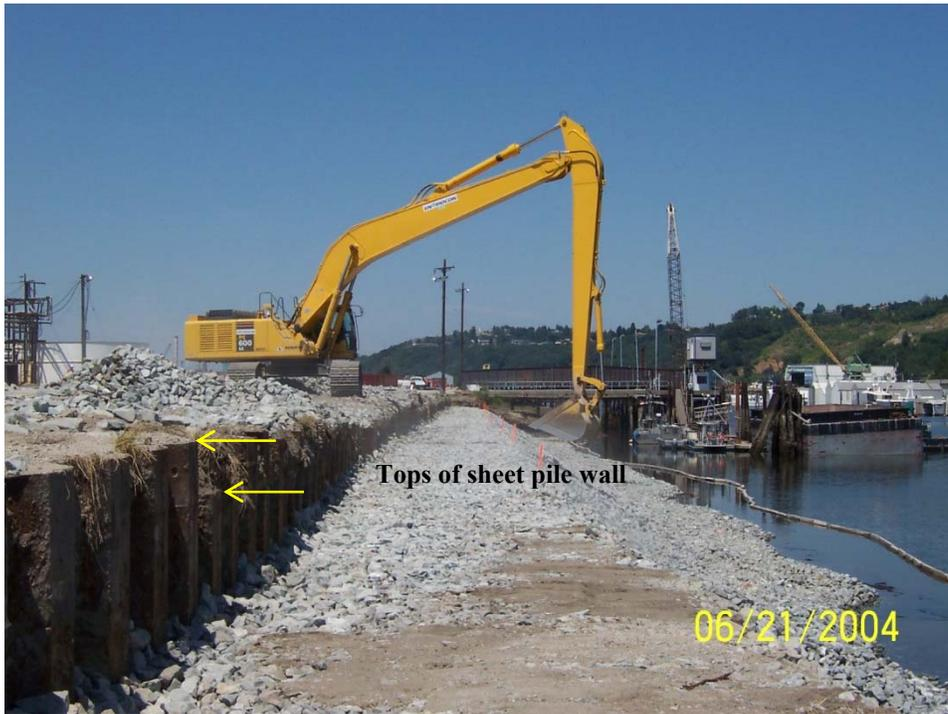
**Photo P-2a:** Top of sheet pile wall varied in elevation by several feet.
