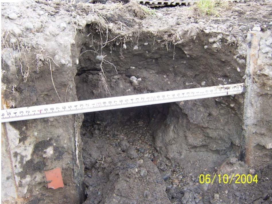
**Photo P-5a:** First hole at top of sheet pile wall resulting from sheet pair being driven too low.
