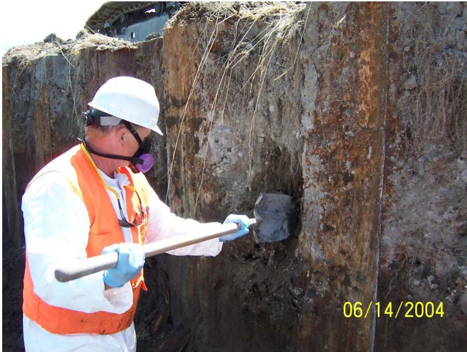
**Photo P-4a:** Worker removing soil from inshore pair of sheet pile.
