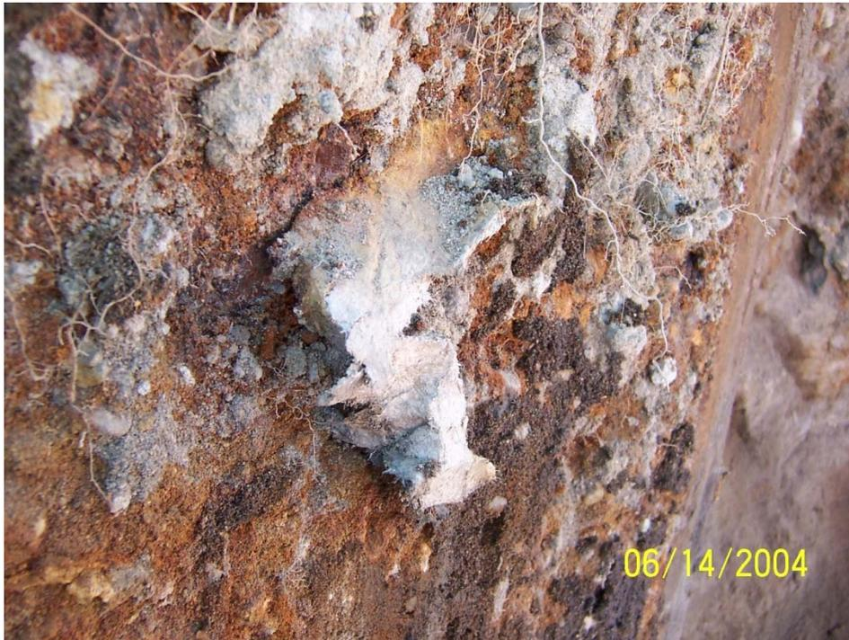
**Photo P-3a:** Close-up of white substance observed on sheets along the length of the wall. Substance was similar to a white precipitate observed along the shoreline prior to remediation
