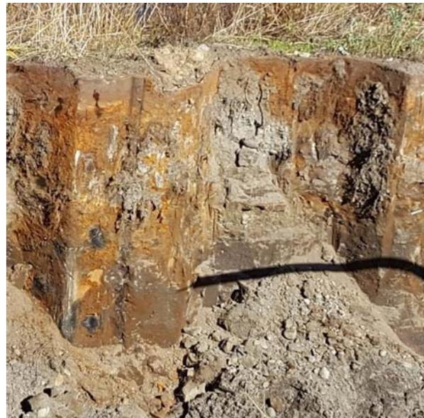
Figure 1: Typical condition of exposed sheet piling
