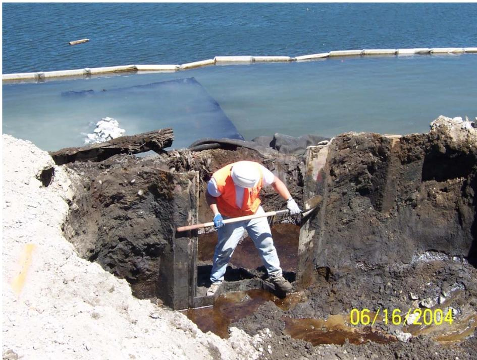
**Photo P-7b:** Second hole in sheet pile wall was approximately 4.5' wide by 5' high. Brown groundwater visible at bottom of excavation.
